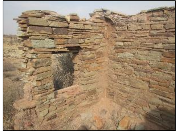
Figure 5-23: Part of a house at waypoint 112 in HLO2 showing stone walling and a remnant of a brakdak.
