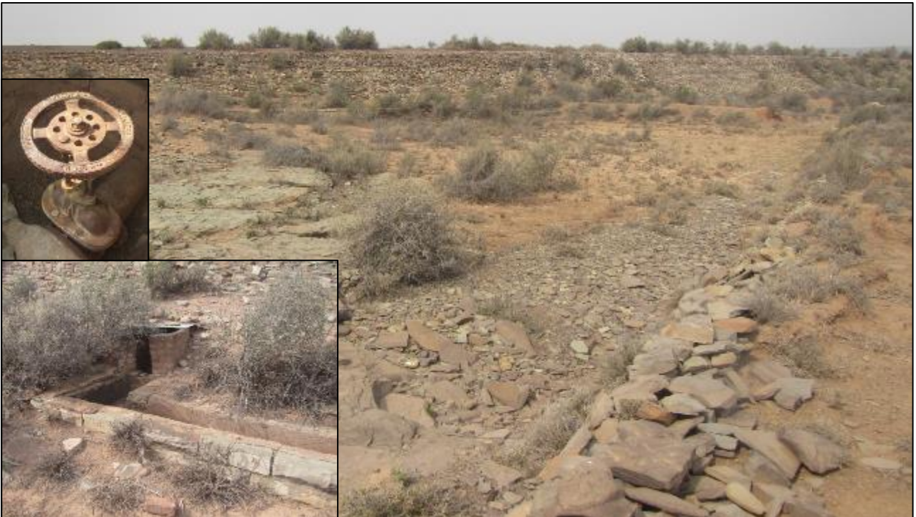
Figure 5-29: View of the large dam at waypoint 100 in HL02 with the insets showing the outlet valve and associated leiwater .
