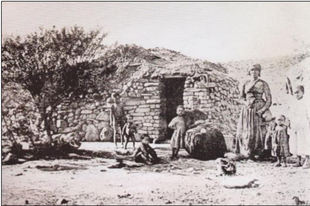
Figure 5-5: A shepherd's hut photographed near Beaufort West in the early 20th century. Note the low, narrow doorway and informal roof structure. Source: Schoeman (2013:48).
