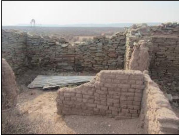
Figure 5-22: Part of a house at waypoint 112 in HLO2 showing sun-dried bricks, stone walls and a filled in doorway.
