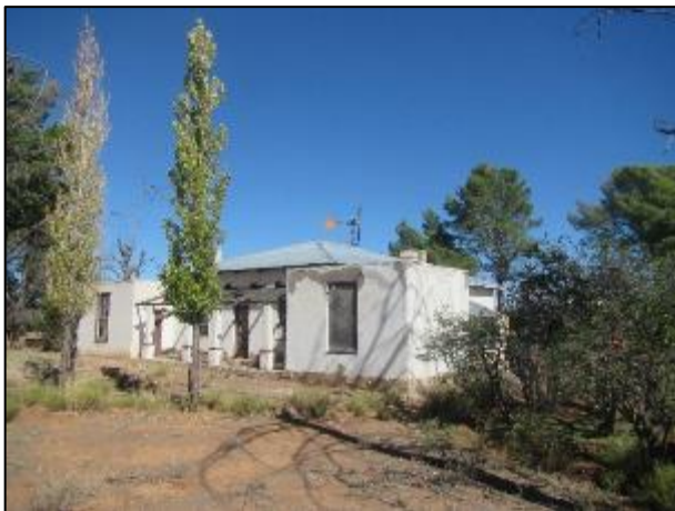
Figure 5-48: The main house at waypoint 1692 in HL01 as seen from the north.
