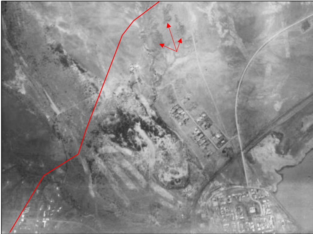
Figure 5-46: Aerial view of northern Beaufort West from 1945 (Job 90, strip 019, photograph 01387) showing the extent of the town. The red line shows the proposed bypass road. The historic quarrying activities can be seen (arrowed).
