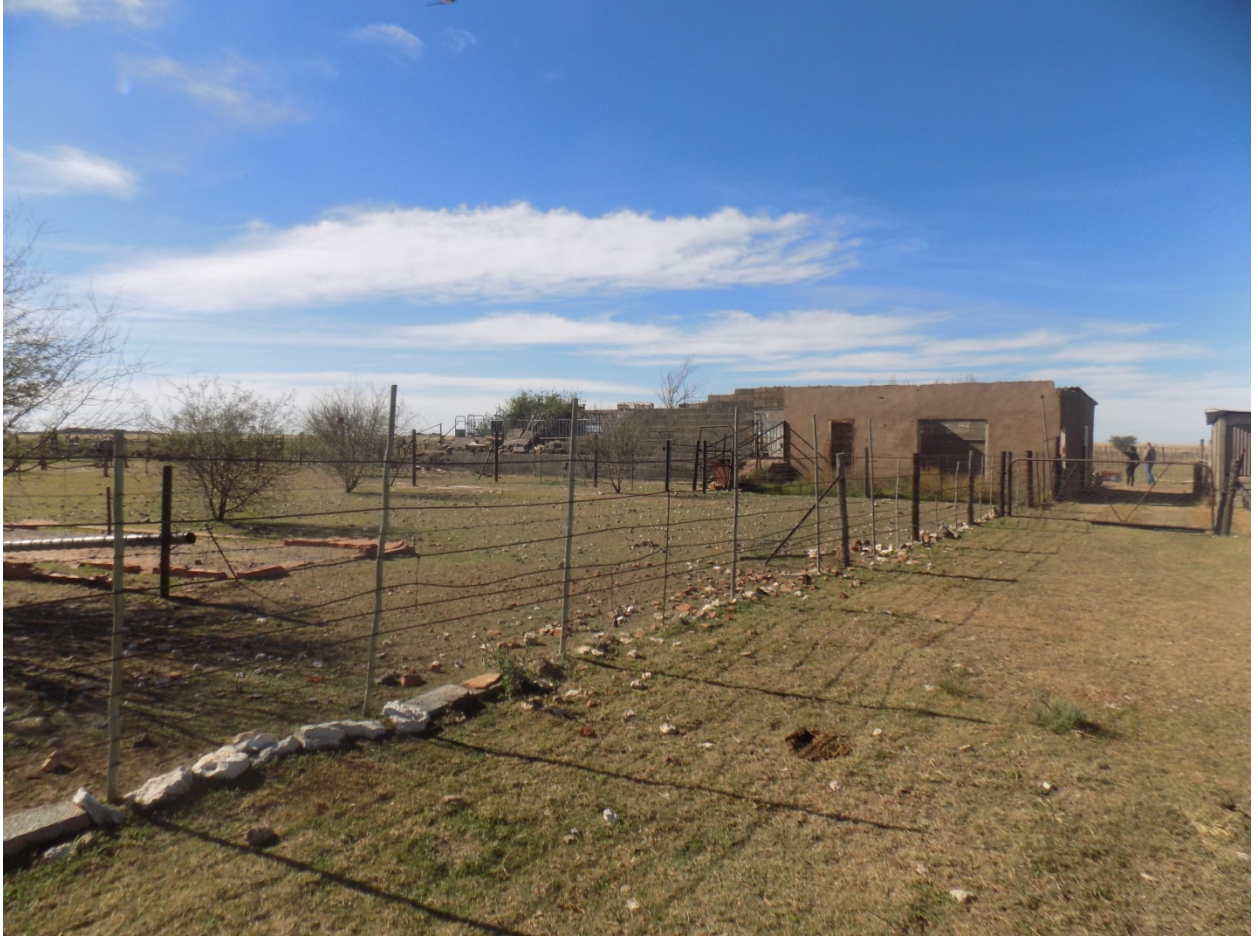
Figure 3. General view of the site, looking west.
