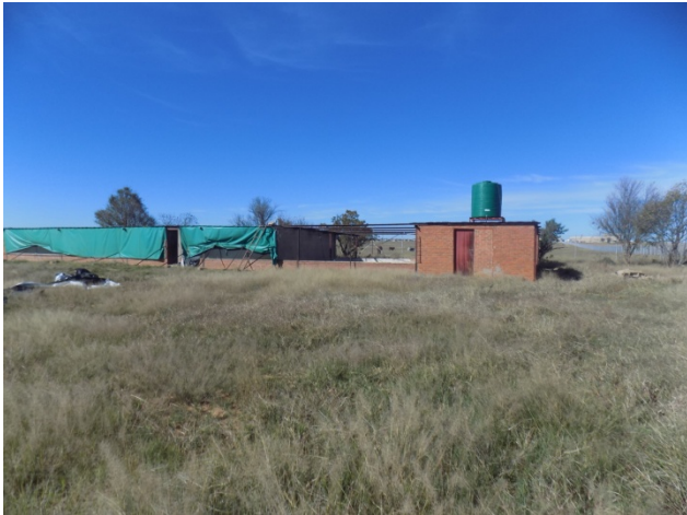
Figure 7. Dilapidated farm workers' dwellings.
