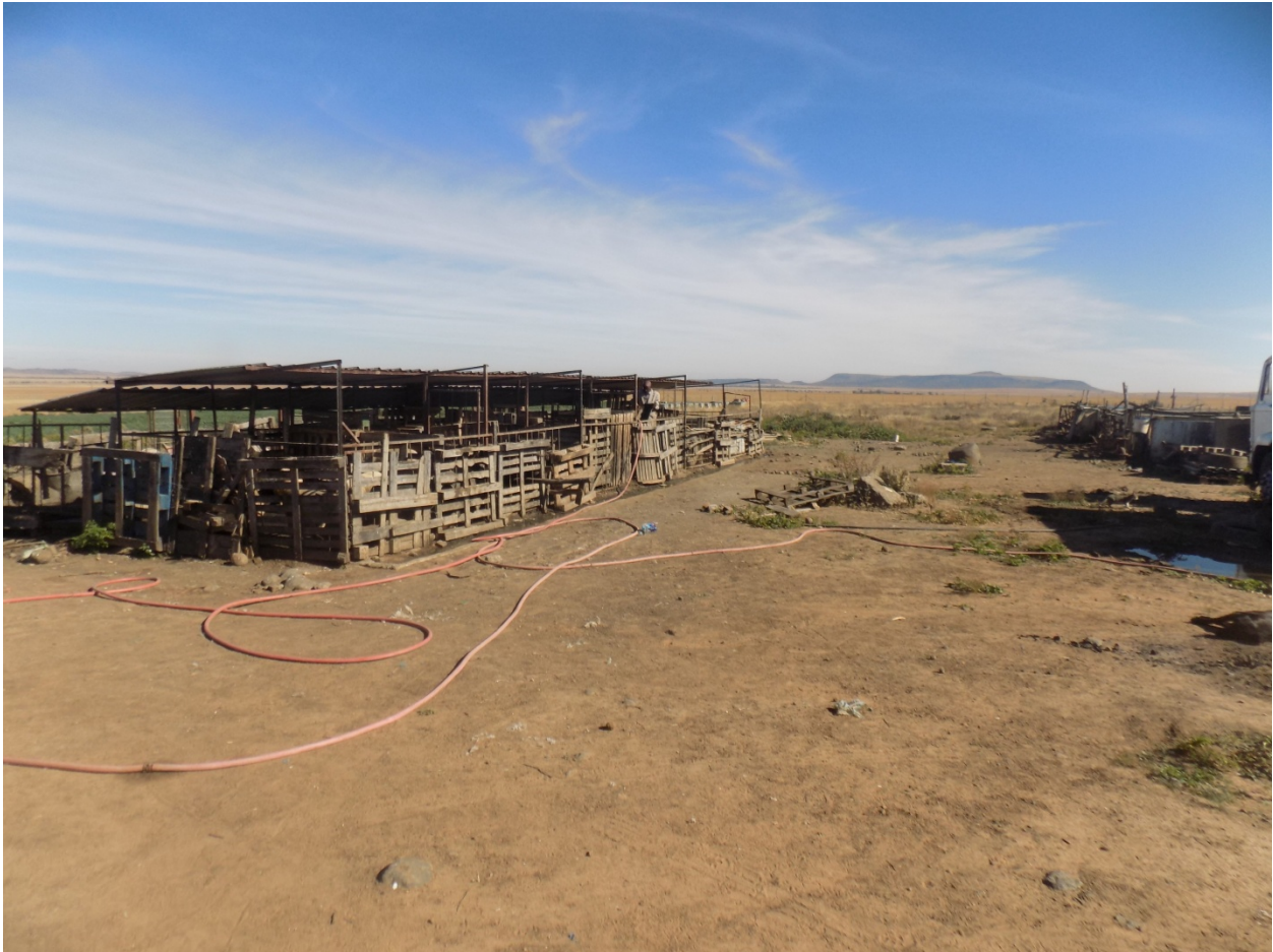
Figure 3. General view of the site, looking north.
