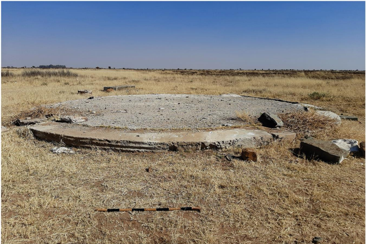
Figure 10. Remains of degraded modern structures identified within the WWTW footprint.
