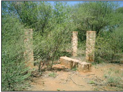
IMAGE 9: VH005 historic structure
