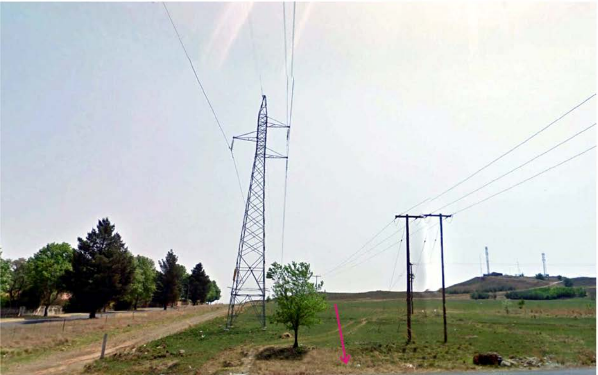
Figure 2. General view of the footprint looking northwest towards the switchyard site (above)
