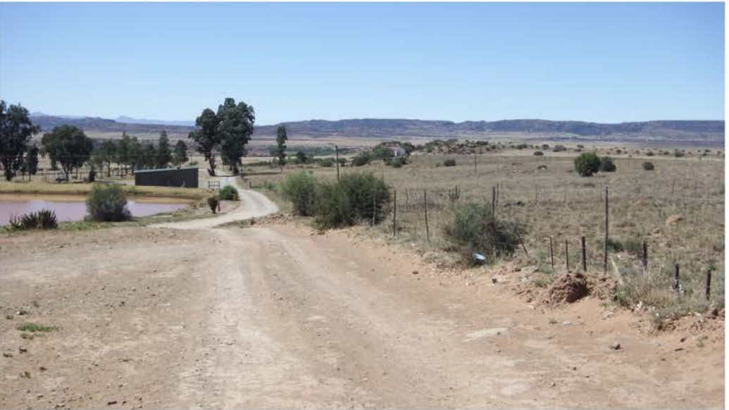
Figure 14. Condition of pipeline sections 1 (top & center) and 2 (bottom).
