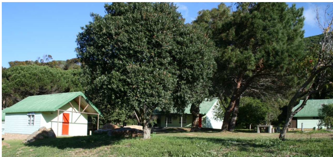
Prefabricated buildings of the Allan Jeffes Camp on the site
