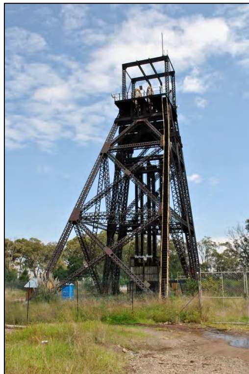
Figure 11-3: Head gear for the Durban Roodepoort Deep Mine
