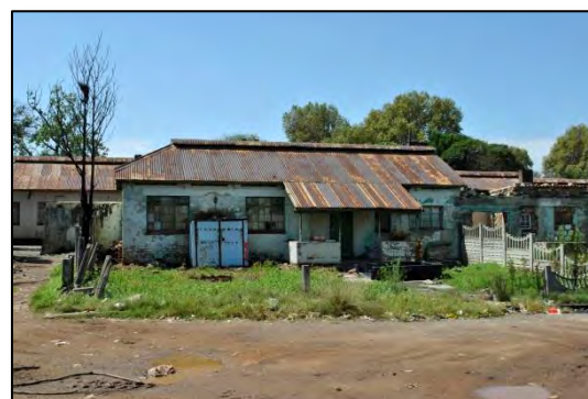
Figure 11-2: Example of remaining house at the Durban Roodepoort Deep Mining Village
