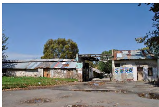
Figure 11-1: Entrance to Durban Roodepoort Deep Mining Village
