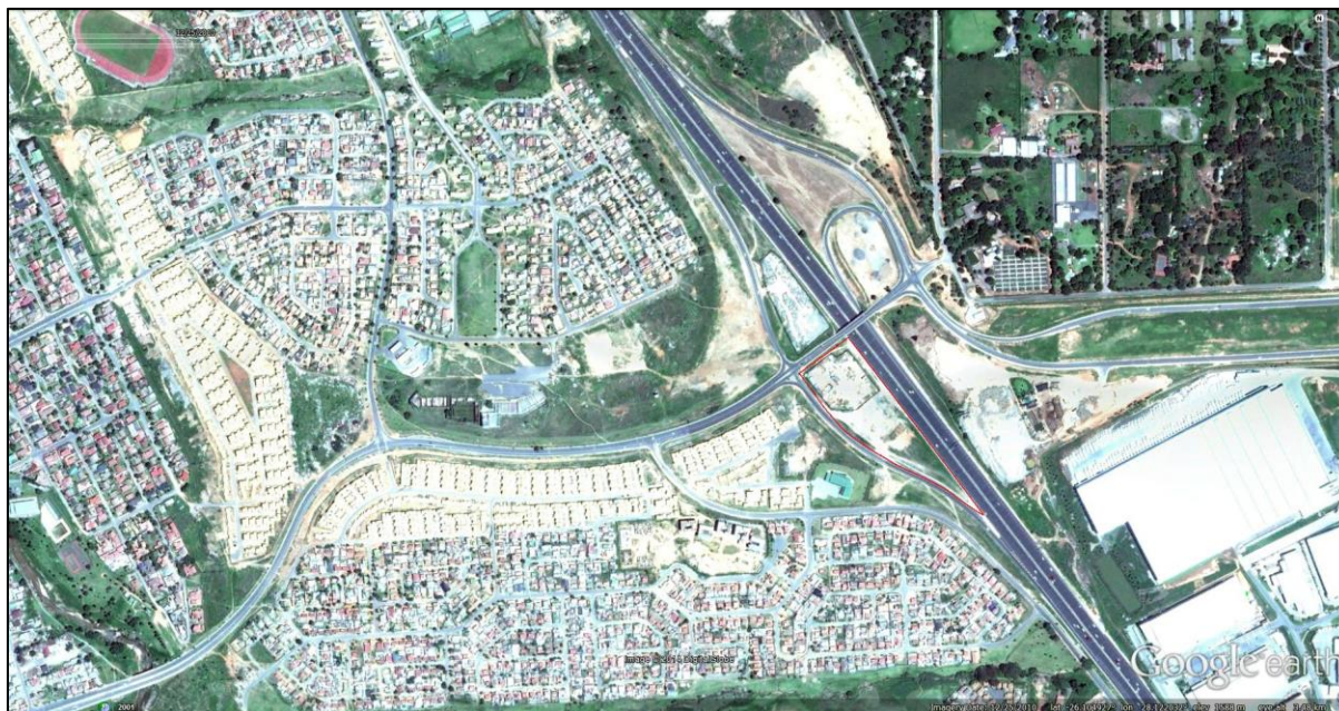
Figure 5-5: Aerial view of London Road/N3 off-ramp in 2010 (Google Earth, 2014)
