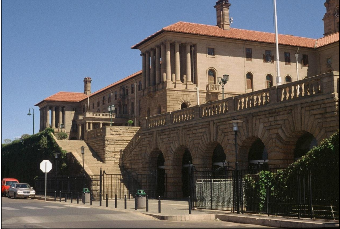
Figure 18: A similar pattern emerges in Baker's work with the simple rectangular floor plan pushed backwards by adding a pavilion at each side of the front elevation - here applied at the Union Buildings but also applied at the ERPM housing units in minute scale.
