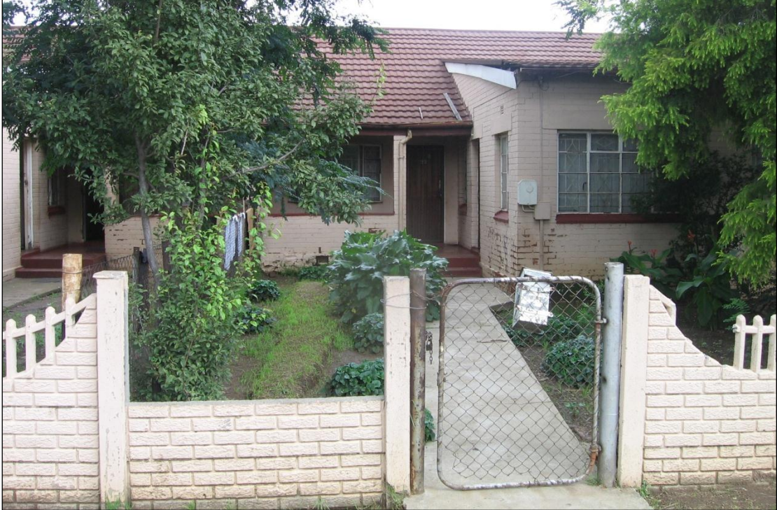
Figure 9: The front elevation and garden of one of the existing units from the old married quarters. This unit is number 22.
