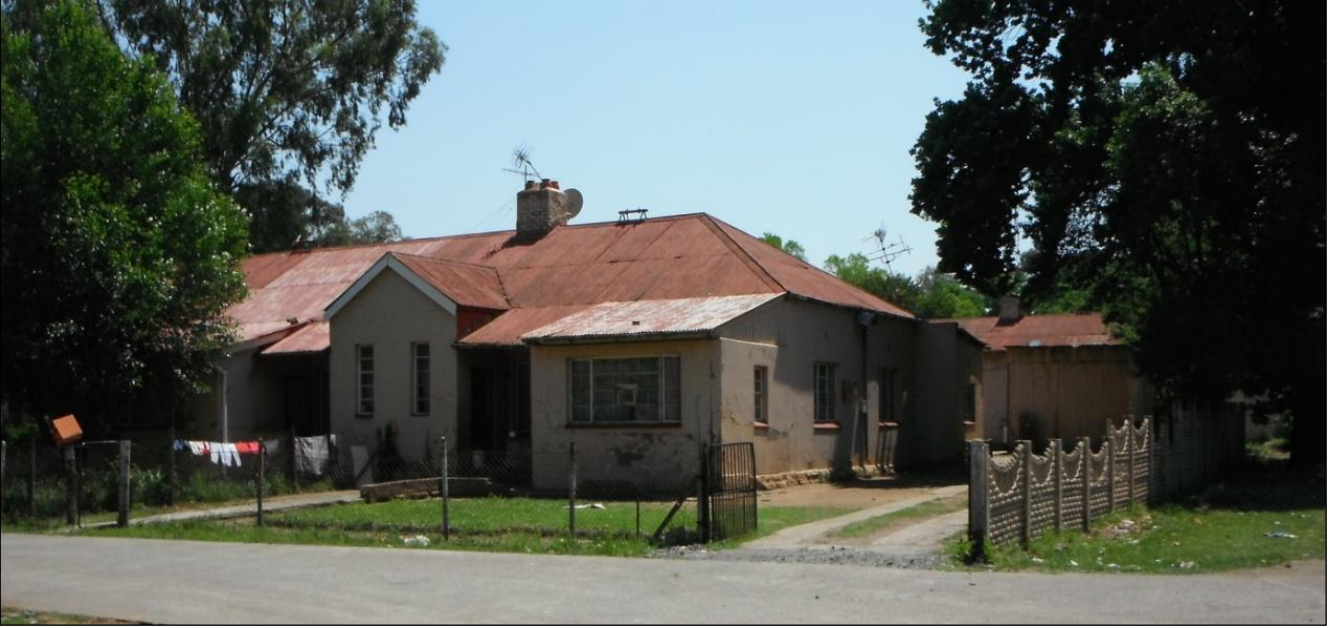
Figure 28: General view of the front and side facades of the first type of dwelling building in Precinct 2.
