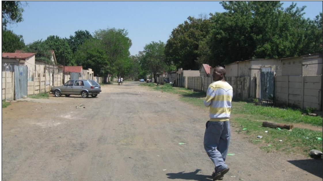
Figure 44: General view along service street running between backyards of residential units.
