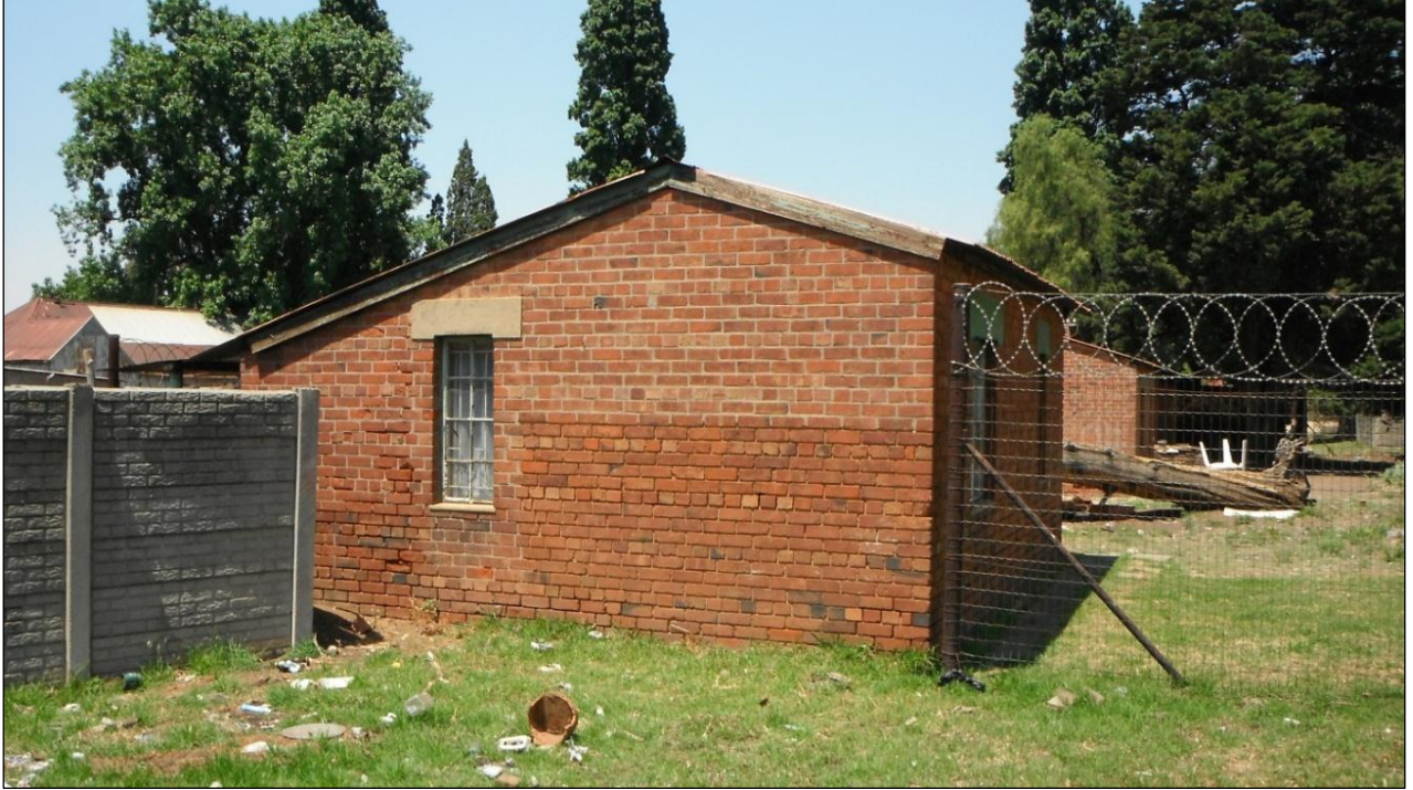
Figure 34: One of the two dwelling types representing some of the earliest buildings from Precinct 3. This type comprises unplastered red face-brick walls.
