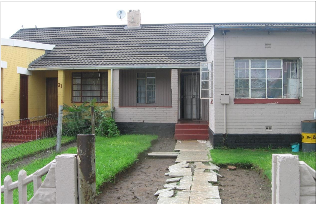
Figure 10: The front elevation and garden of another one of the existing units from the old married quarters. This unit is number 32, with unit 31 to the left.
