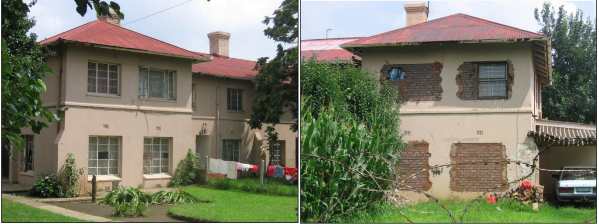
Figure 20: Second generation steel frame windows (left) are replaced by the current residents.
