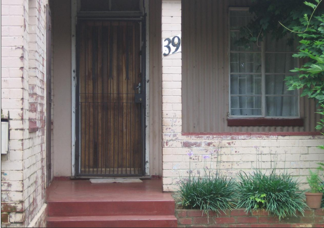
Figure 11: The front veranda of one of the existing units from the old married quarters. This unit is number 39. The corrugated iron sheeting on the walling next to the door can clearly be seen. As discussed elsewhere the corrugated sheeting must have formed part of the original structure.
