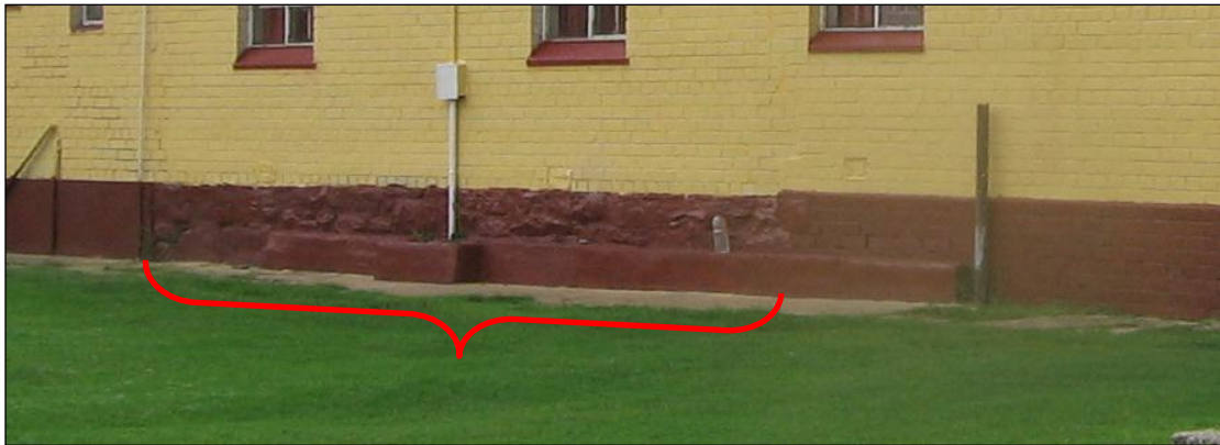
Figure 8: Side elevation of one of the existing buildings from the old married quarters. The enlarged image (bottom) clearly shows the original stone foundation. The stone foundation is marked in red.
