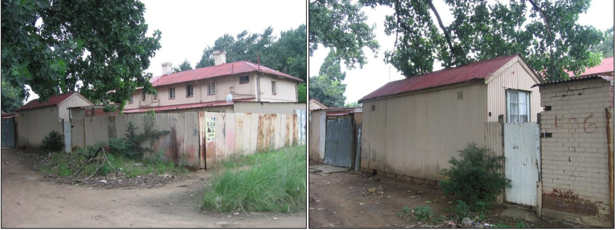
Figure 25: Exterior of backyard walling and small timber and iron outbuilding.
