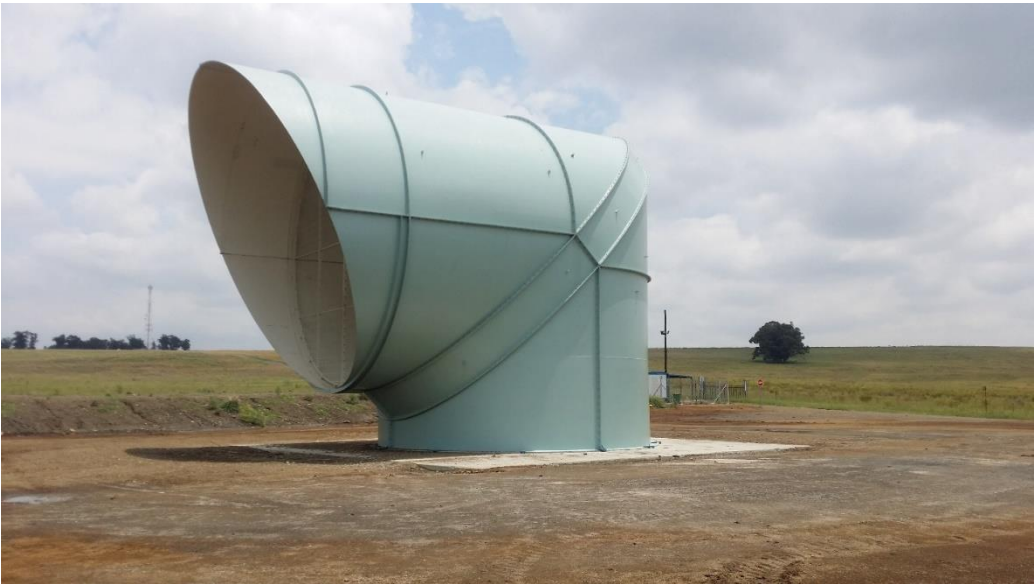
Figure 1-4: Surface infrastructure associated with a down-cast shaft
