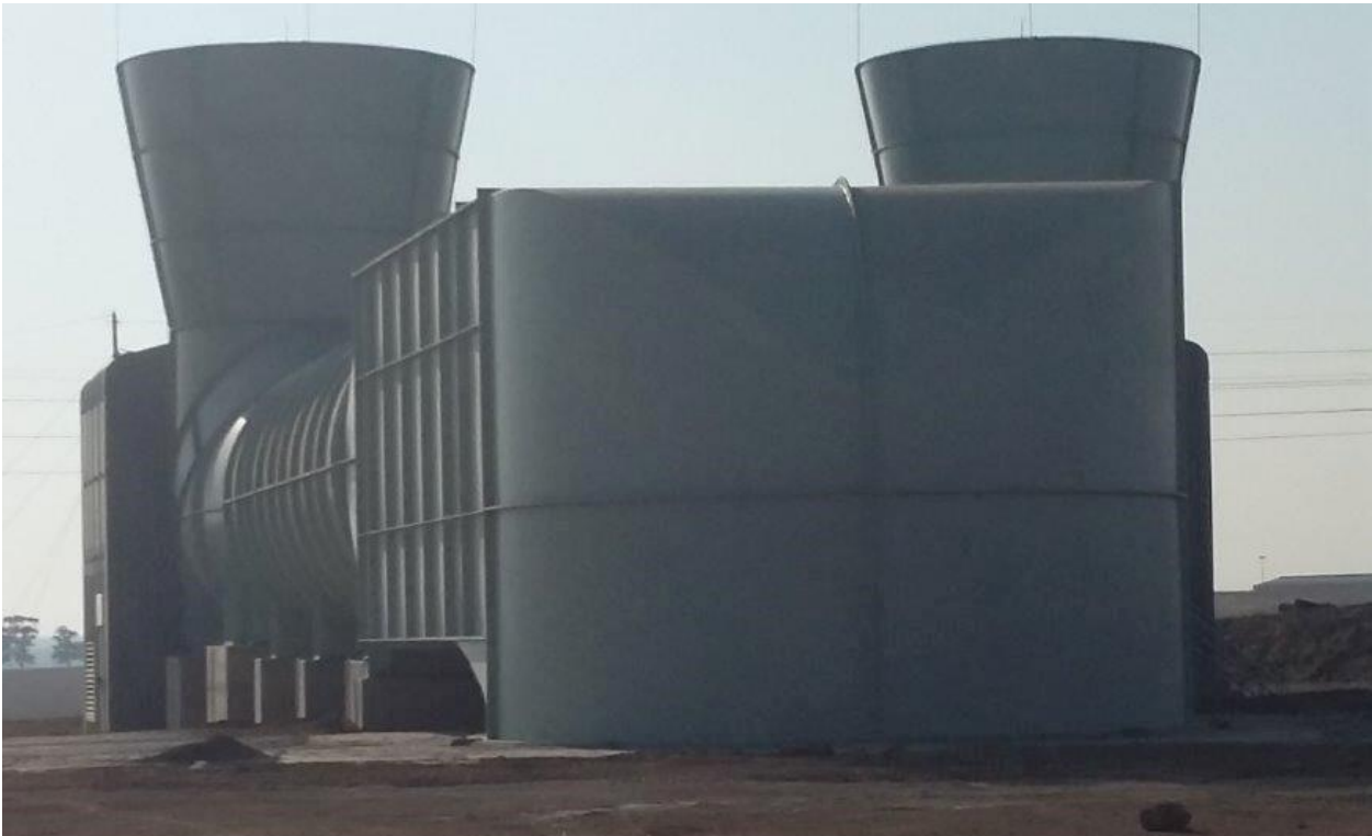
Figure 1-5: Example of completed up-cast ventilation shaft (Height 12-15m)
