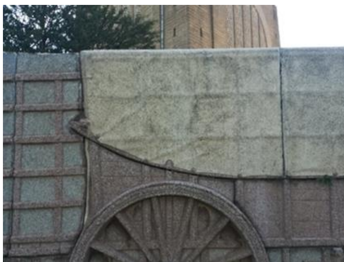
Figure 11: Seals removed after curing and before grouting and pointing.
