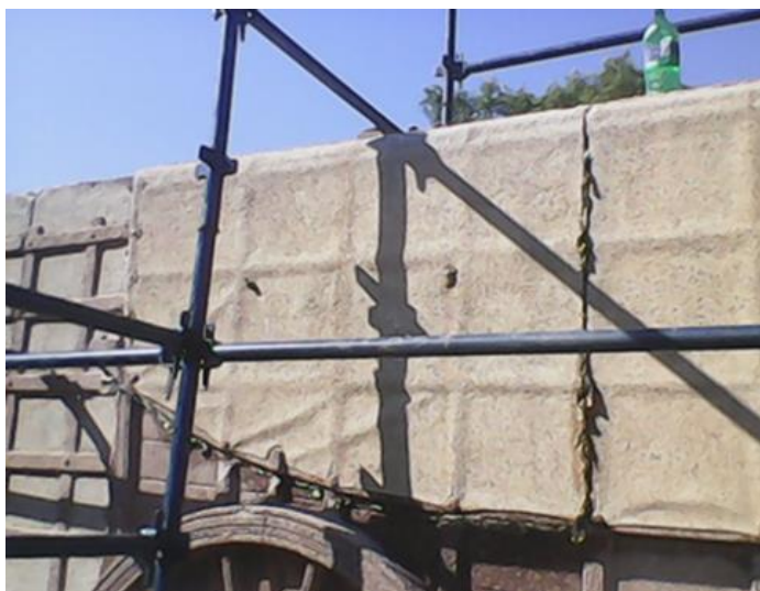
Figure 10: Step 2 – Wet newspaper inserted into joints as temporary seals.
