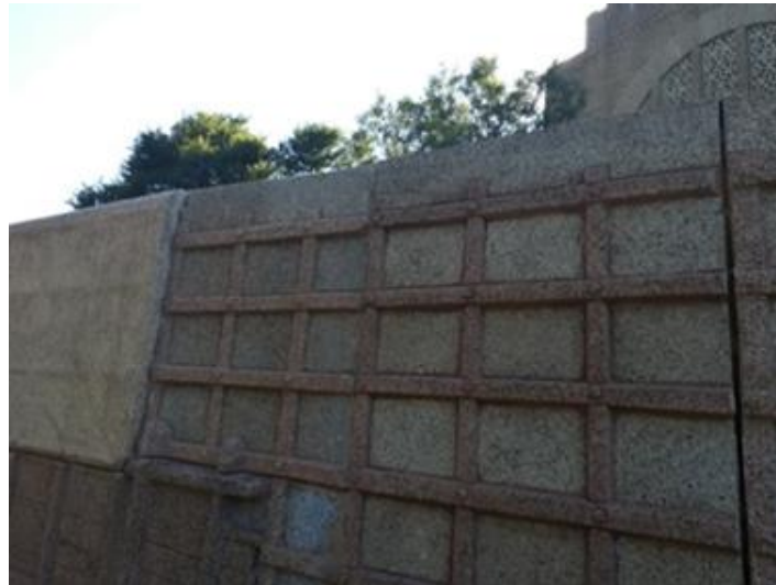
Figure 8: Step 1 – Opening of old joints around panels.
