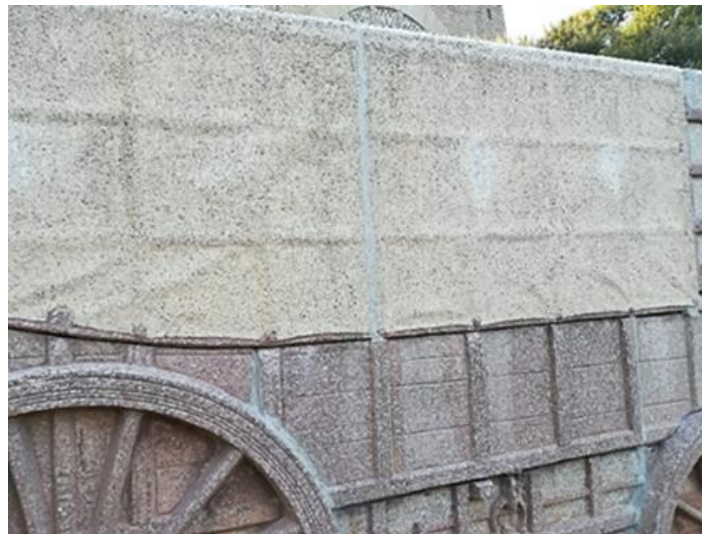
Figure 12: Example of final grouted and pointed joints.
