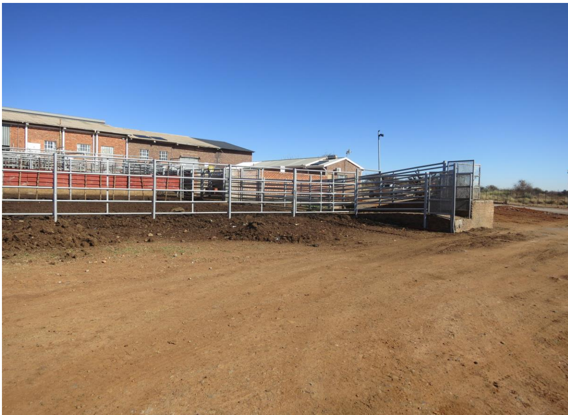
Figure 3: A view of part of the existing Excelsior Abattoir.
