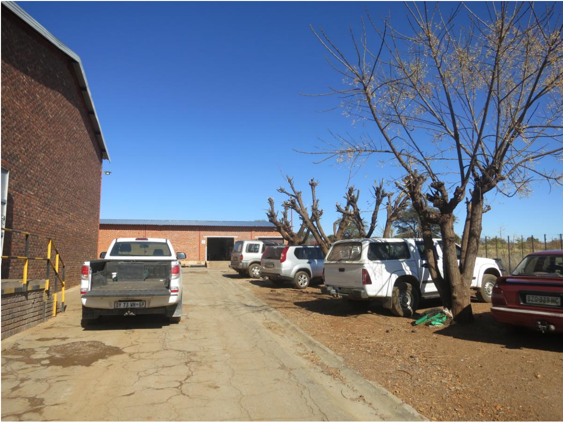
Figure 8: View of the specific area where the existing structures here will be extended.
