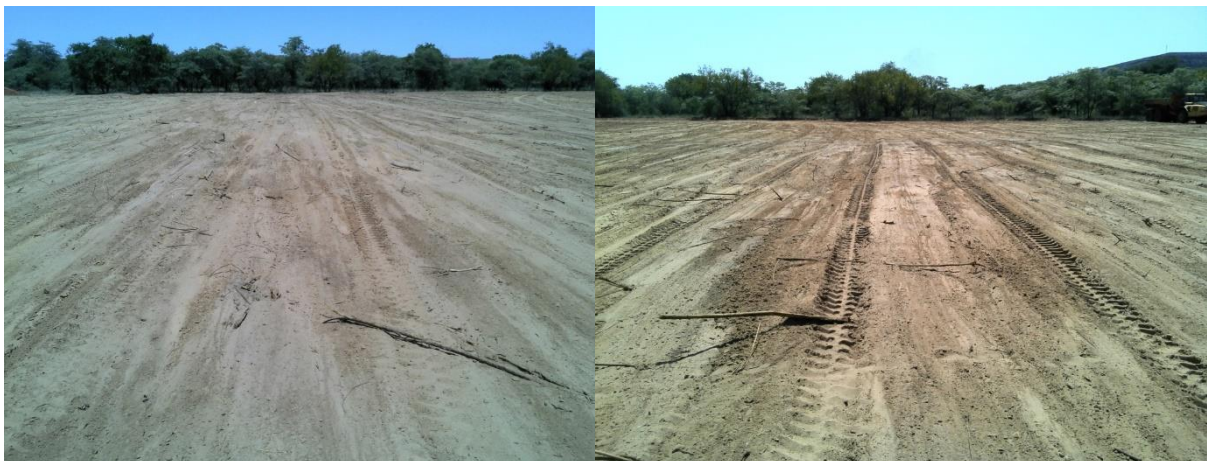
Figure 4-4: Site after clearing and levelling
