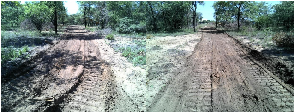
Figure 4-2: Initial strip clearing
