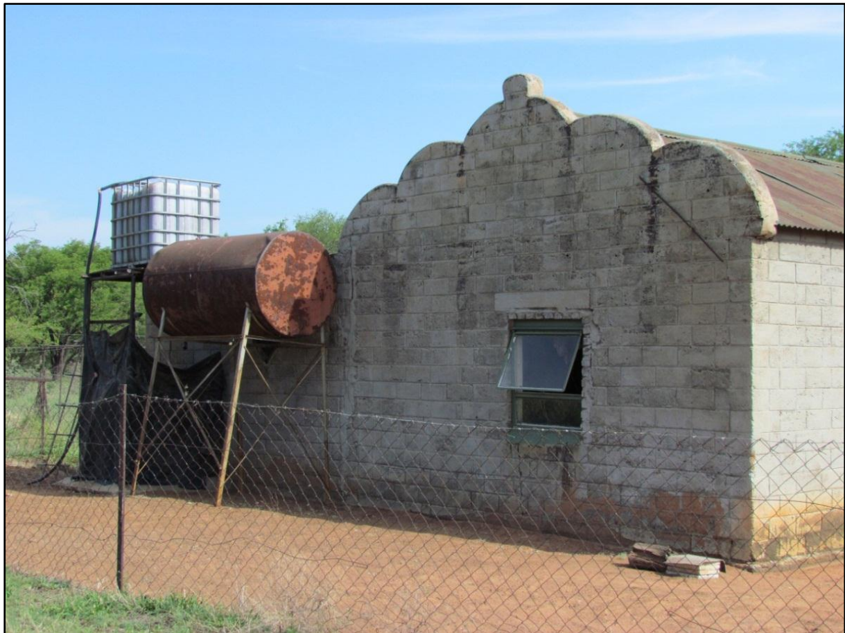
Figure 11-2: Gables and modern fitments (water tank) at Site S.34-001
