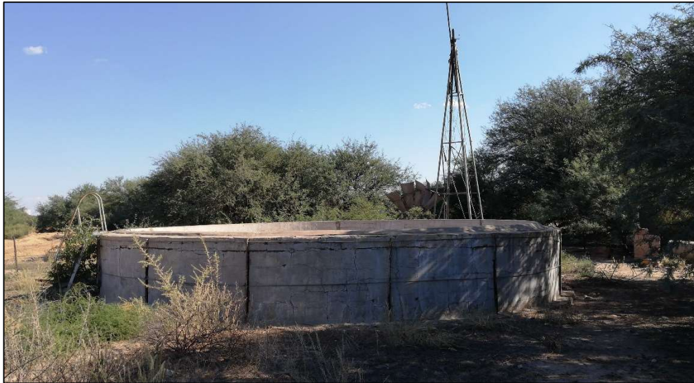
Figure 15: Windpump and reservoir at Site B01.
