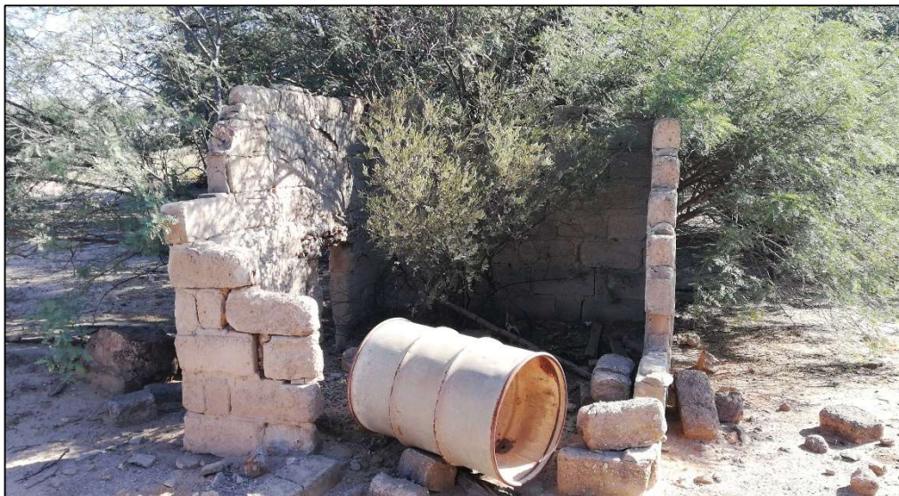
Figure 16: Structure at Site B01.
