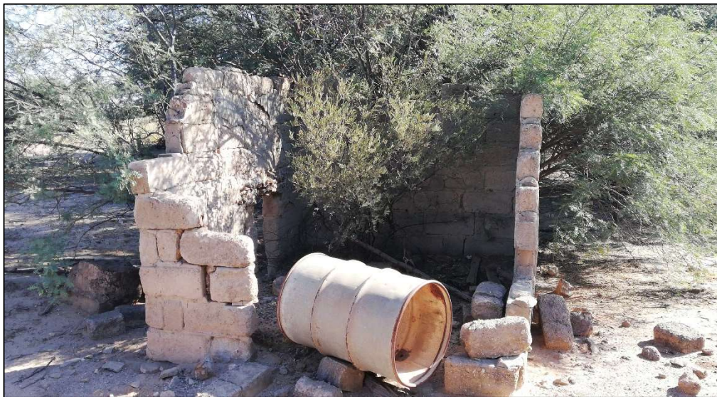
Figure 16: Structure at Site B01.
