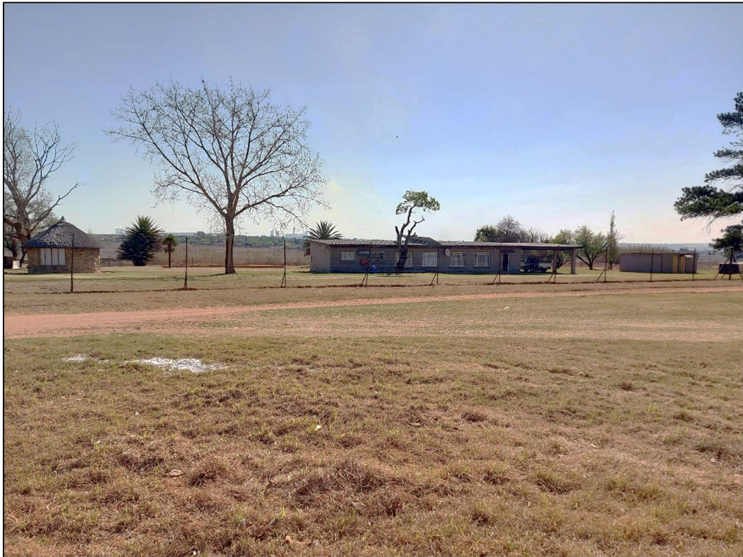
Figure 19: Buildings at Site B02.
