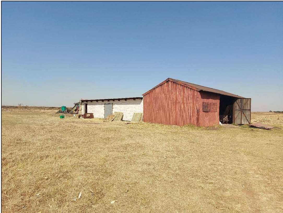
Figure 17: North-western aspect of building at site B01.
