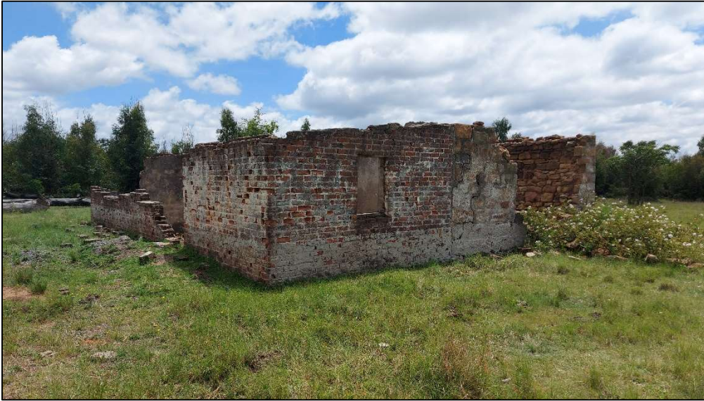
Figure 23: Site B03 seen from the southeast.
