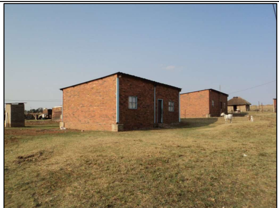
Figure 59: K08 – Old brick buildings.
