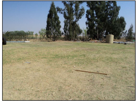
Figure 65: K01 – Demolished building.
