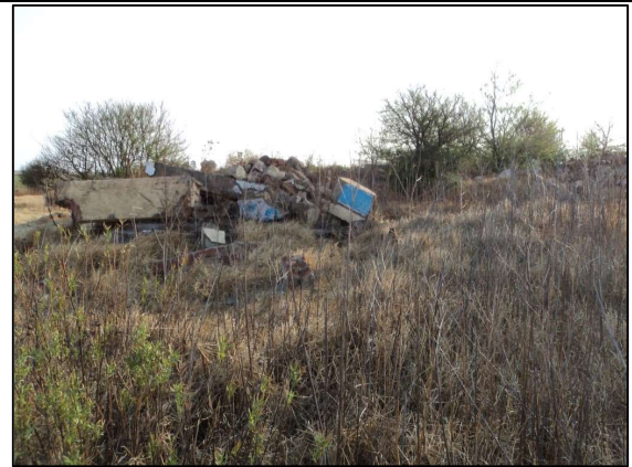
Figure 28: K22 – demolished building.
