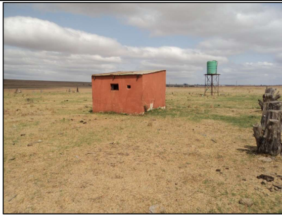
Figure 62: K15 – Outbuilding & eater tank.
