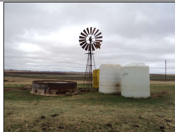
Figure 73: K40 – Reservoir & windpump.
