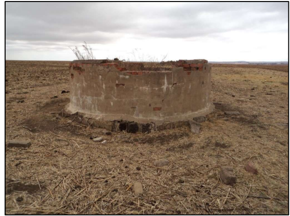
Figure 39: K20 – Circular brick & cement structure.
