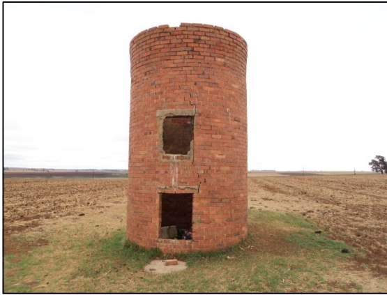
Figure 38: K20 – Brick structure.
