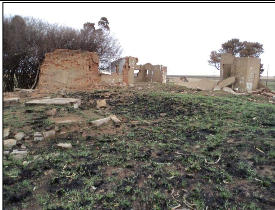
Figure 42: K21 – Building ruin.
