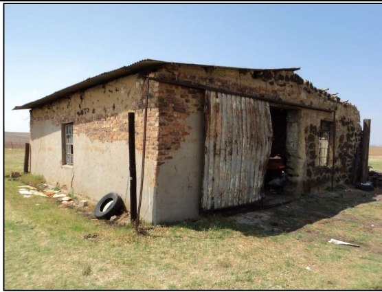
Figure 50: K03 –Stone building repaired using bricks.
