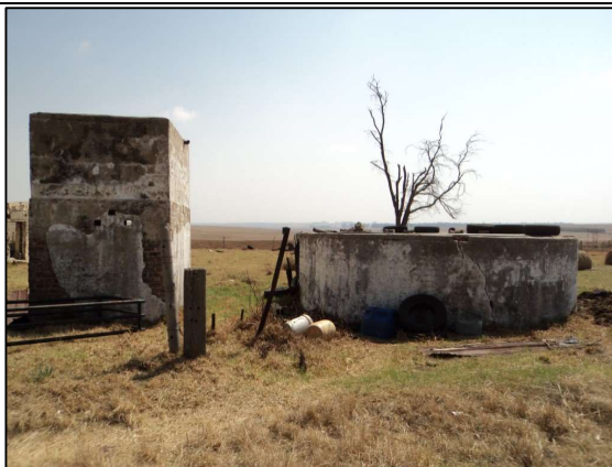
Figure 52: K03 – Angular building & reservoir.
