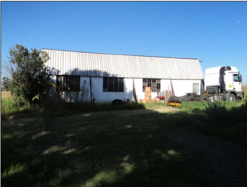
Figure 29: Outbuilding at Site L04.
