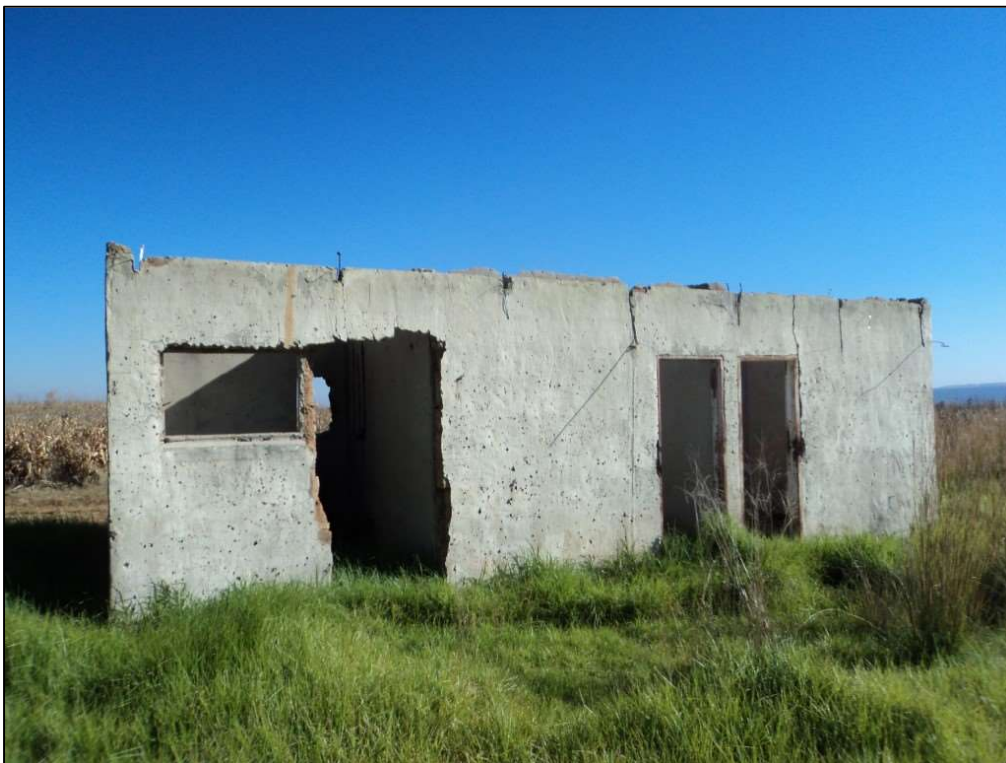
Figure 33: Building ruin adjacent maize field at Site L04.
