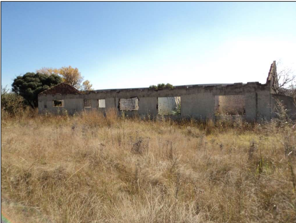
Figure 35: Main building ruin at Site L06 seen from the south.
