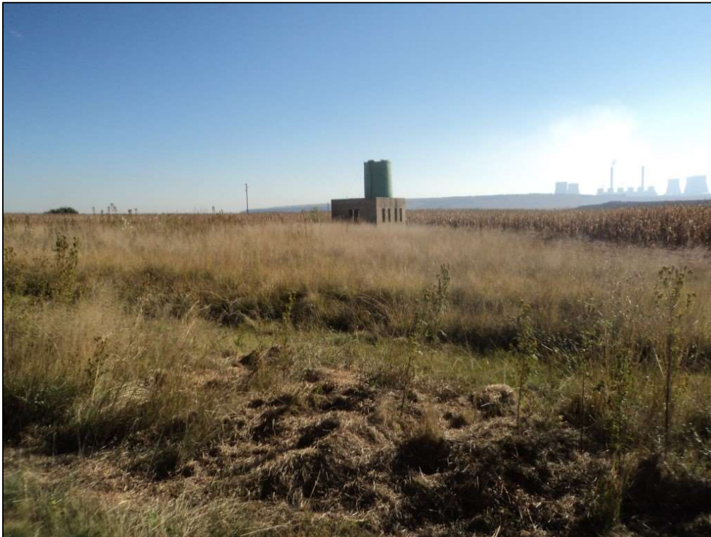
Figure 30: Modern structure with water tank at Site L04.
