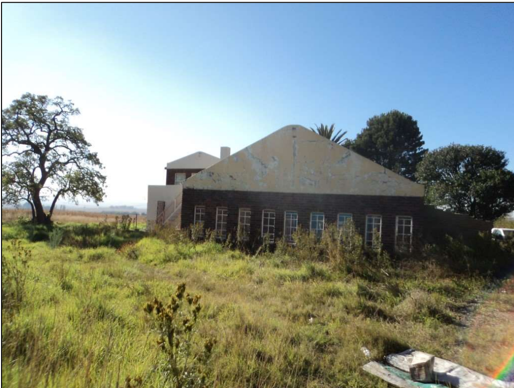
Figure 27: Site L04 – Rear view of the main residence.
