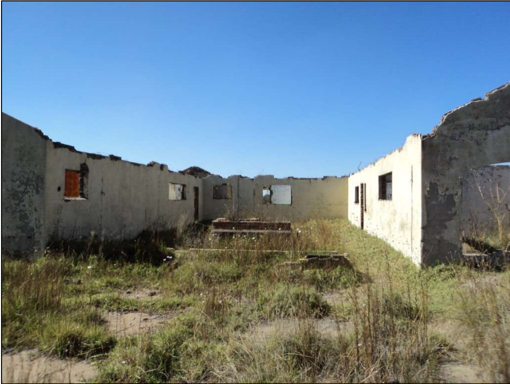
Figure 36: Main building ruin at Site L06 seen from the west.
