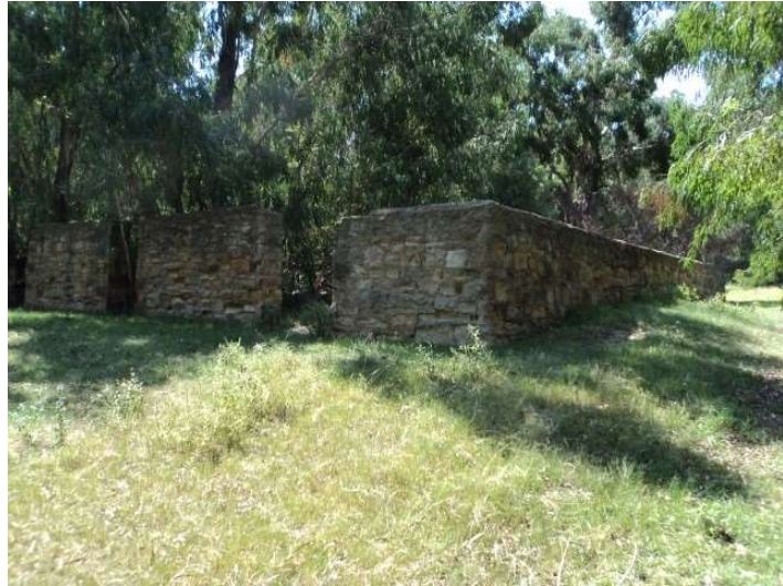
Figure 17: Example of a dilapidated historical kraal.
