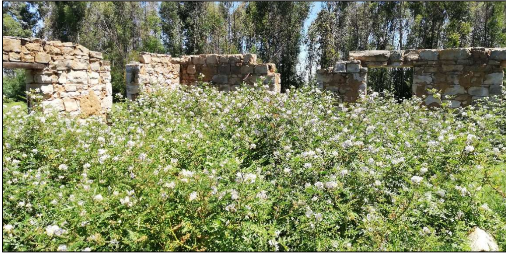
Figure 18: Interior of building ruin at site B04.
