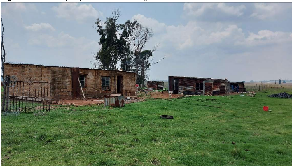
Figure 22: Southern perspective of the building at Site B03.
