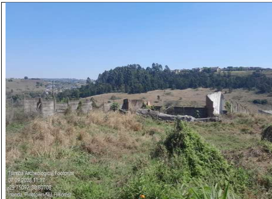
Figure 3: View of the rubbles from the old servant's quarters
