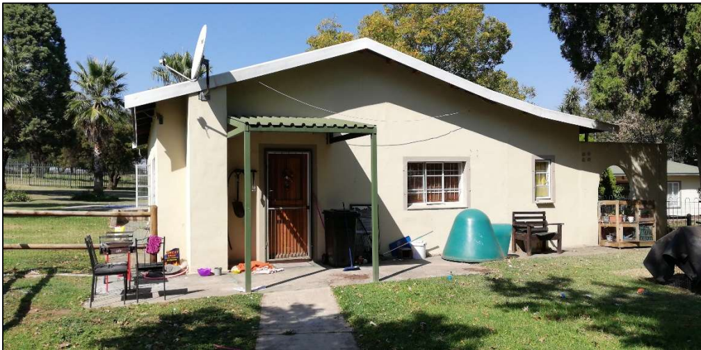
Figure 24: Northern aspect of the eastern building at Site B04.
