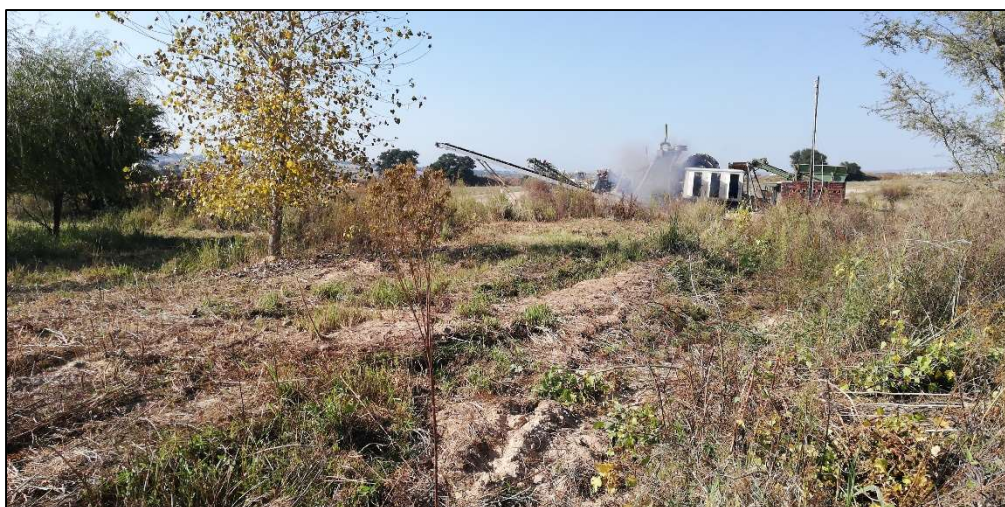
Figure 29: Demolished contemporary Site B06.
