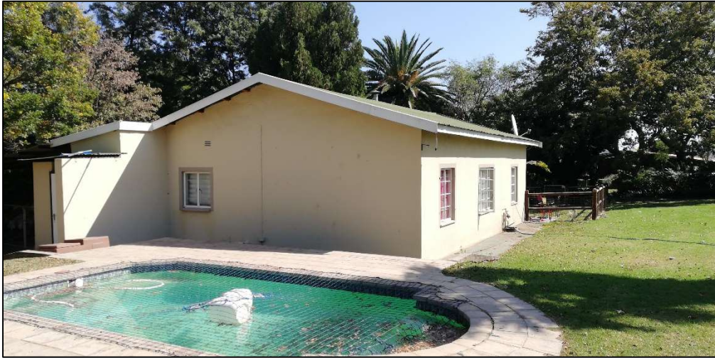
Figure 26: South-eastern aspect of the eastern building at Site B04.
