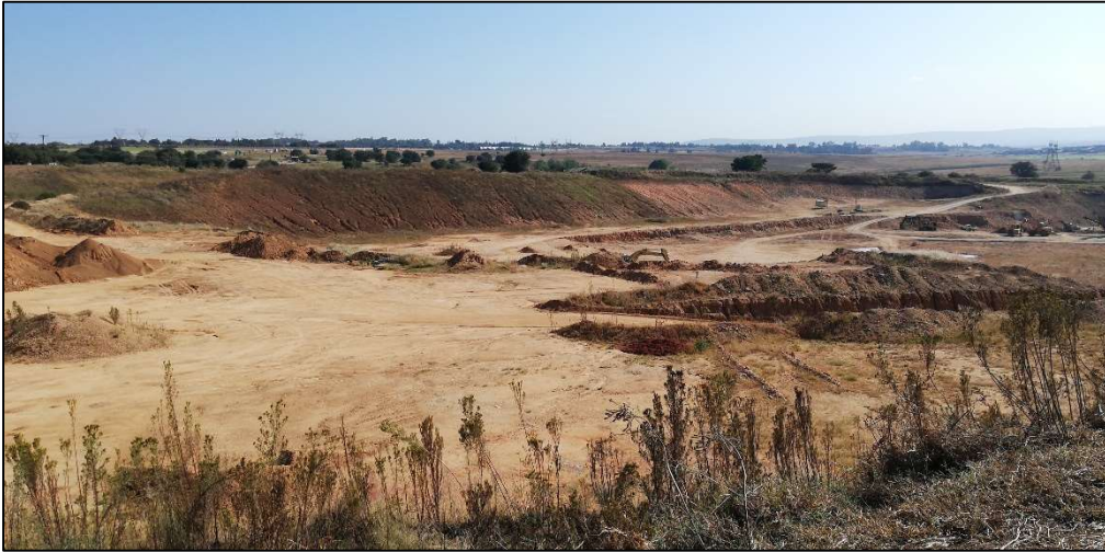
Figure 17: Demolished Site B01 towards the north.
