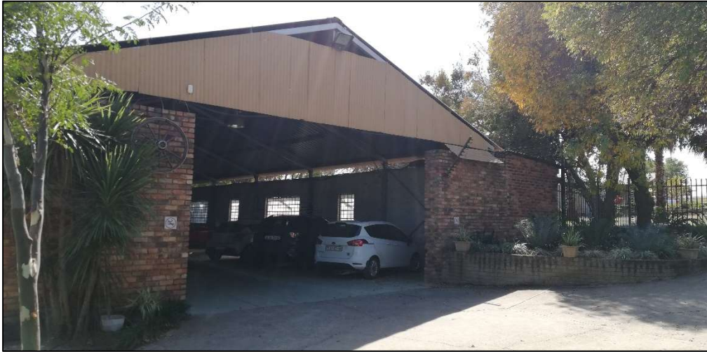
Figure 33: Modern building – garage.
