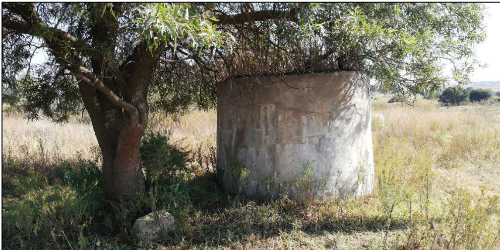
Figure 31: Water tank platform at Site B08.
