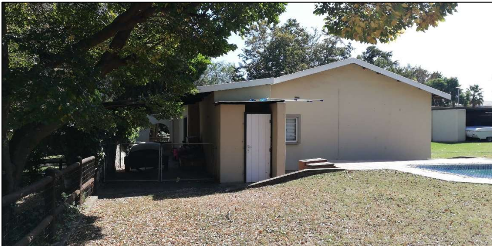
Figure 27: South-western aspect of the eastern building at Site B04.
