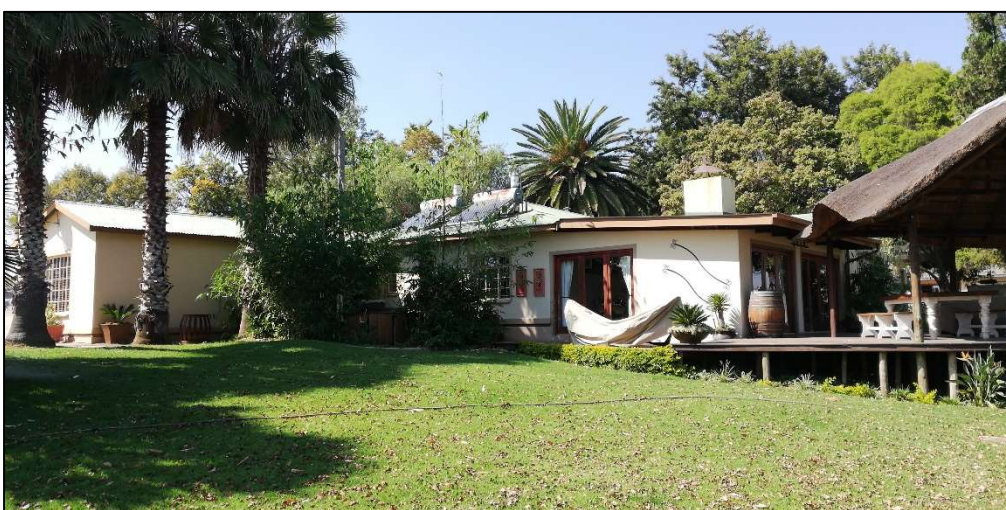
Figure 22: North-western aspect of the western building at Site B04.
