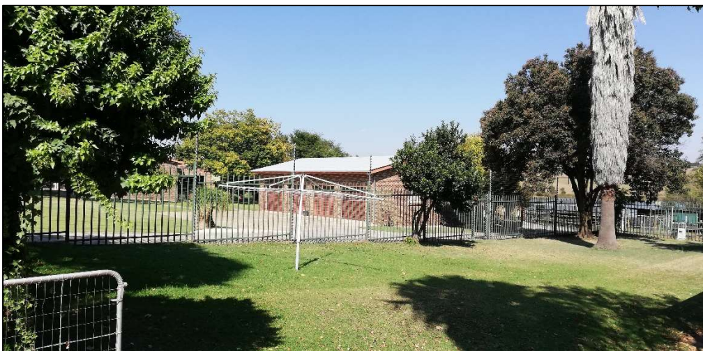
Figure 32: Modern residential building.
