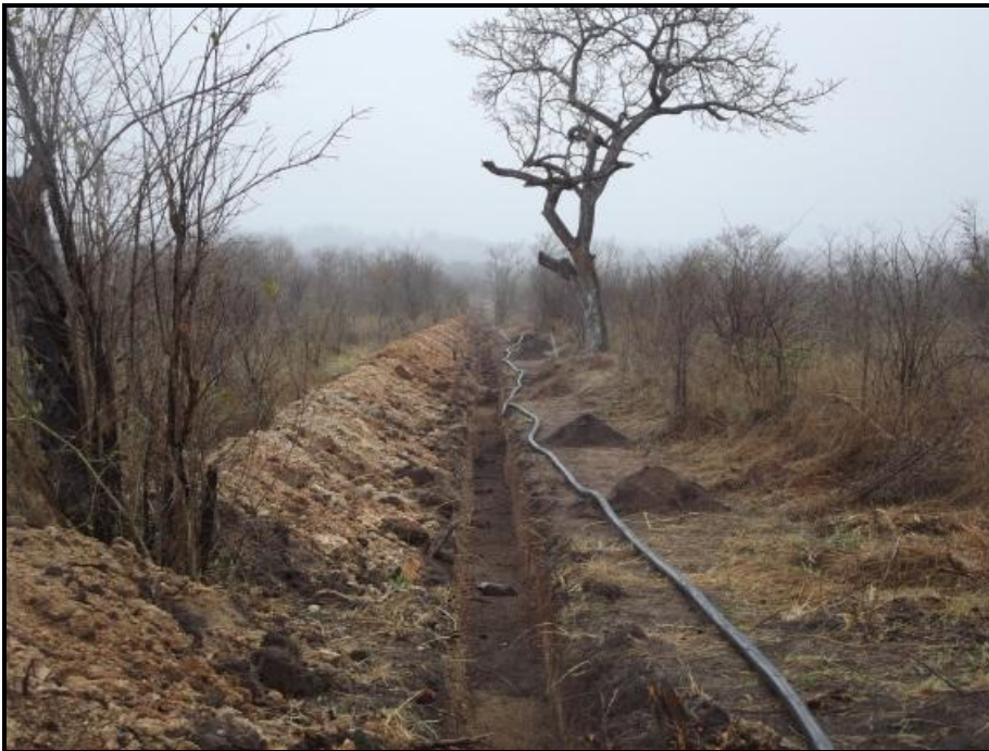
Fig. 4. The same position as fig. 3. Photo taken in Eastern direction.
