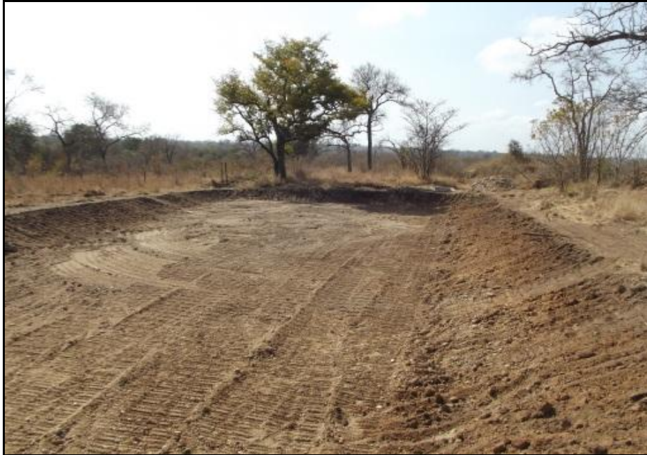
Fig. 9. Groundworks in preparation for foundation. Photo taken East.
