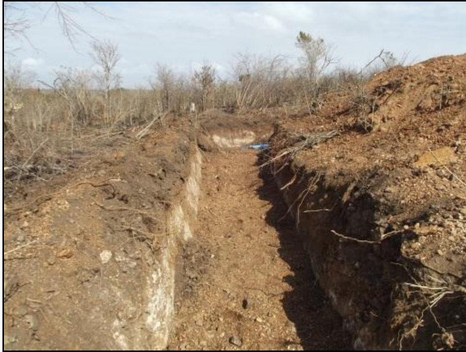
Fig. 7. A small section of the water supply line monitored on Aug 18, 2012.
