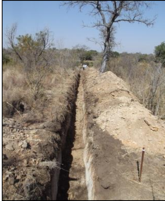
Fig. 3. A sewage line running in a southern direction. Inspected on Aug 3, 2012.
