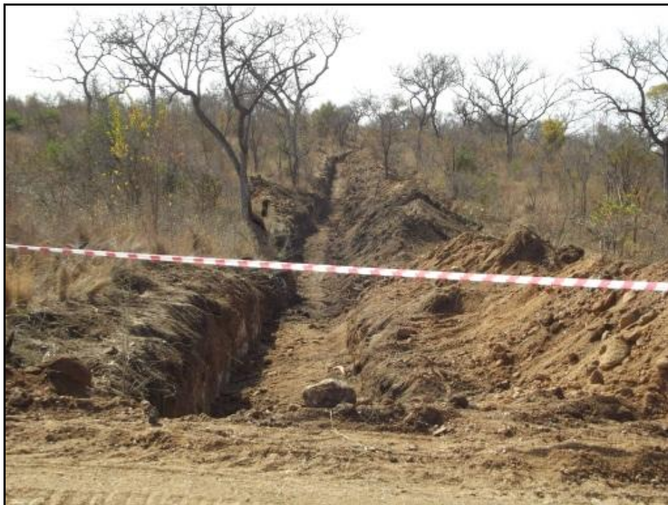
Fig. 8. The water supply line continues in an eastern direction.
