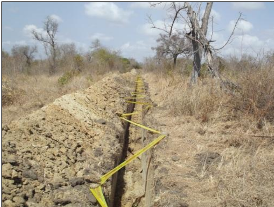
Fig. 10. Continuation of the electric cable trench. Monitored on Aug 18, 2012.
