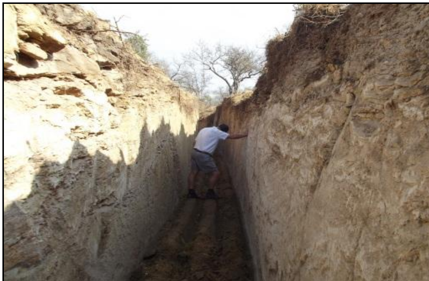
Fig. 6. Sewage trench monitored on Aug 18, 2012. Photo taken west.
