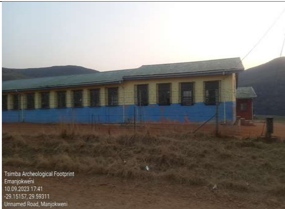
Figure 8: A closer view of the Manjokweni Primary School
