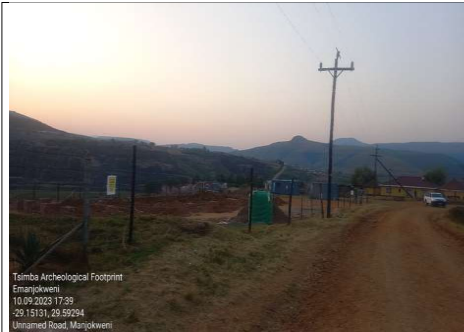
Figure 6: View Of an access road to the site
