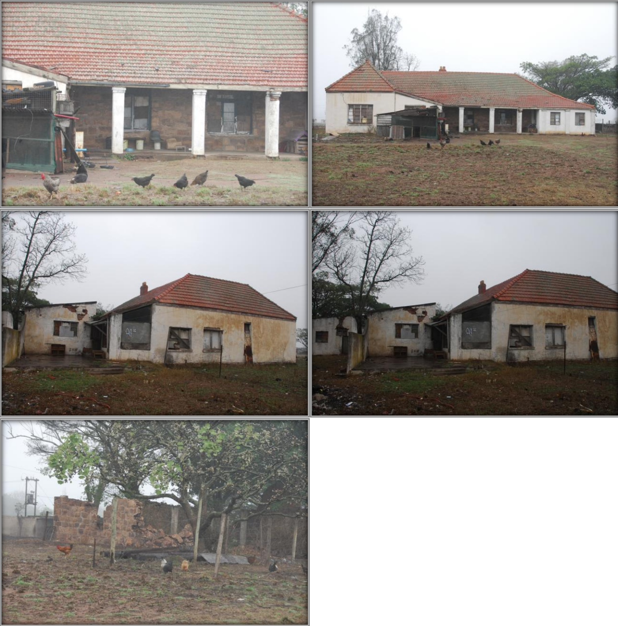
FIGURES 9-13 VIEWS OF BUILDING 1 AND OUTBUILDINGS.
