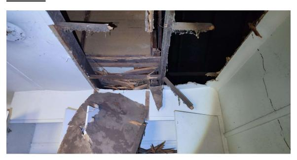
The supports to the first floor have been severely damaged. The current floor is unstable and will need to be removed before any loading or occupation can occur. This is a hazard as many of the support beams and rafters have been damaged.
