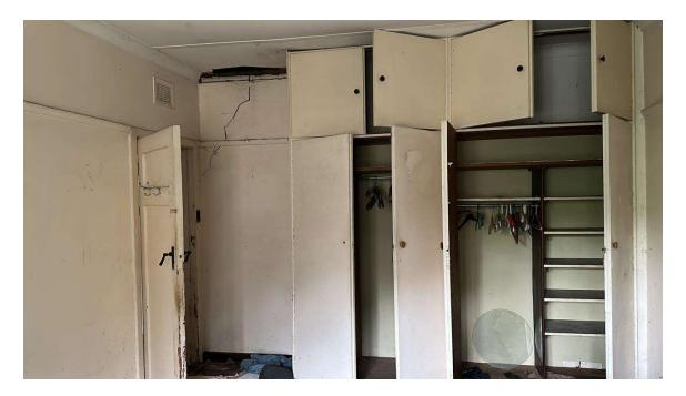
In this room another structural cracks was noticed. The location of this is an internal wall. This is the staircase adjoining wall. This crack has a width of 3 mm and runs the length of 600~mm.
