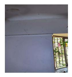
In this room three structural cracks were noticed. As this is a corner room with two external walls , two of the cracks were noticed on external walls and one on an internal wall. These cracks are severe with a width of 2 mm to 5 mm and running the length of 500 mm to 1000 mm. The locations of these cracks led me to believe that they are not purely simple settlement cracks.
