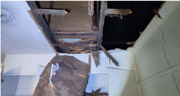
This is the room that partially supports the first floor. Within this room another two cracks were noticed. This ranged from 2 mm to 4 mm wide and runs the length of 500 mm to 1500 mm. The greatest concern of this is that these walls partially
