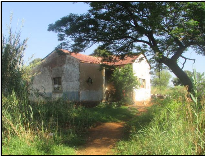
Figure 5: Structure in the study area (Feature 1).
