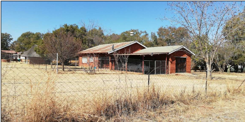
Figure 37: Intact building associated with Site B10.
