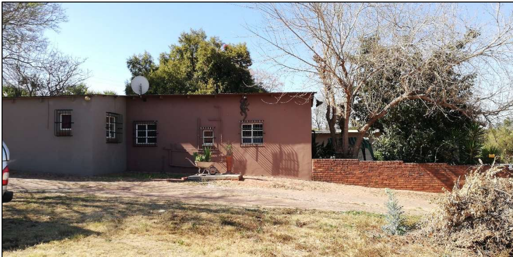
Figure 31: Eastern building associated with Site B07.
