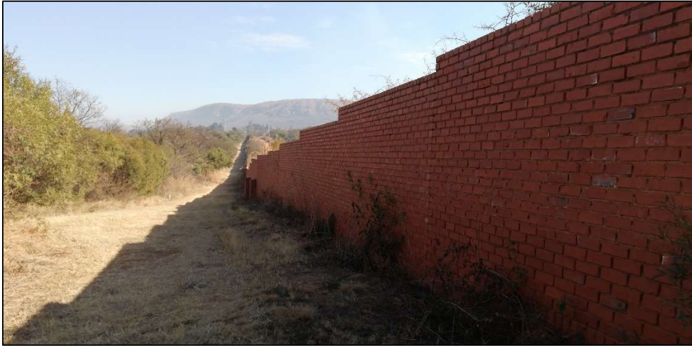
Figure 9: Brick wall along the northern and eastern boundary.
