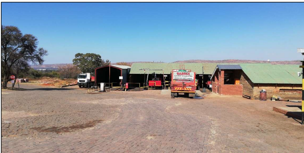
Figure 39: Existing modern SABRIX infrastructure.
