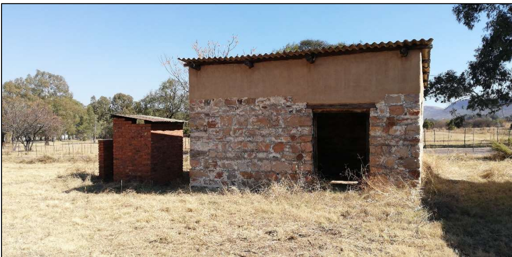
Figure 20: Partially restored building at Site B03.
