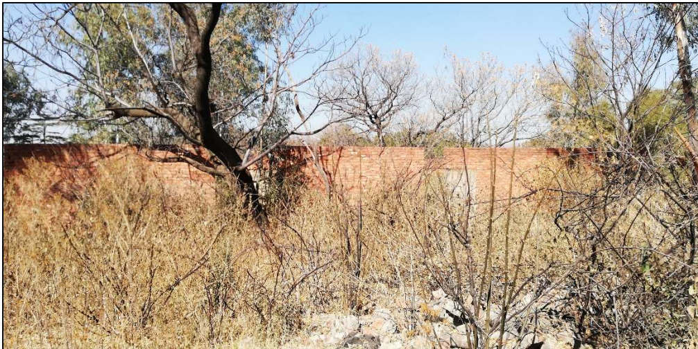
Figure 28: Potentially modern building ruin at the southern boundary of Site B09.
