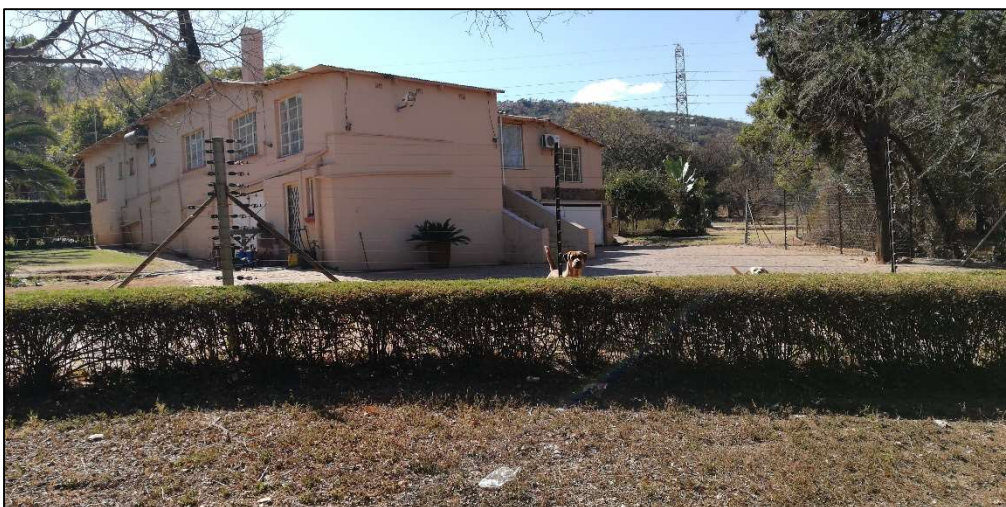
Figure 32: Northern building associated with Site B07.
