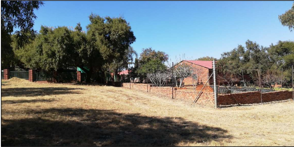
Figure 30: Demolished building at Site B06.
