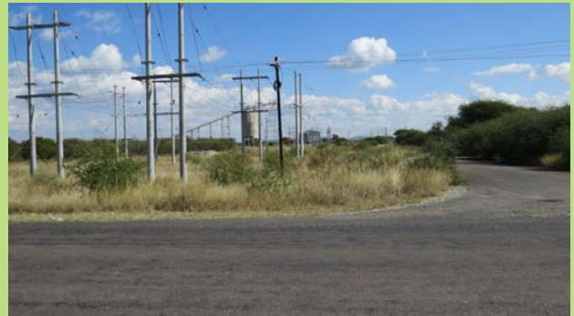
View at site entrance towards west showing transmission line infrastructure and 62 East Decline Shaft in the background.
