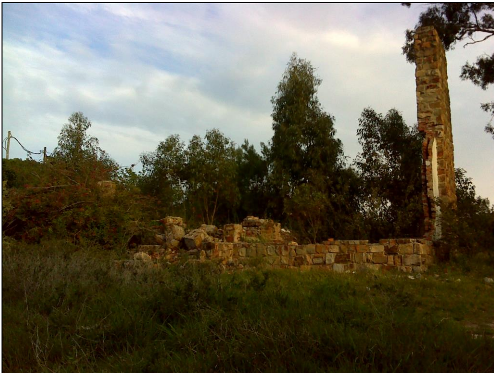
Figure 17. View of the ruins of a farmstead situated at the area marked QBE3.
