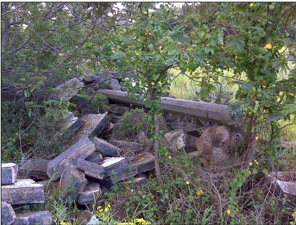
Figure 15. Alternative view of the building ruin situated at QBE2.
