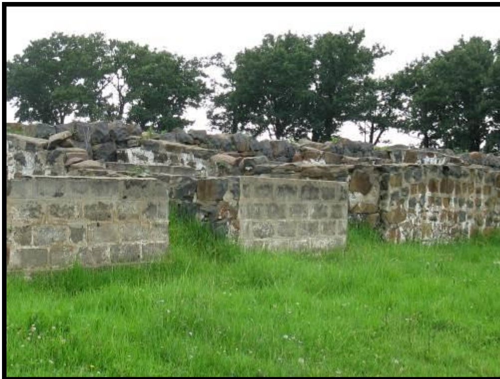
Figure 5. Northern section of the stone walled livestock enclosure
