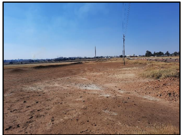
Figure 7.8. Cleared area as a result of the reclamation of the mine dump.
