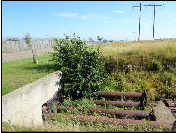
Figure 7.1. The power line follows the existing pipeline.
