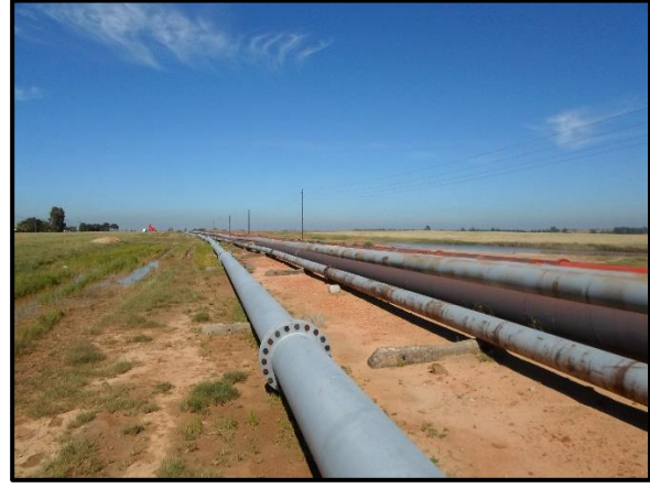
Figure 7.2. The power line follows the existing pipeline servitude.
