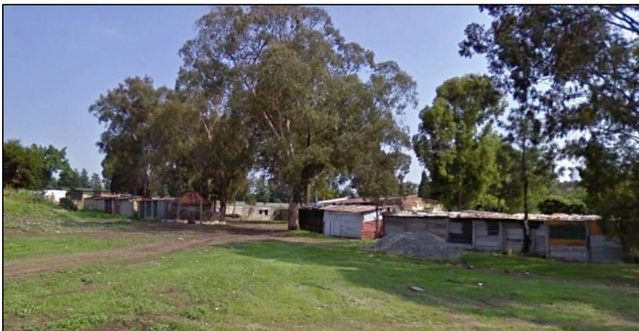
Figure 10. Remains of structure at Site 001
