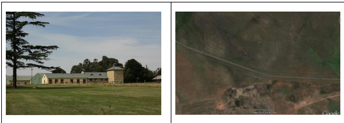
Fig. 15. Nooitgedacht farm and the track of the old railway line.
