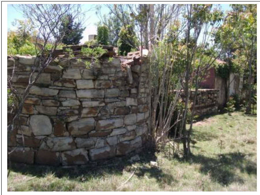
Figure 11- An outbuilding and outer wall constructed with stone is part of HH01 (above).
