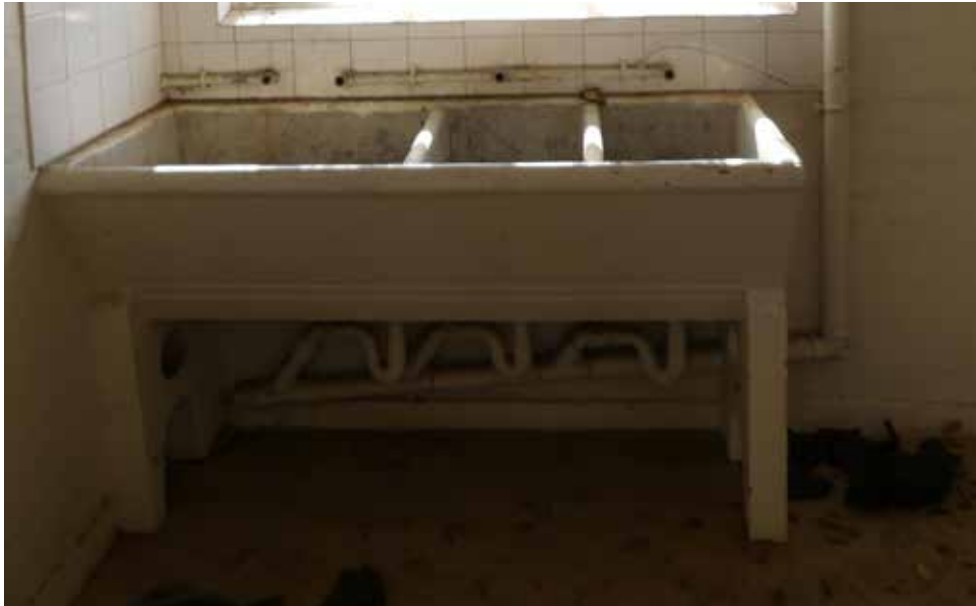
Trough in outbuildings of building 2 - Doctor's House Type 7.
