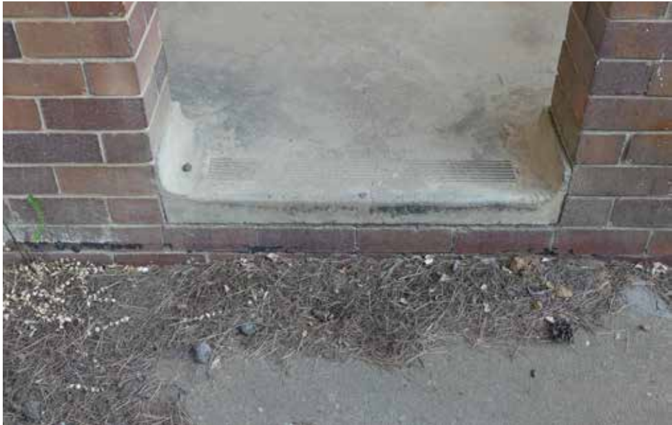
Threshold detail to exterior corridor - building 40.
