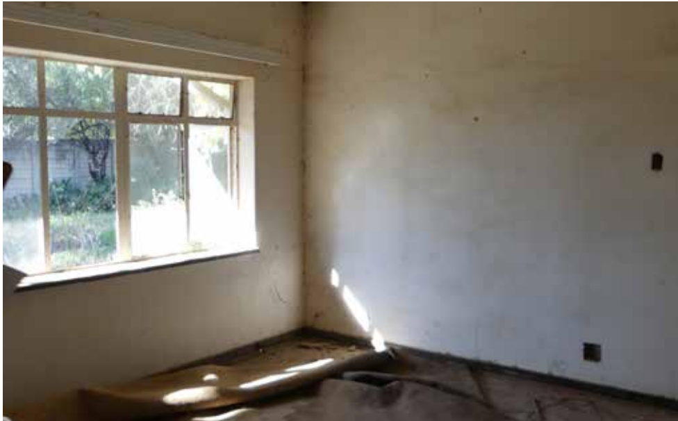
Bedroom in building 7 - Doctor's House Type 6.
