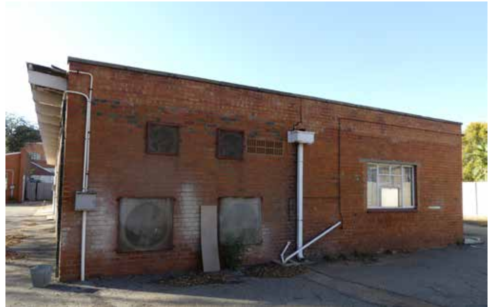
Southern elevation - building 31.
