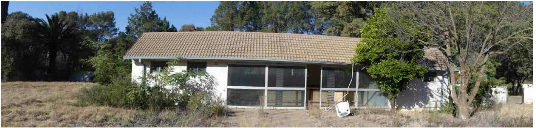
Panoramic view of front of building 11.
