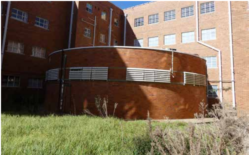
ICU unit - building 17.
