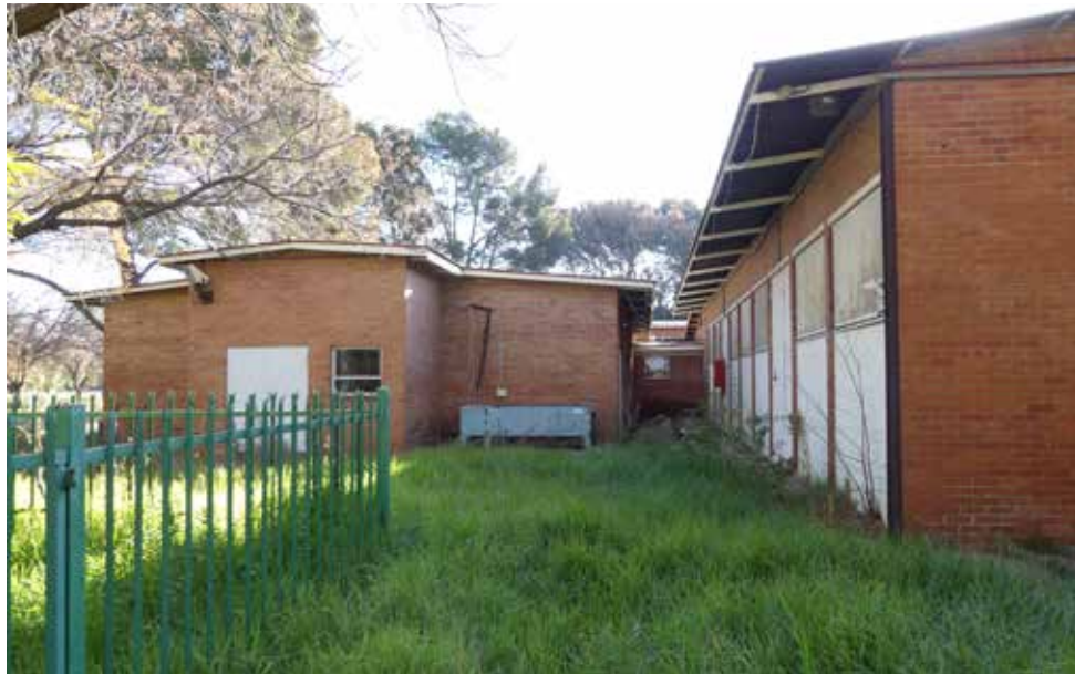
East elevation of building 13.
