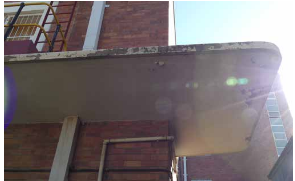
Detail of overhang of Laundry - building 21.
