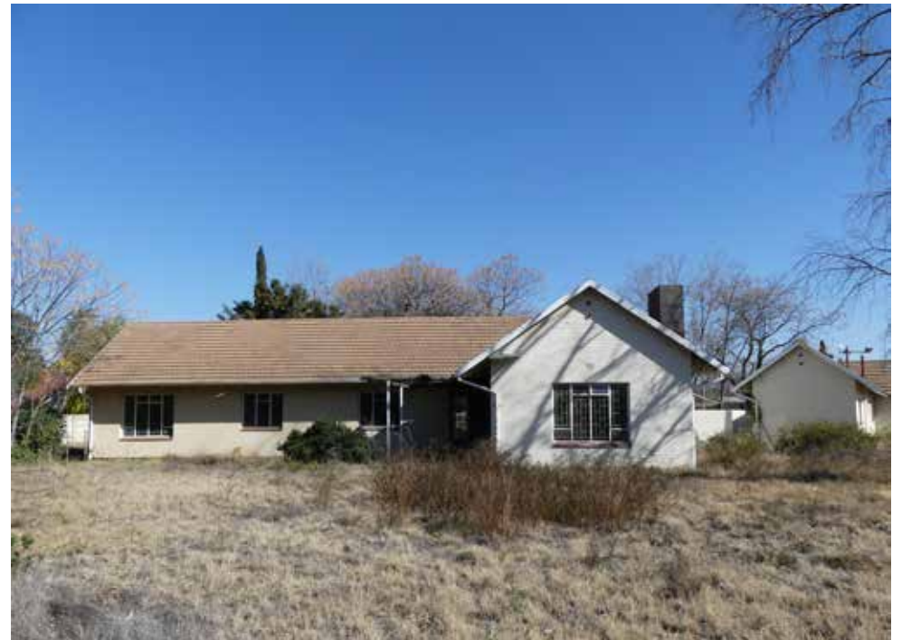
Back elevation of building 2 - Doctor's House Type 7.
