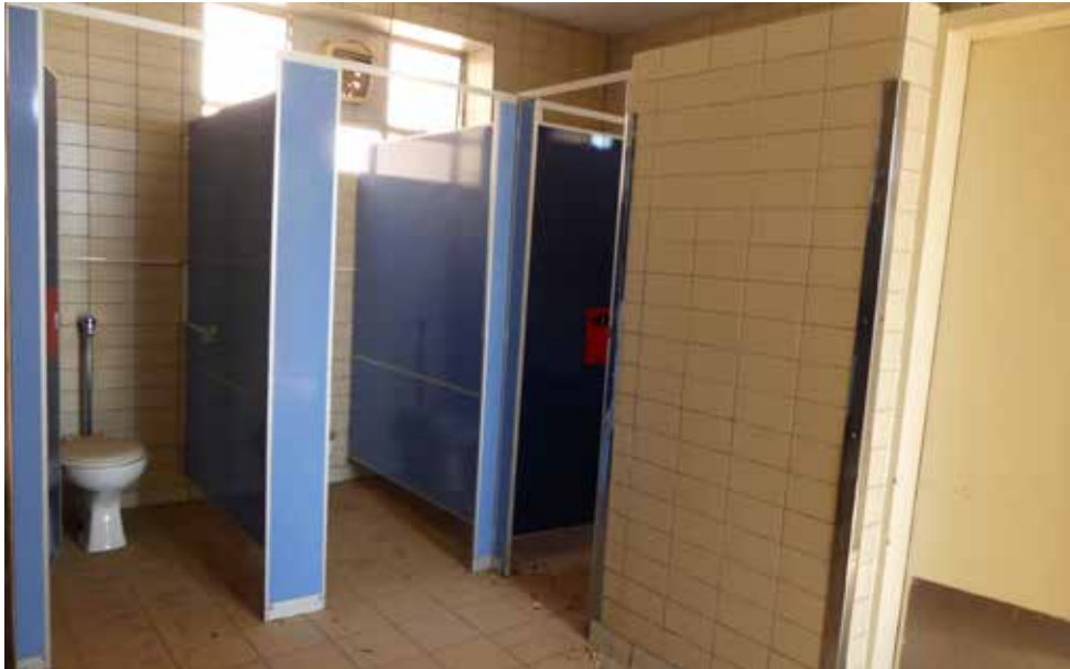
Bathroom to wards - building 17.
