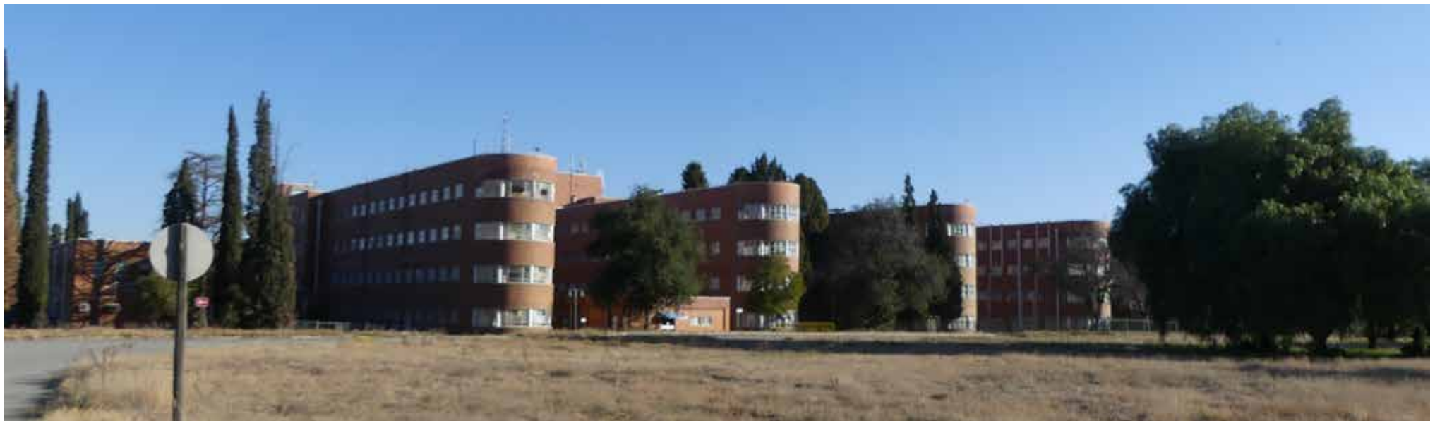
ERNEST OPPENHEIMER HOSPITAL , ERF 7186, REITZPARK, WELKOM, ORANGE FREE STATE: Proposed upgrade of existing facilities - September 2016.
