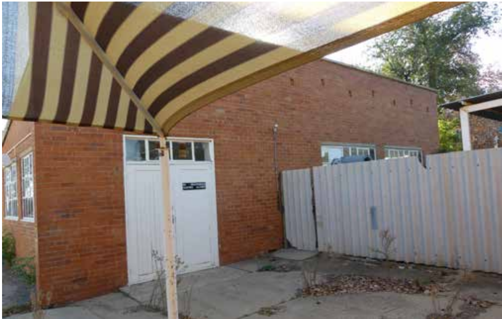
Eastern elevation - building 28.
