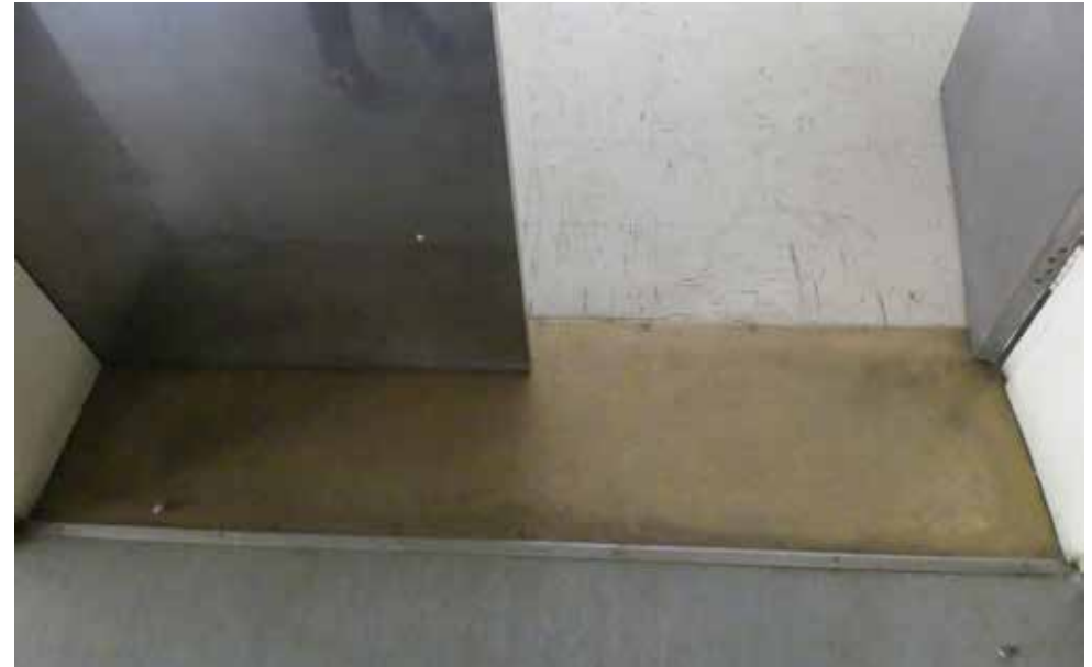
Original brass threshold plate - found in some areas - building 17.
