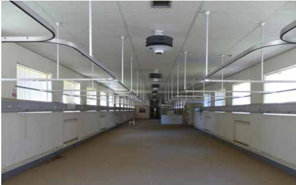
Open ward on the Ground Floor - building 17.
