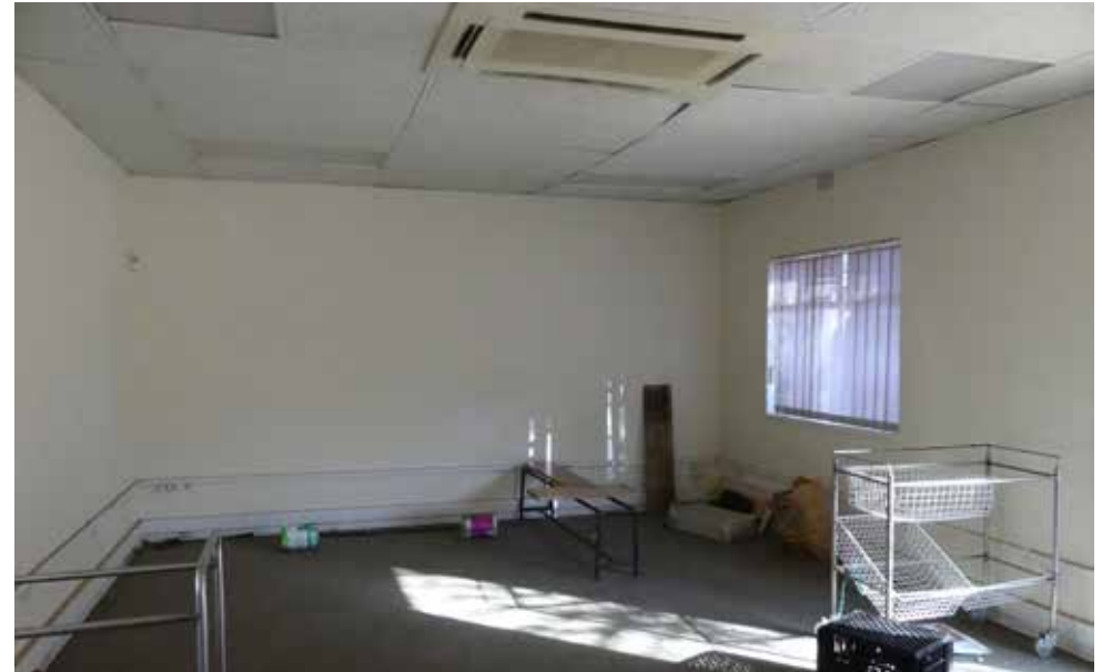
Interior office - building 16.
