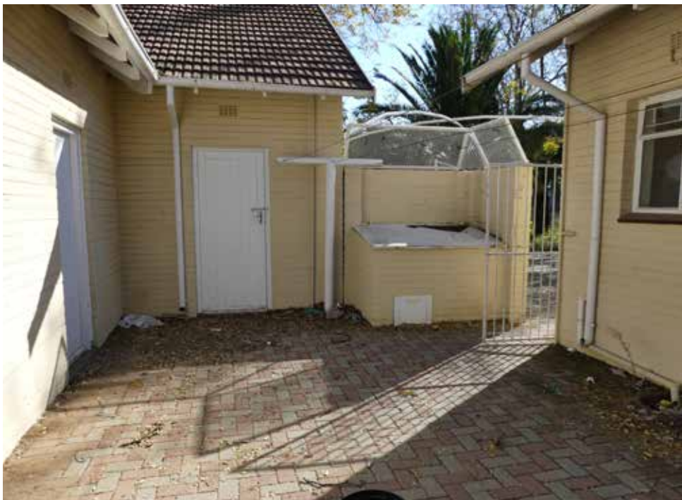
Courtyard of building 6.
