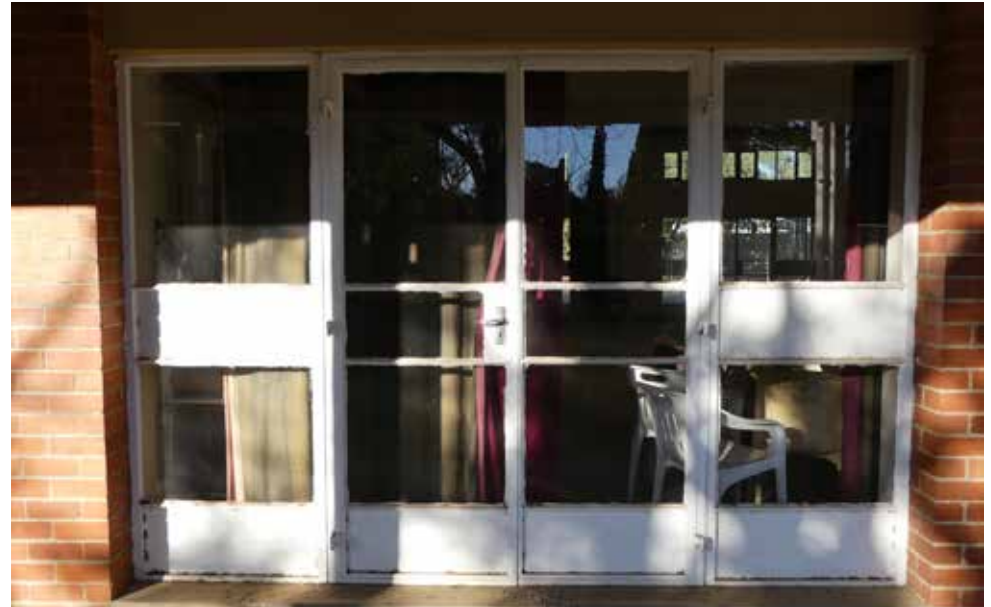
Doors on Western side to building 14.
