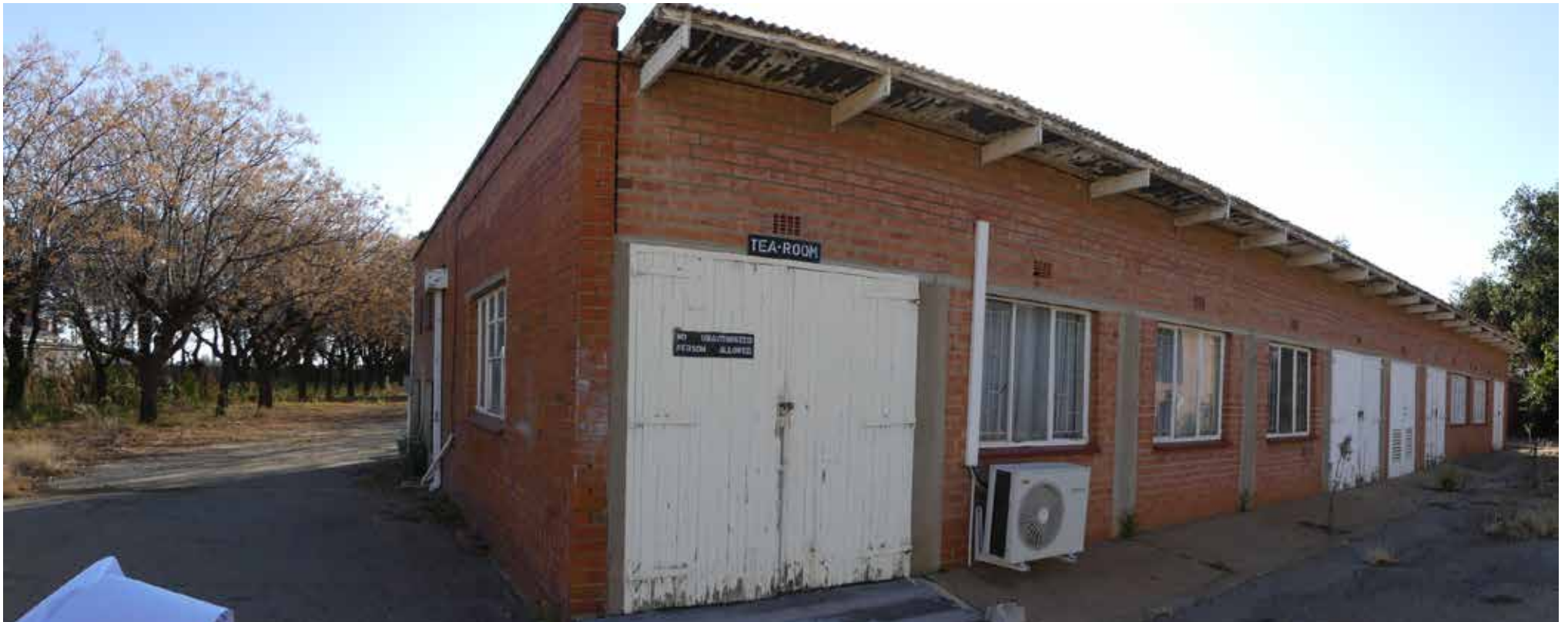
Eastern elevation - building 31.
