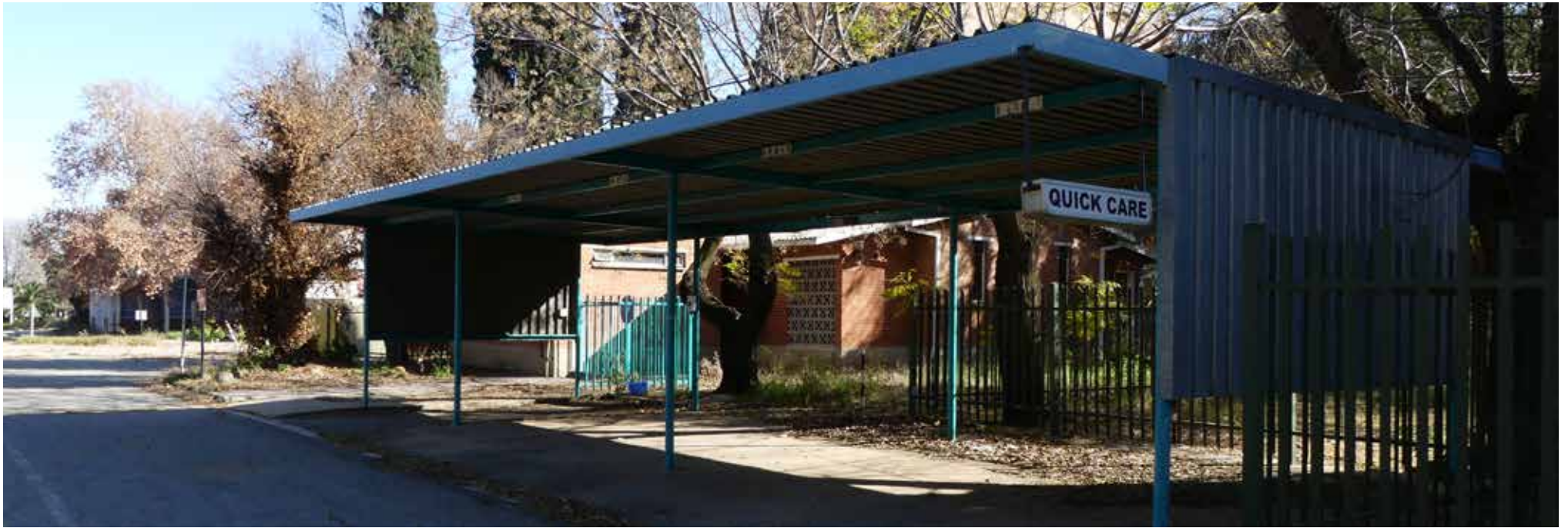
South, Eastern elevation - building 47
