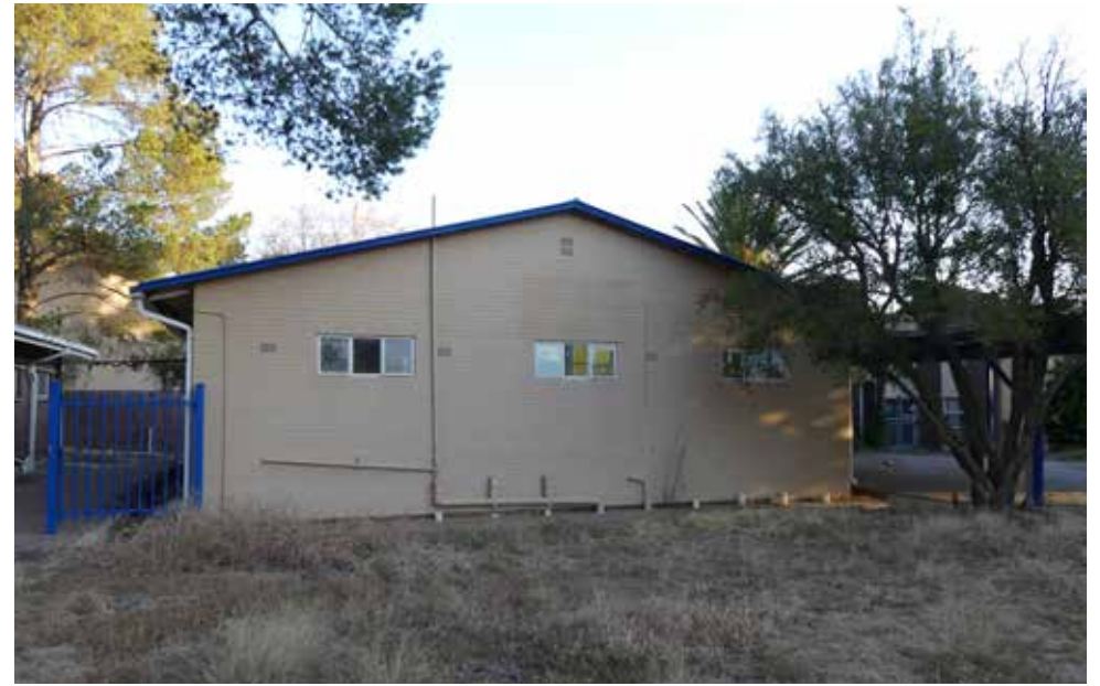
Northern elevation - building 41.
