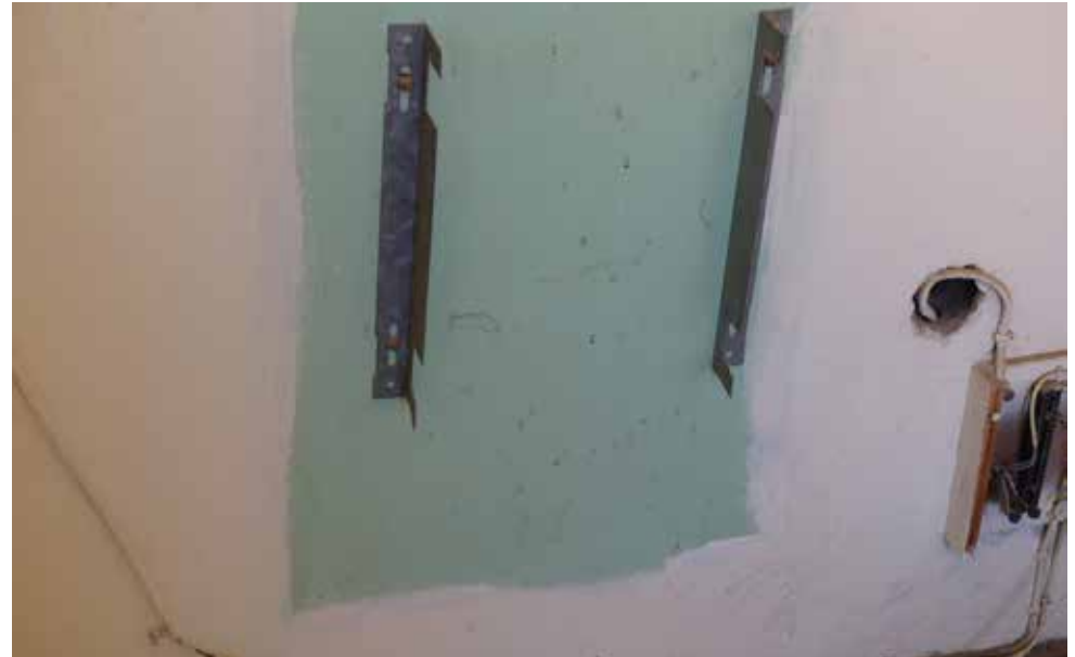
Original wall colour on Third Floor - building 17.
