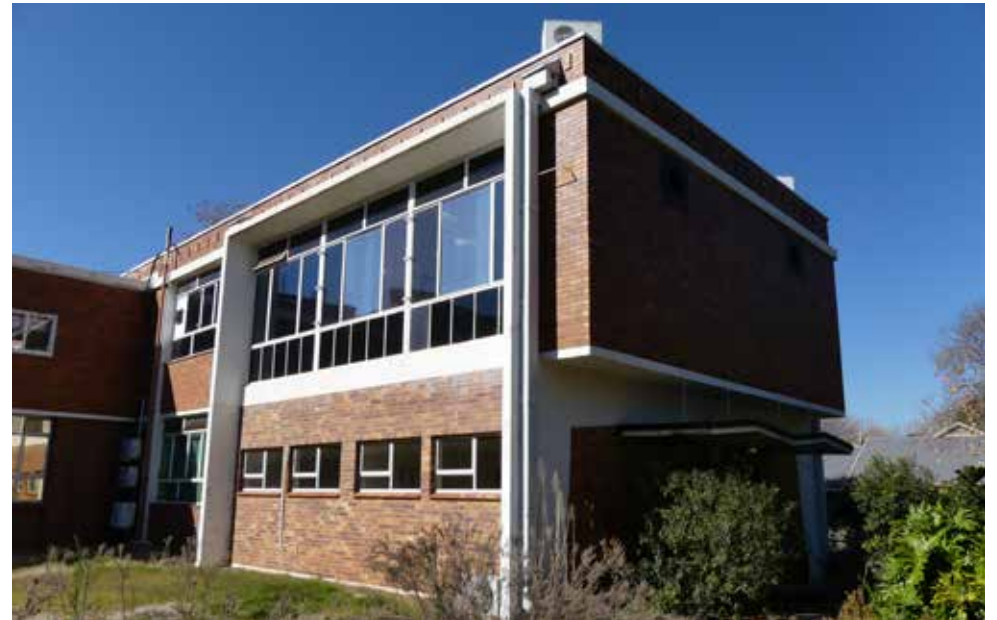
North / Western elevation of Laboratory building - building 23.
