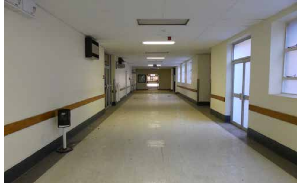
Main Ground Floor corridor (looking west) - building 17.
