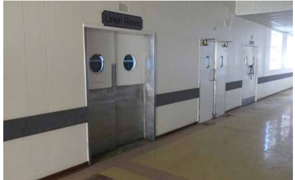
Doors to service area on Third Floor - building 17.
