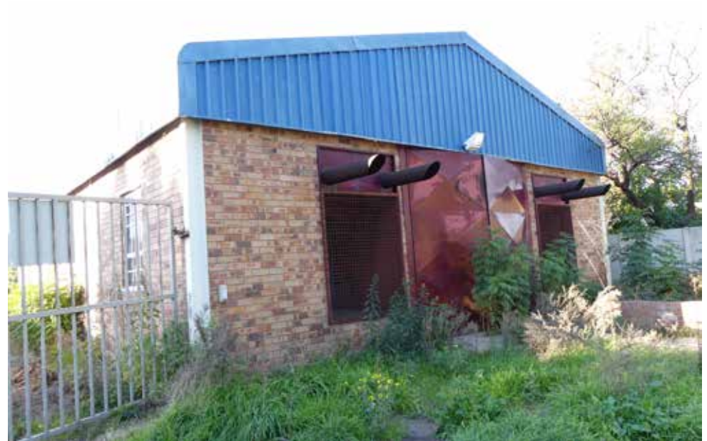
Southern elevation of electrical room - building 34.
