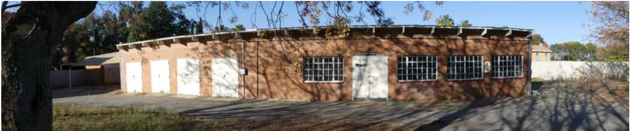
Western elevation - building 31.
