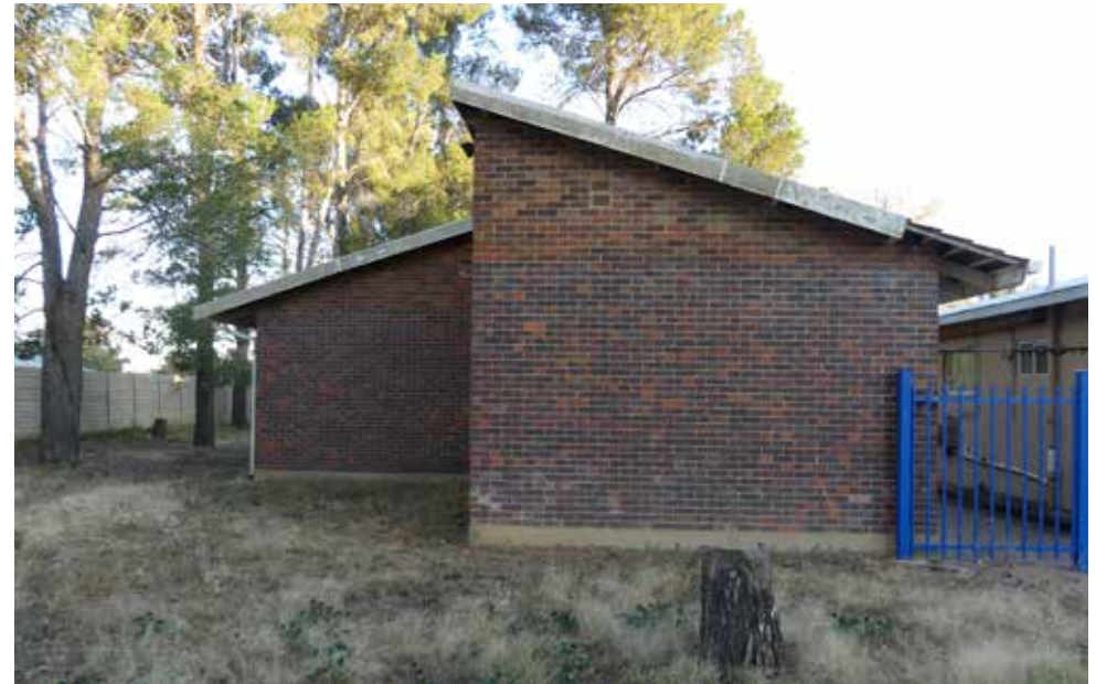
Northern elevation - building 42.
