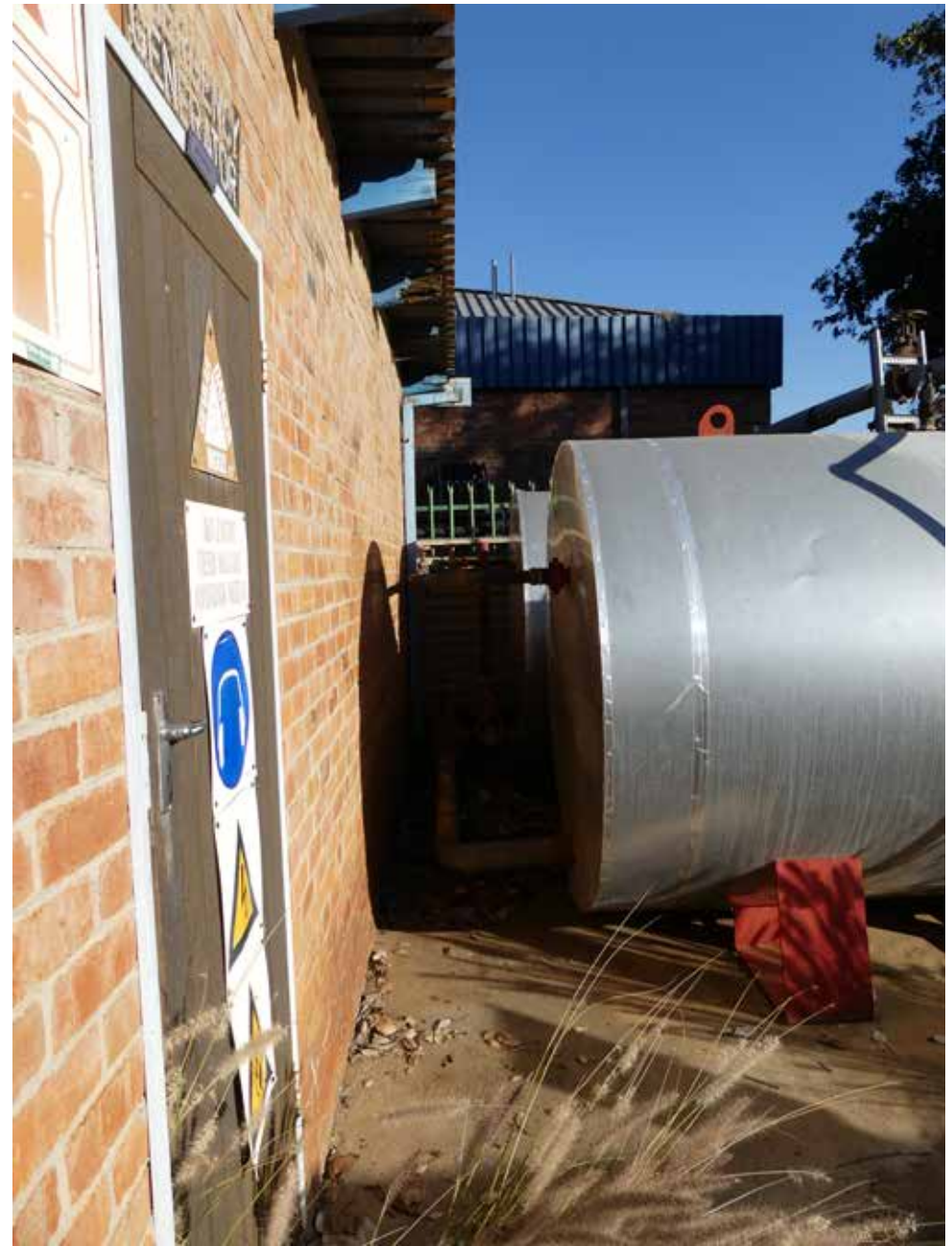
Side of Boiler Room - building 32.
