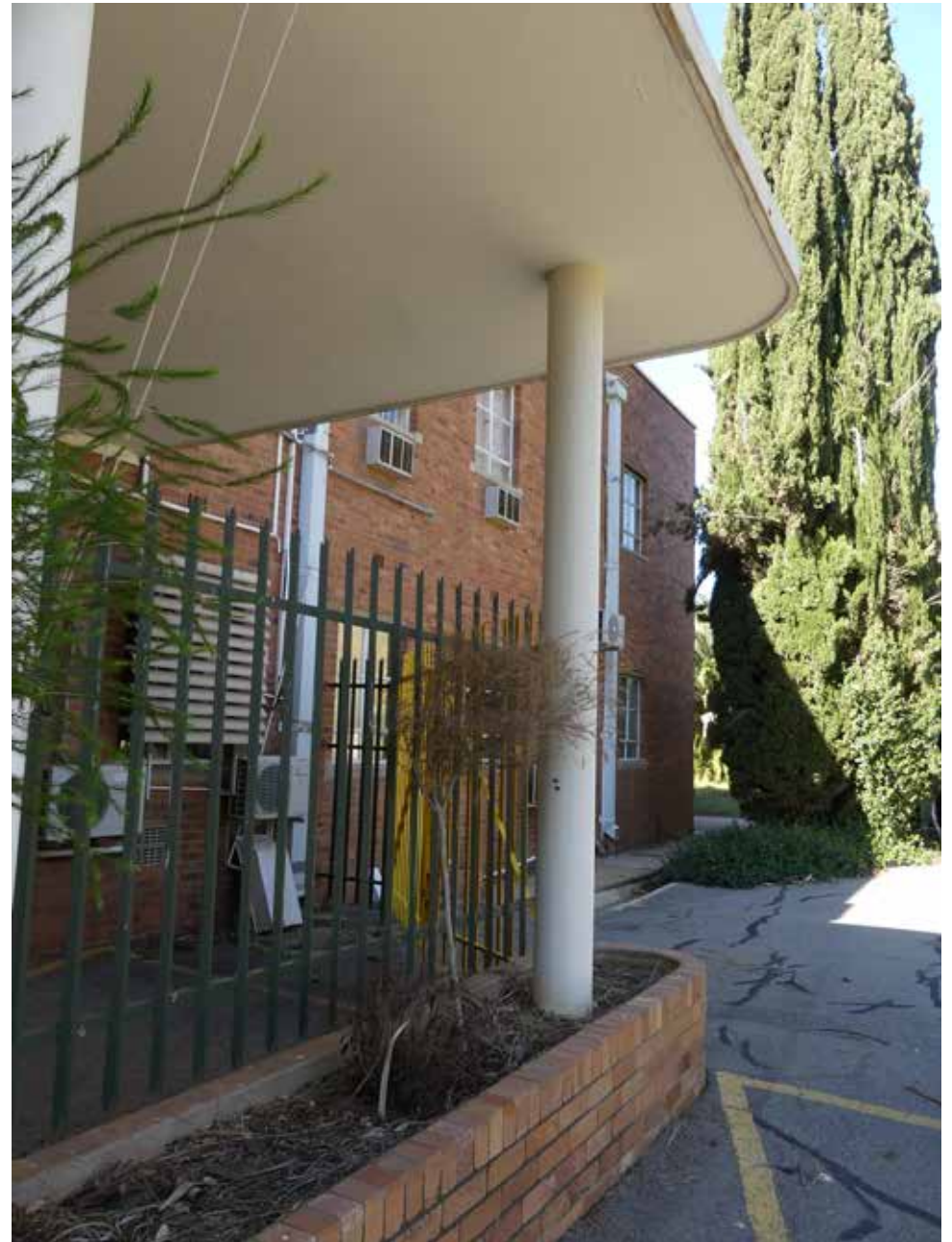
Detail of entrance portico - building 17.
