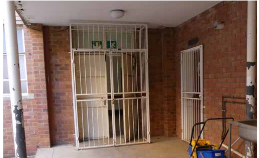
Entrance into Hospital from Laundry courtyard - building 21.
