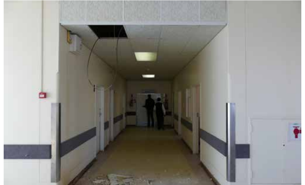
Corridor on Third Floor - building 17.
