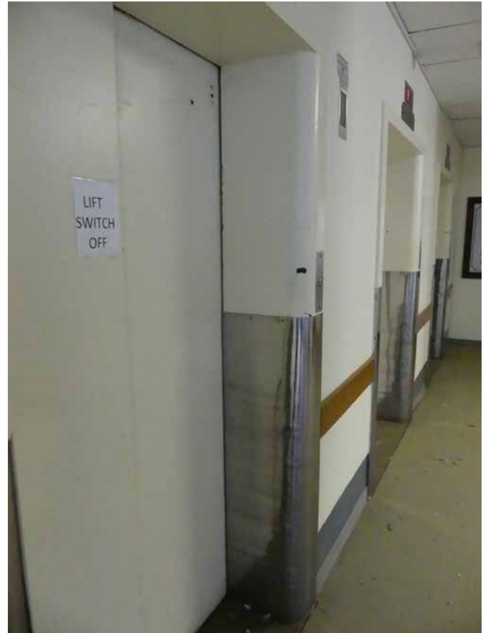
Original lift doors and surrounds - building 17.
