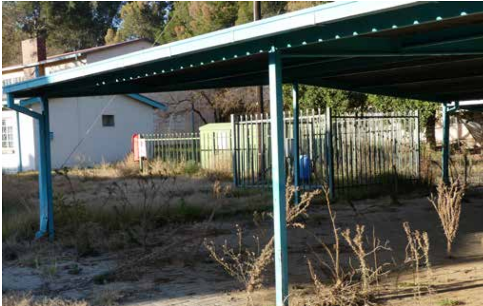
Detail of carports - building 35.
