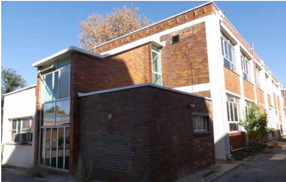
North / Eastern elevation of Laboratory building - building 23.
