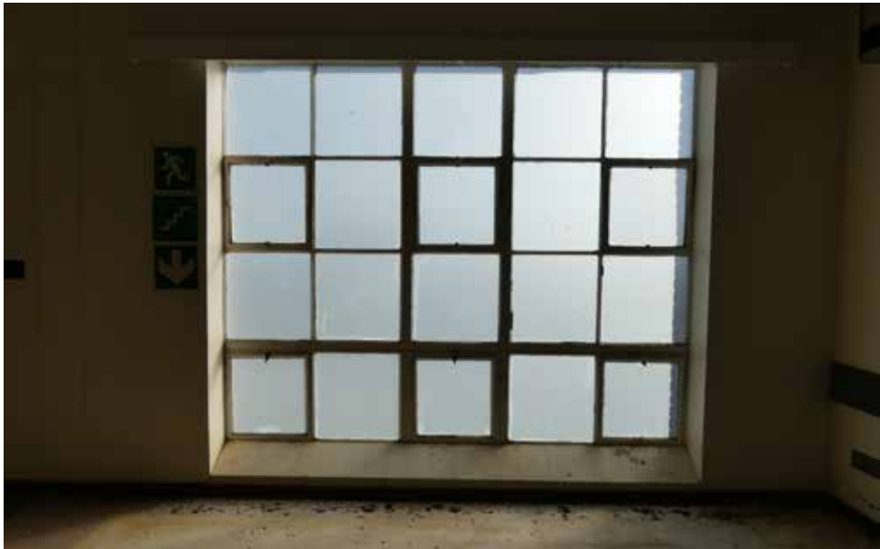
End windows to corridor on Third Floor - building 17.
