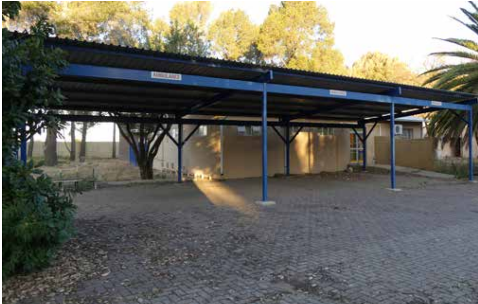
Western elevation - building 43.
