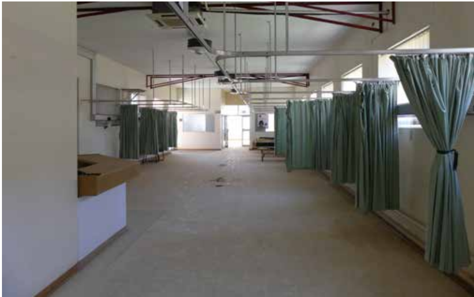
A ward on the Ground Floor - building 17.
