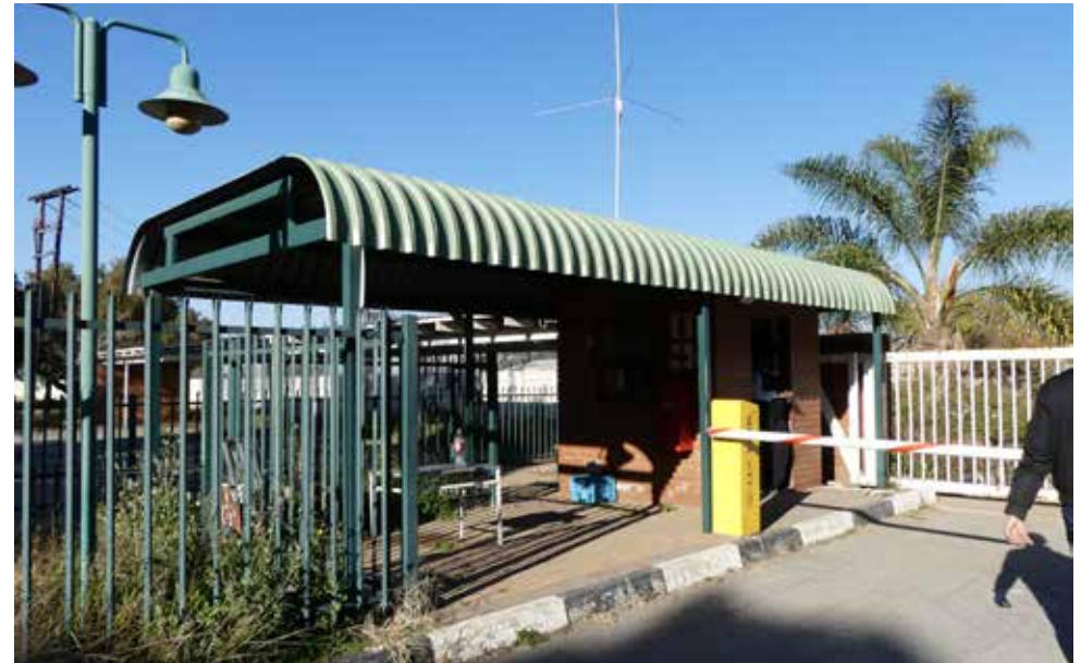
Exterior view of gate house from road - building 15.
