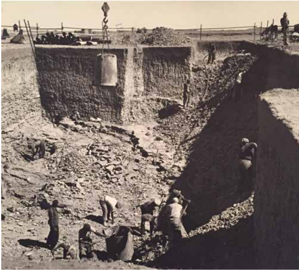
Excavations for a collar, Welkom No.2 (August 18th 1947) - Unknown. (1950).
