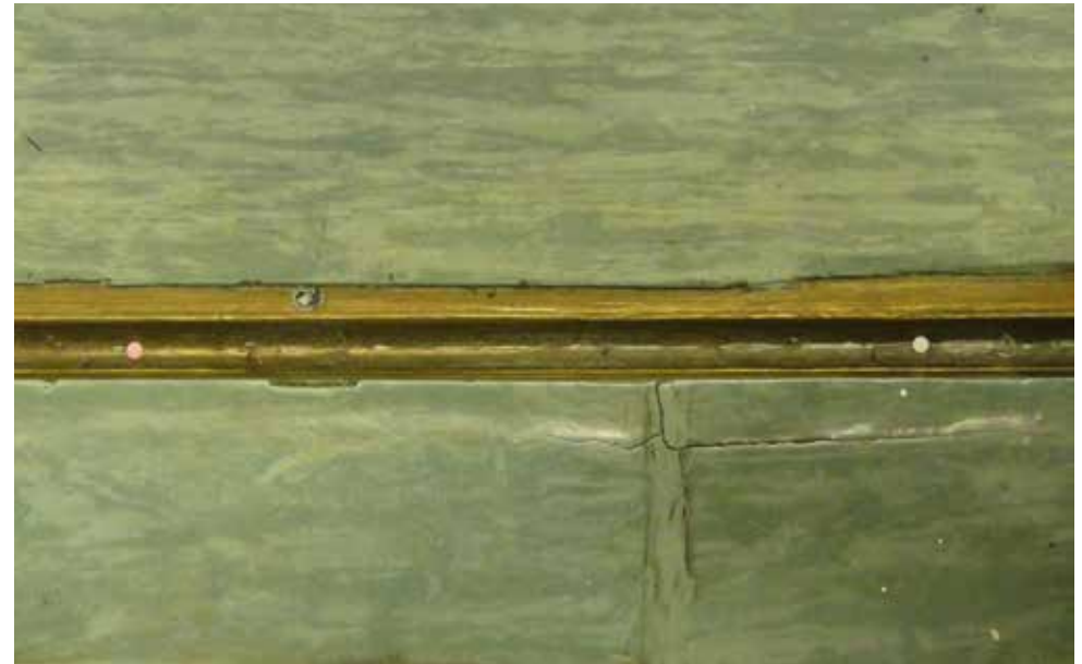
Brass tracks to original theatre doors - building 17.
