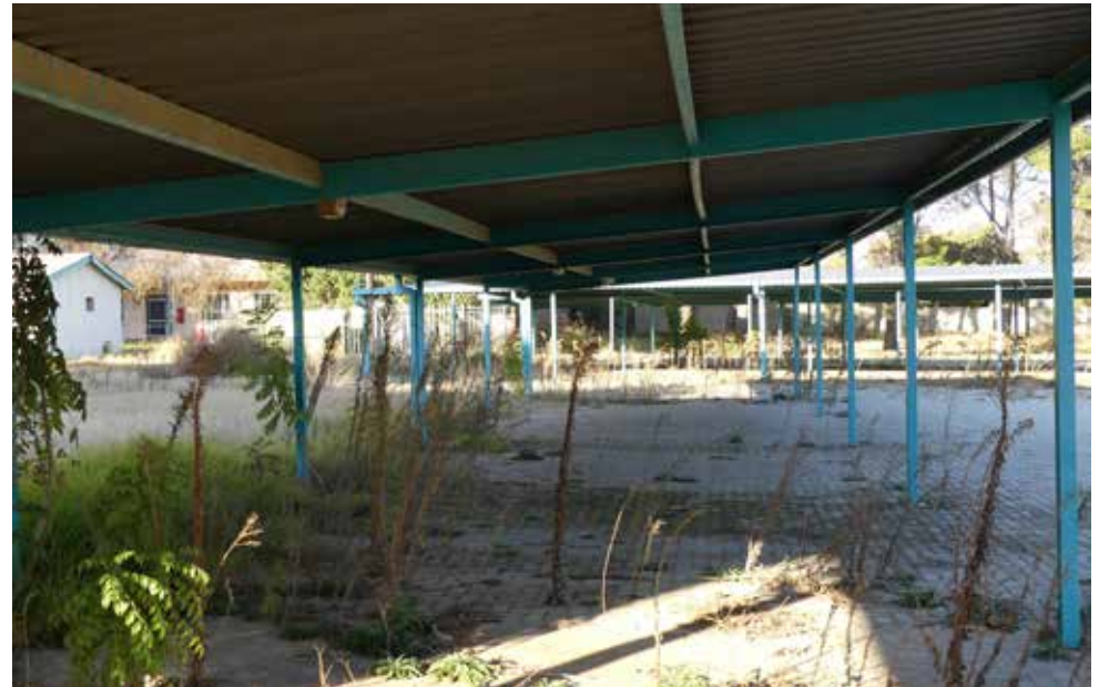
Detail of carports - building 35.
