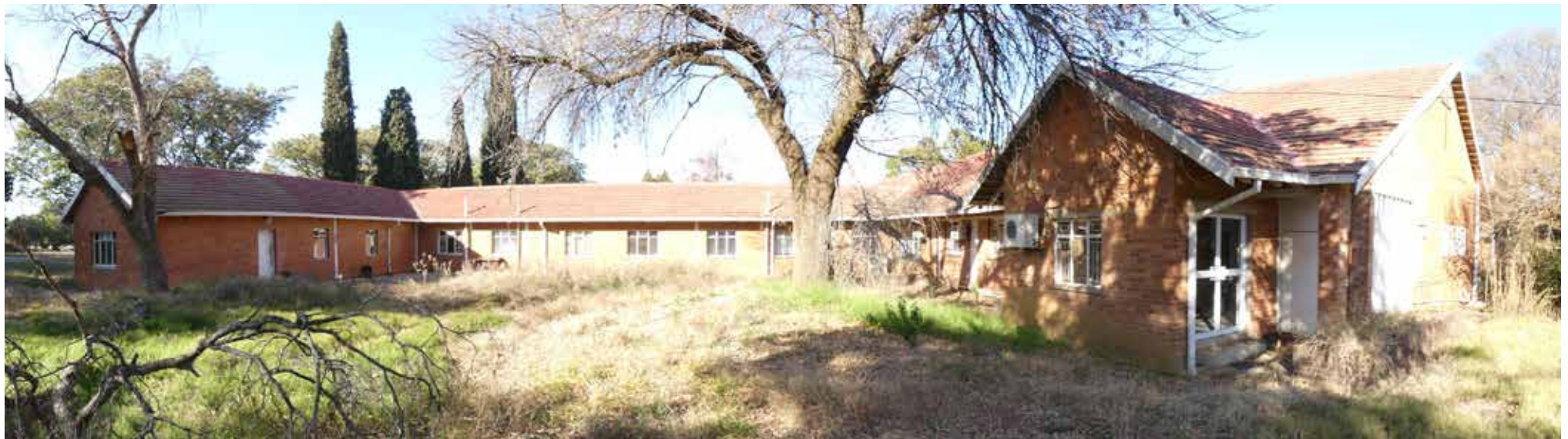
Panoramic view of partial Northern elevation - building 16.
