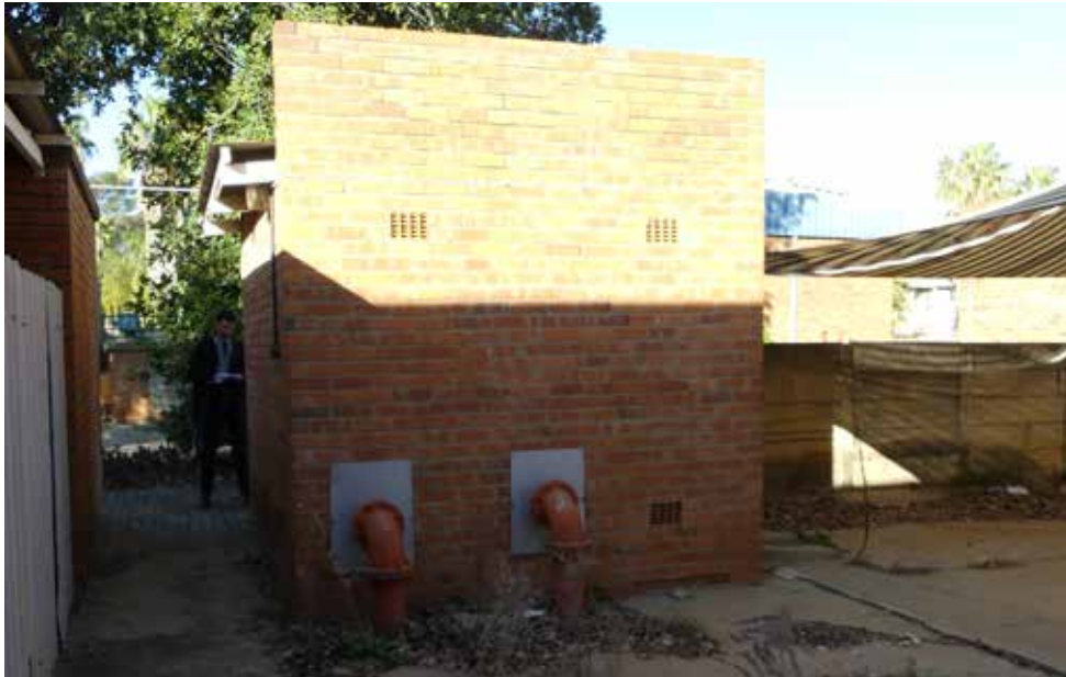
Side of pump house - building 29.
