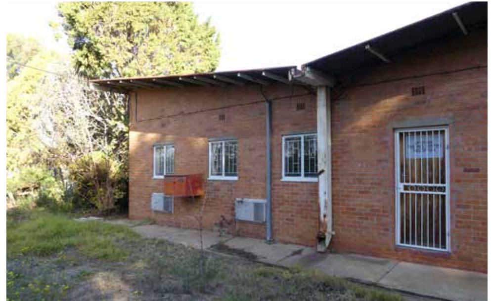
Butterfly roof on section of South elevation of building 13.
