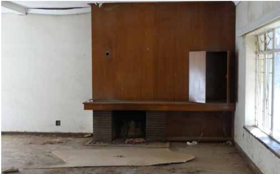
Fire place in lounge of building 7 - Doctor's House Type 6.
