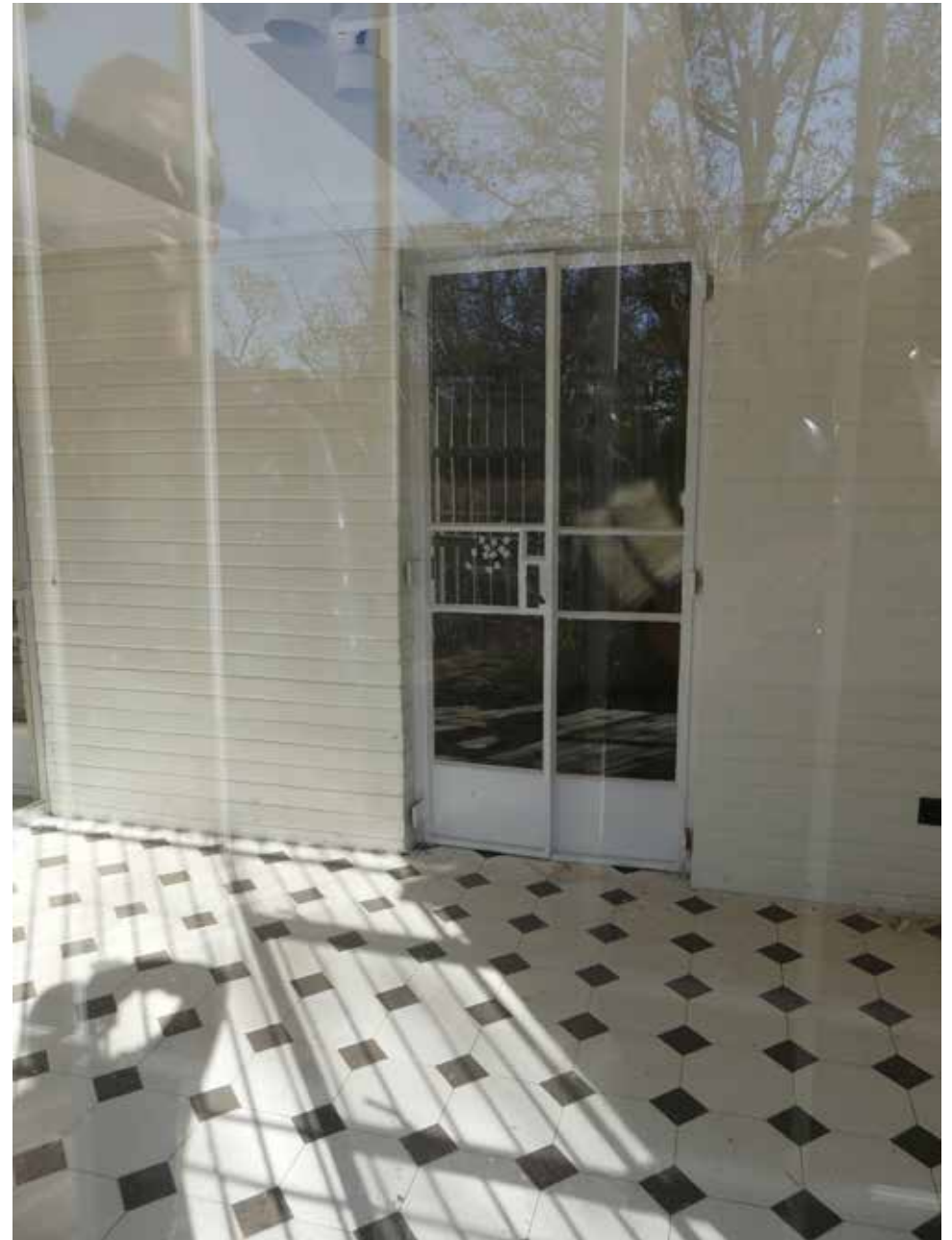
Original door on patio of building 6.
