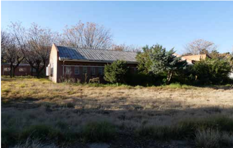
Southern elevation - building 33.
