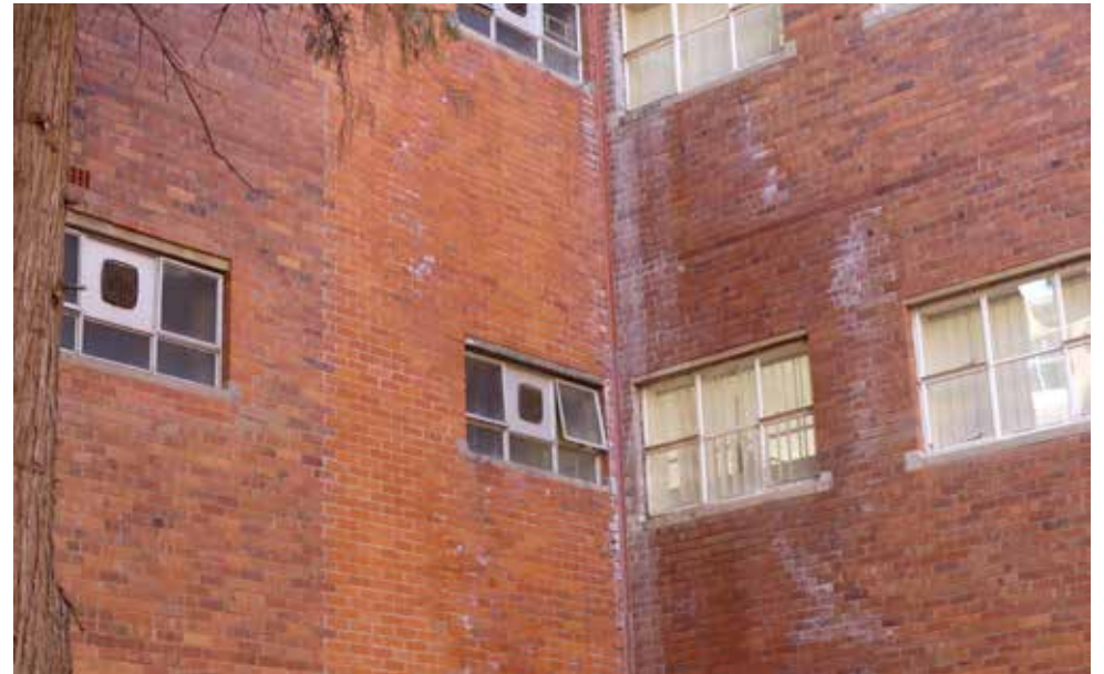
Addition to toilet block - filled in section in different brick - building 17.
