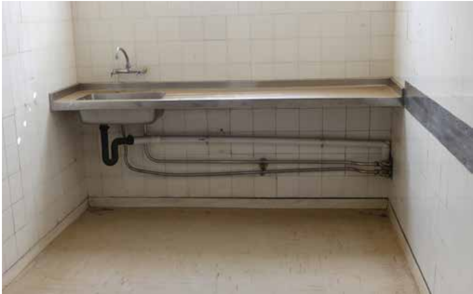
Original sink and pipes on Third Floor - building 17.
