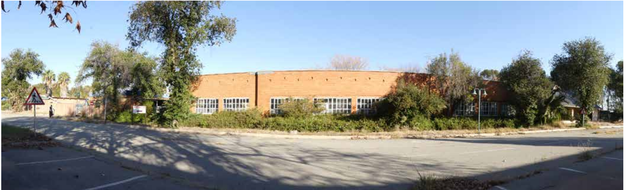
Northern elevation - building 28.
