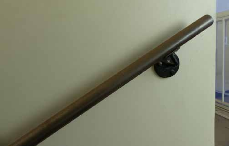
Handrail in staircase of Laboratory building - building 23.
