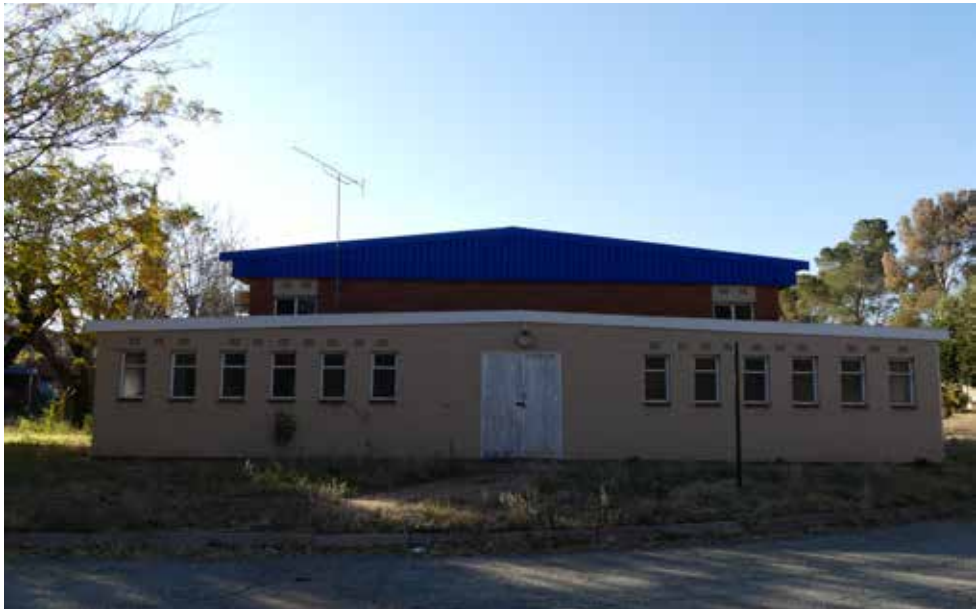
South elevation of building 14.
