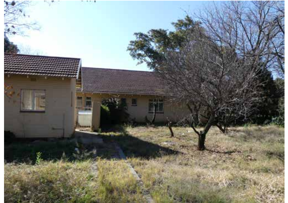
Back elevation of building 3 - Doctor's House Type 6.
