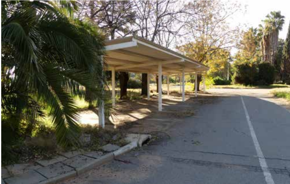
View of carports from the South - building 24.
