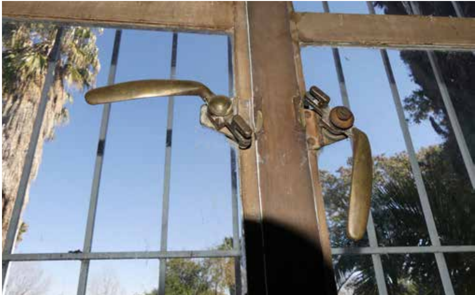
Original window openers of the Boardroom of the Admin Building - building 17.
