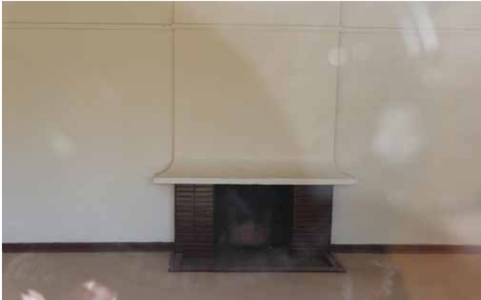
Fire place in lounge of building 4 - Doctor's House Type 5.
