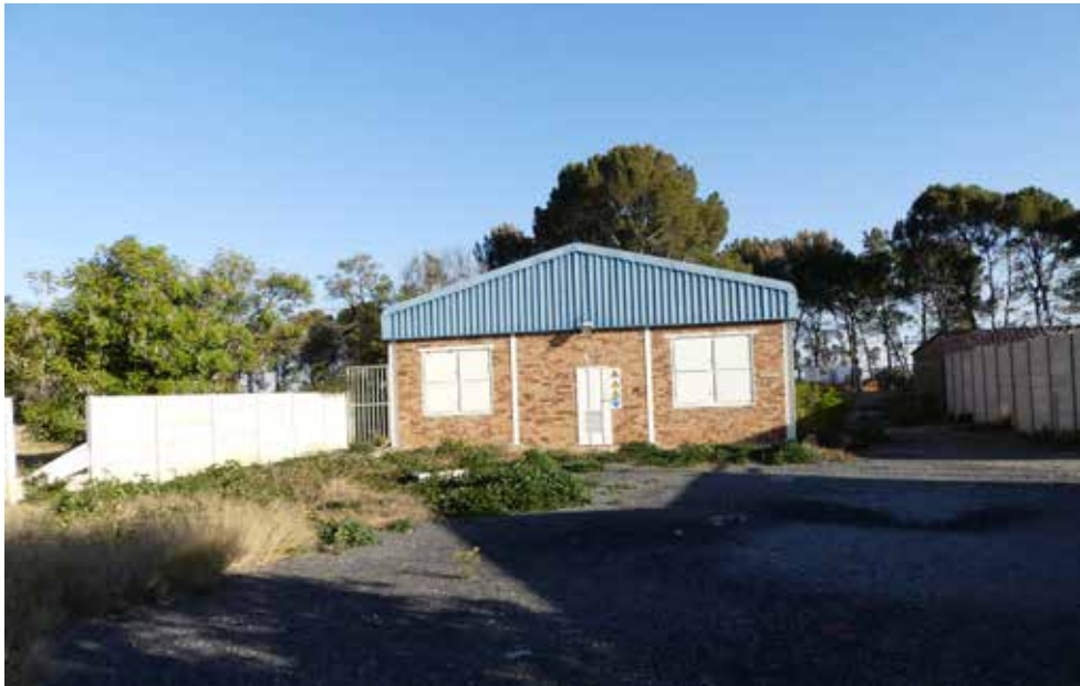
Northern elevation of electrical room - building 34.
