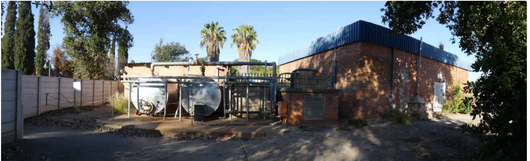
Western elevation - building 32.
