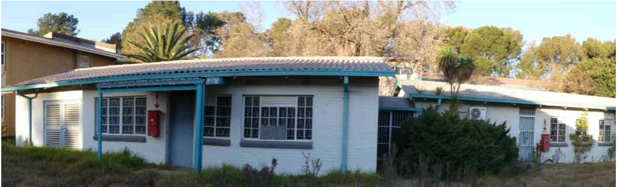
Western elevation - building 39.
