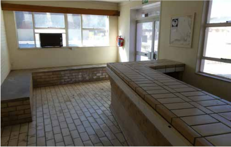
Interior of Laboratory building - building 23.
