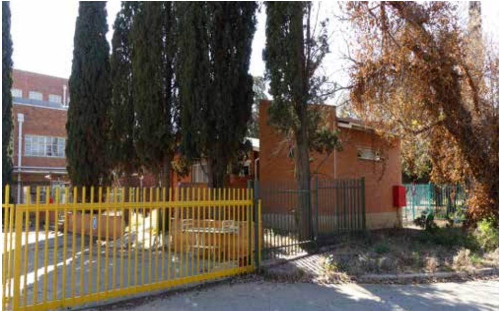
Southern elevation of Mortuary - building 20.
