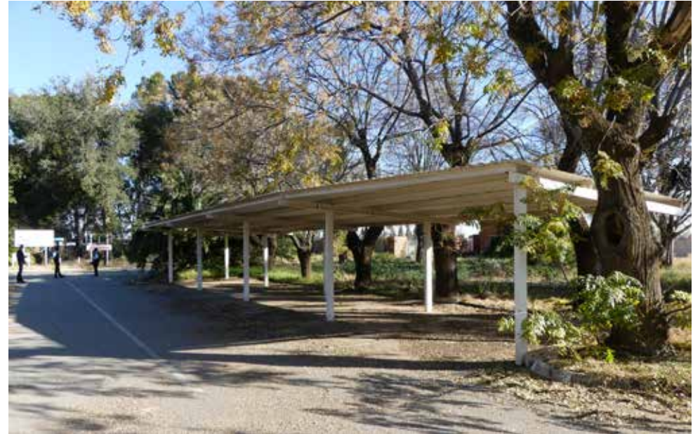
View of carports from the North - building 24.
