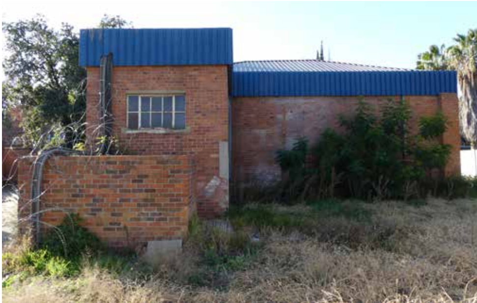
Southern elevation - building 32.
