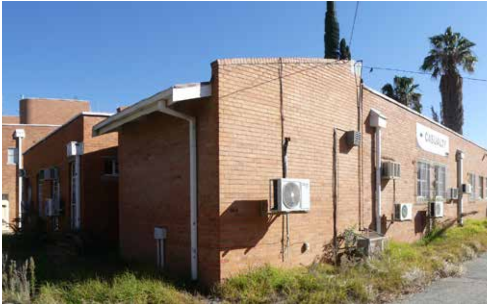
Back elevation of Admin building - building 17.
