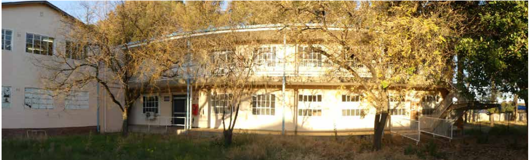
Southern section of Western elevation - building 40.
