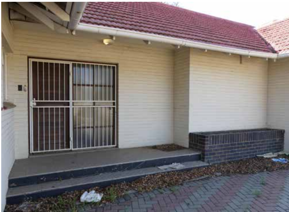
Entrance door of building 5 - Doctor's House Type 7.
