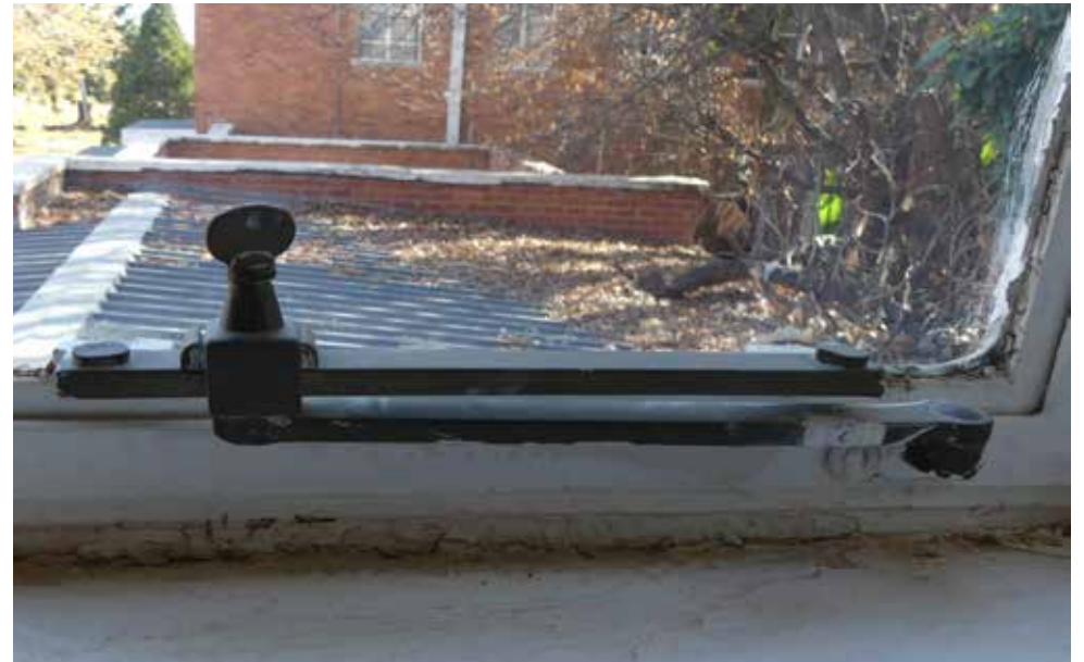
Original window hardware in link between Hospital and Laboratory building - building 17.
