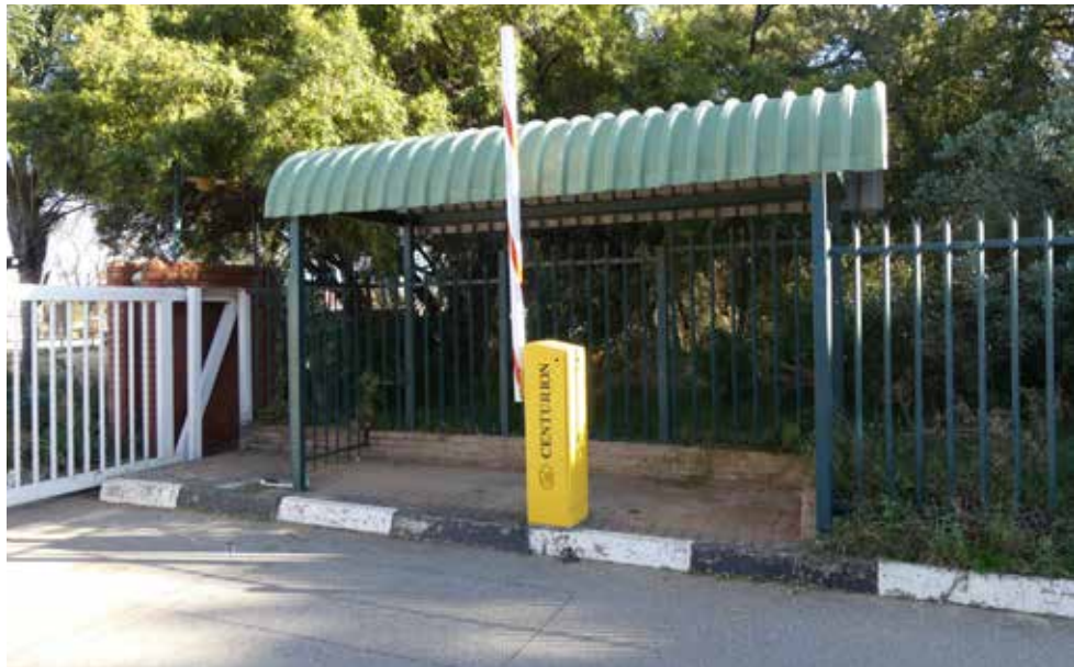
Roof over walkway opposite side of road of gate house - building 15.
