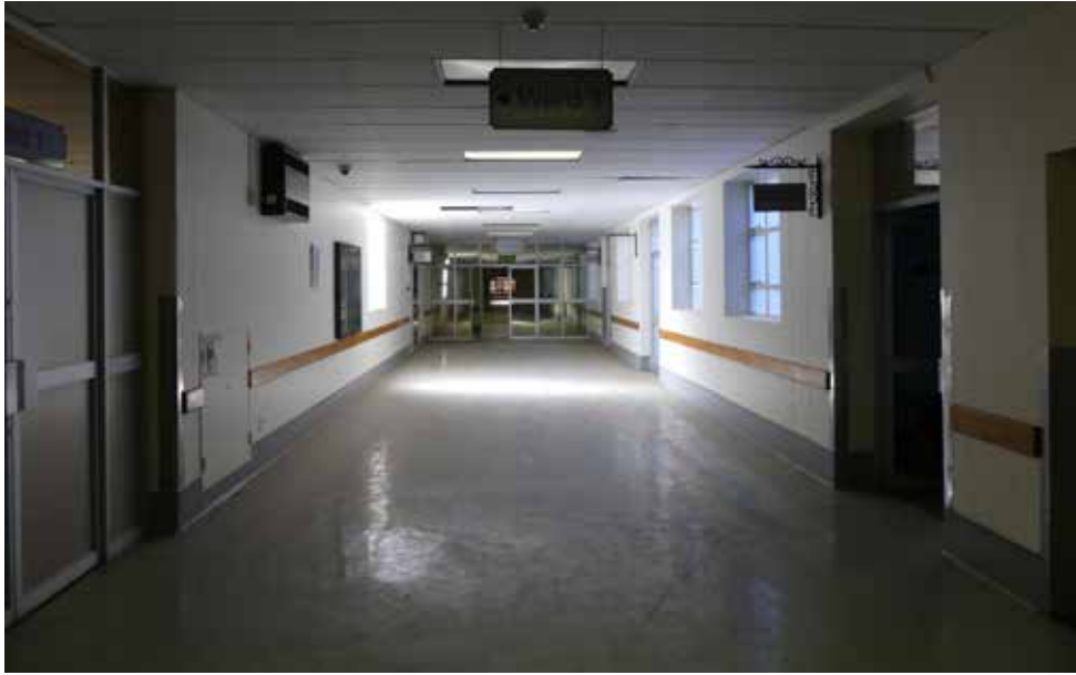
Main Ground Floor corridor (looking east) - building 17.
