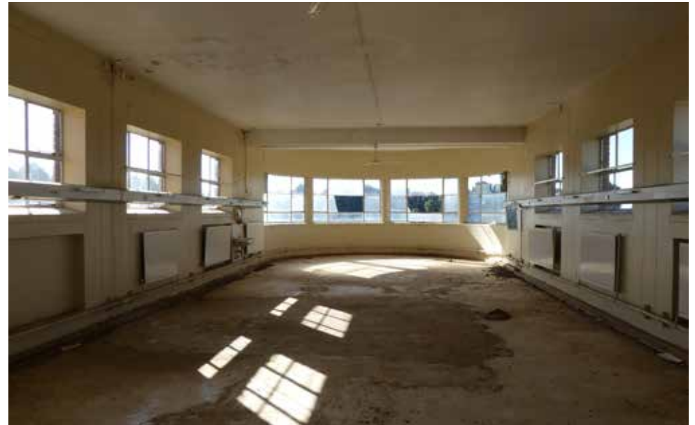
Ward on Third Floor - building 17.
