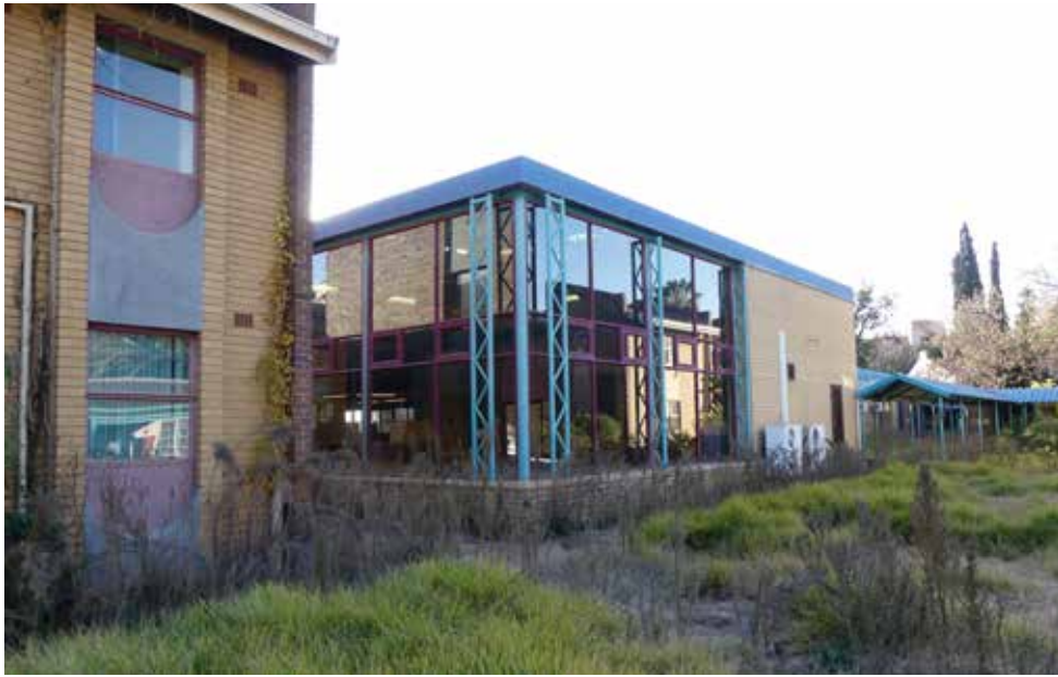
Eastern elevation - building 36 & 37 link.
