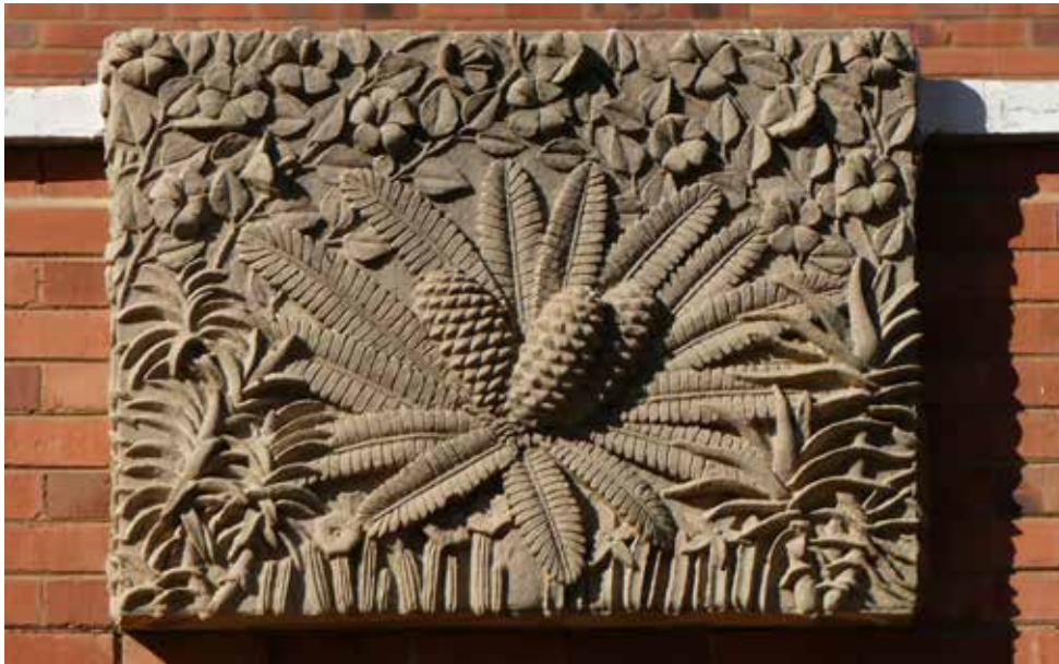
Detail of relief over Administration Block entrance - Cycads - building 17.
