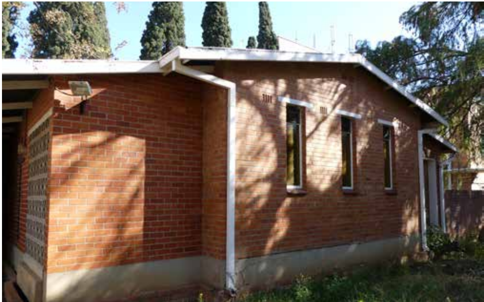
Eastern elevation of Mortuary - building 20.
