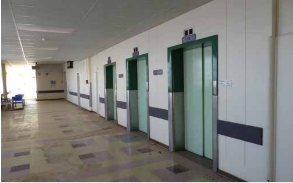
Corridor and Lifts on Third Floor - building 17.
