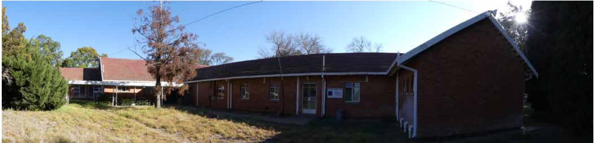
Panoramic view of partial Northern elevation - building 16.
