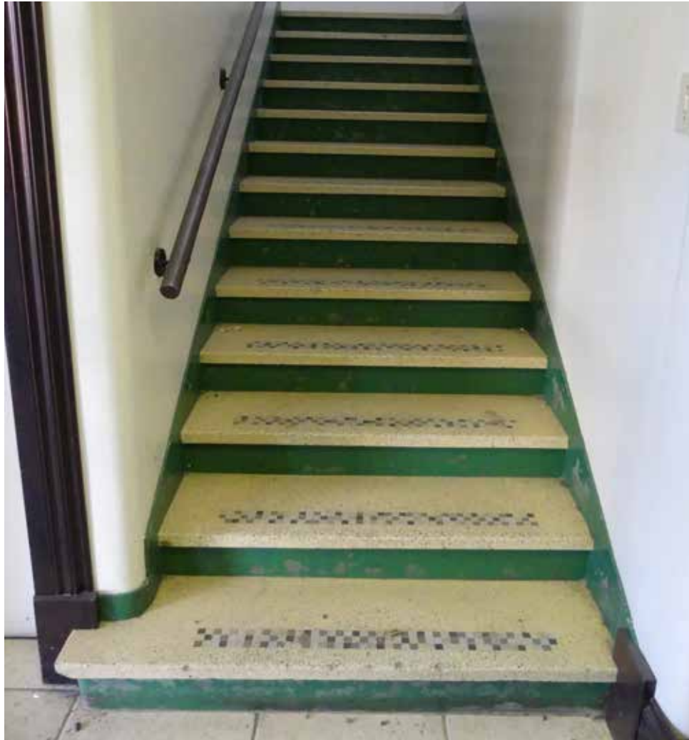
Original terrazzo and mosaic staircase to Admin (East) Block - building 17.
