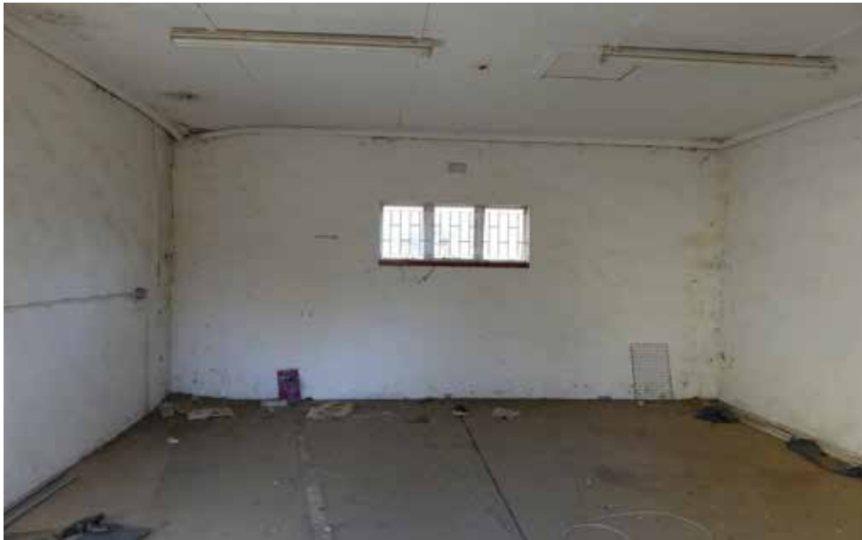
Interior of garage of building 6.
