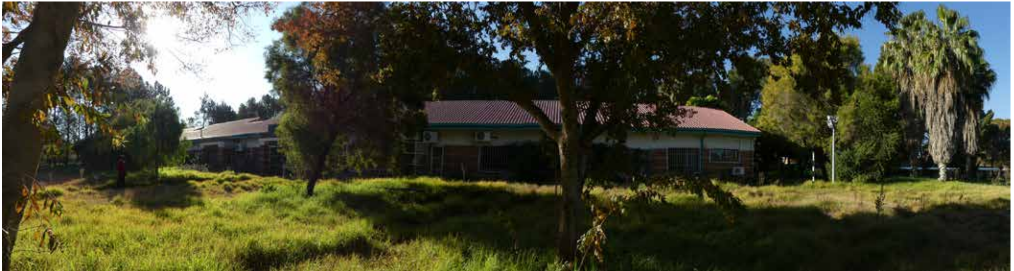
Panoramic view of Southern elevation of building 12.
