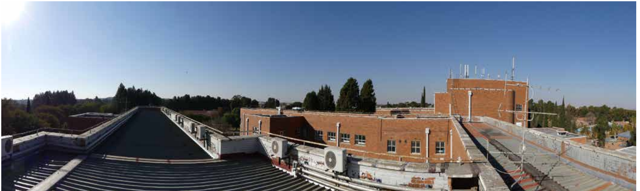
Contemporary corrugated roof sheeting placed over original flat roof - building 17.
