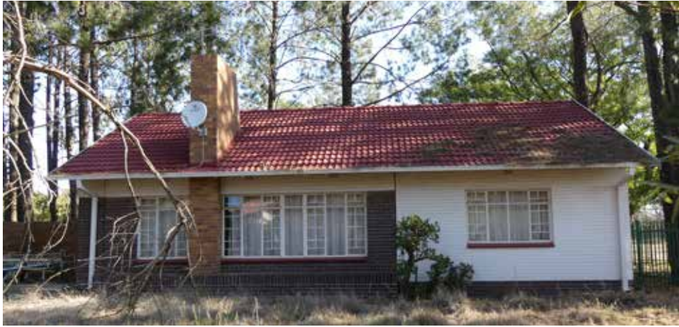
Back view of building 9.
