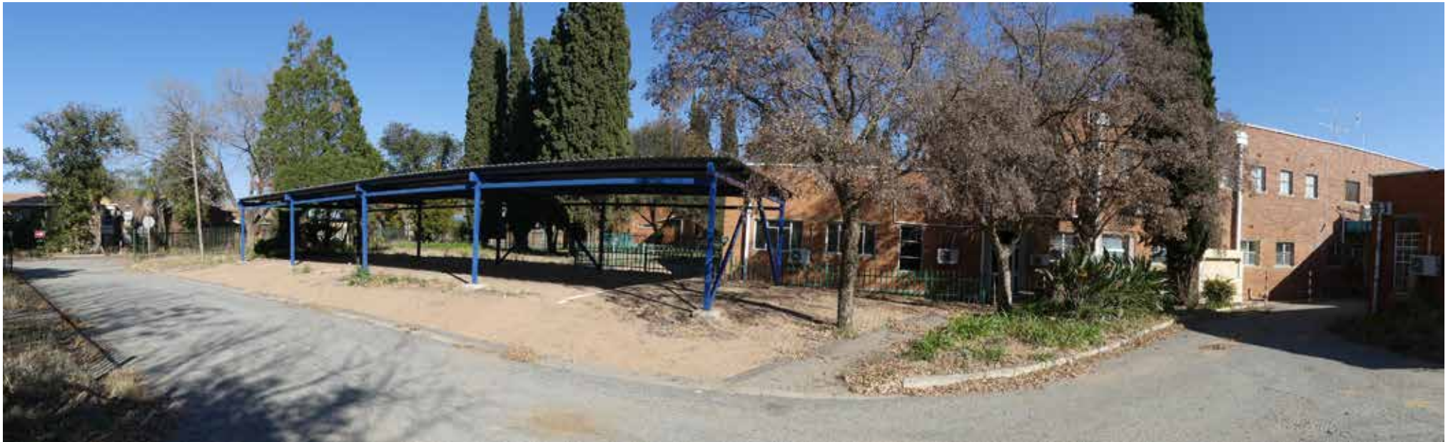
Eastern elevation - building 46.
