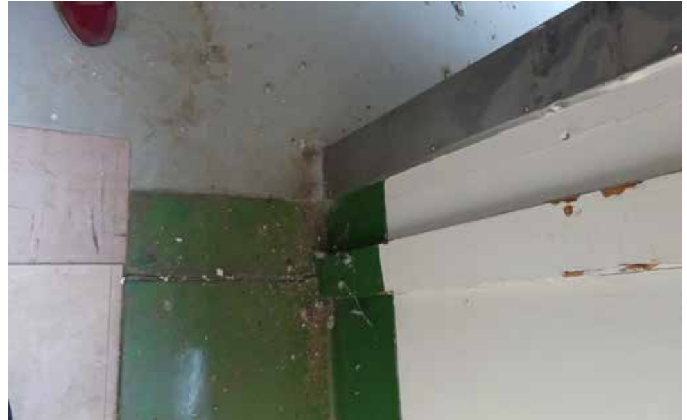
Detail of skirting on Second Floor - building 17.
