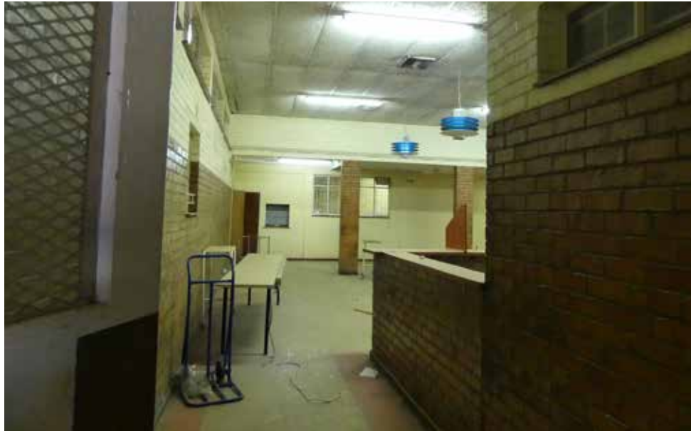
Interior of building 13.
