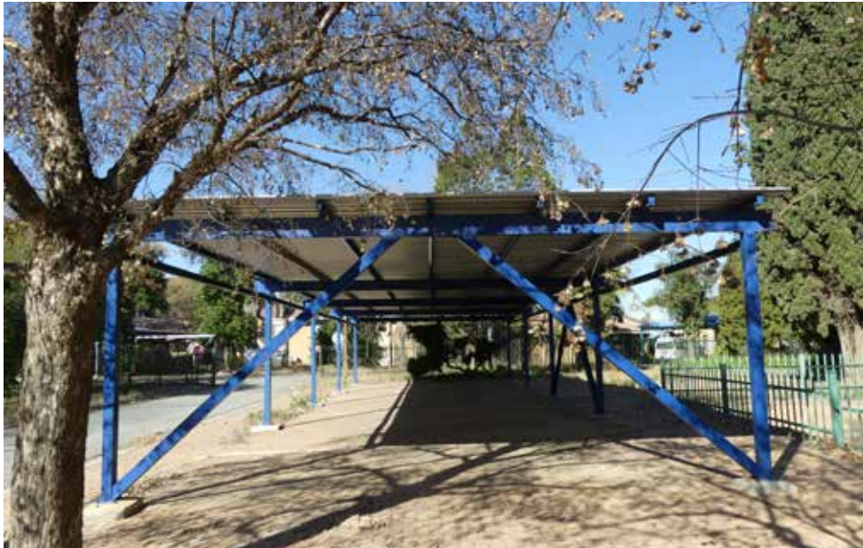
Northern elevation - building 46.
