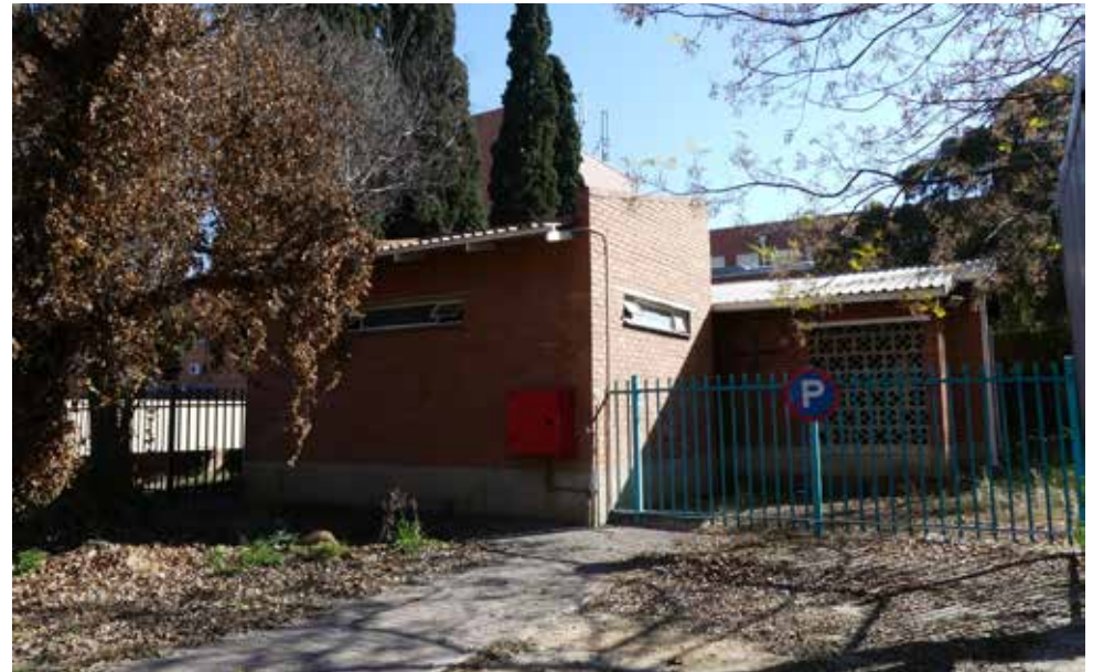
Southern elevation of Mortuary - building 20.
