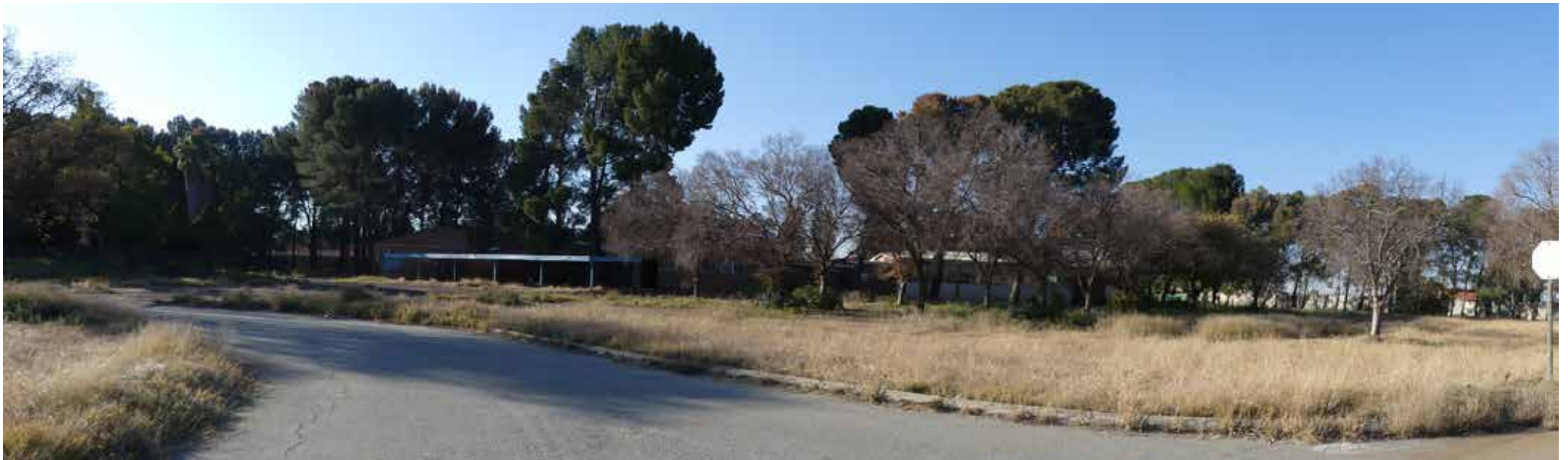
Back (South) elevation of building 13.
