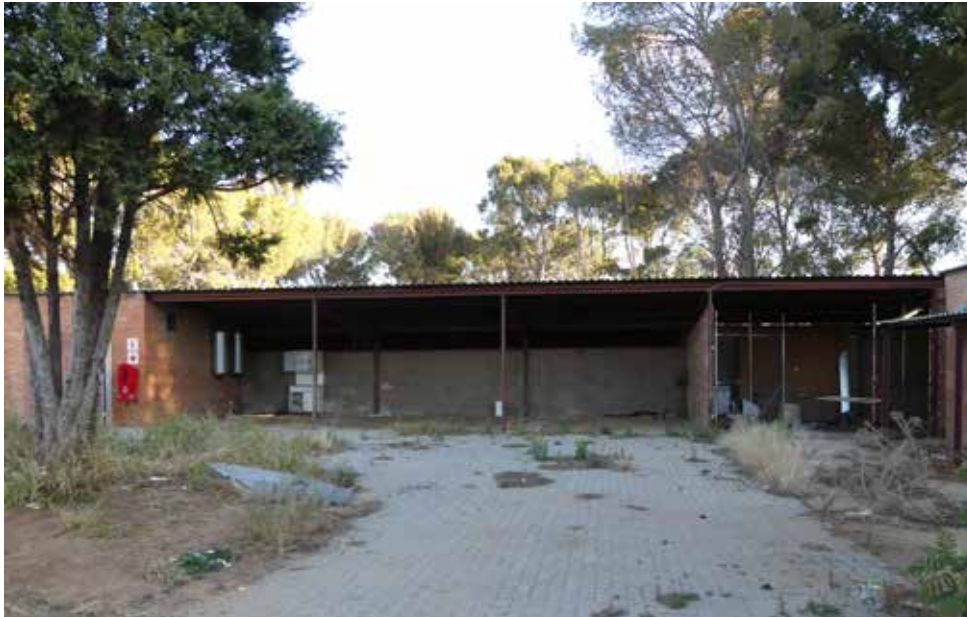
Storage area in the Nursery - building 34.
