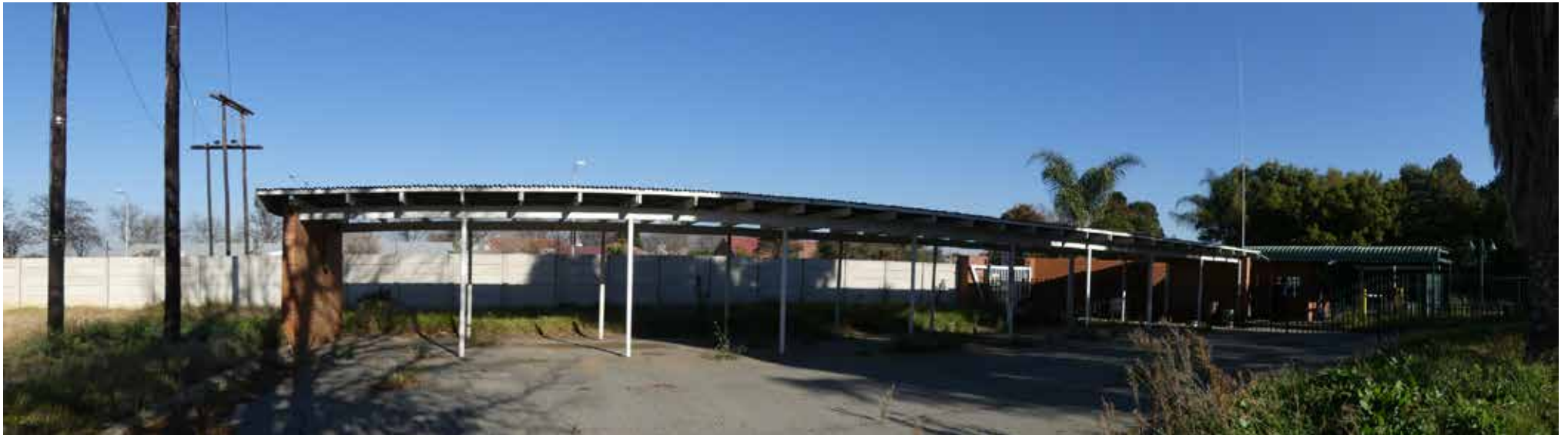
Panoramic view of carport - building 15.
