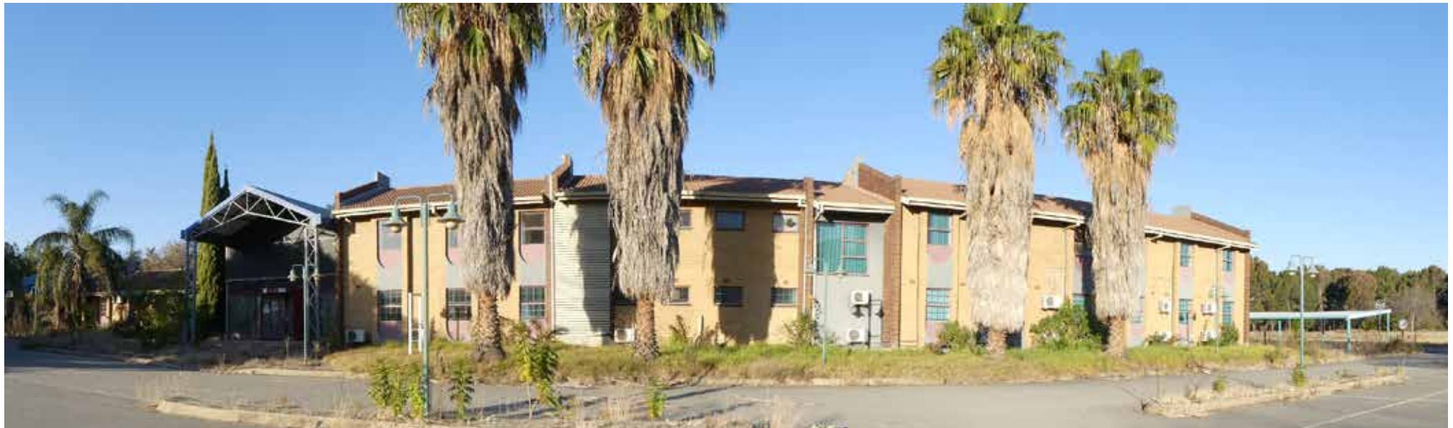
Western elevation - building 36.
