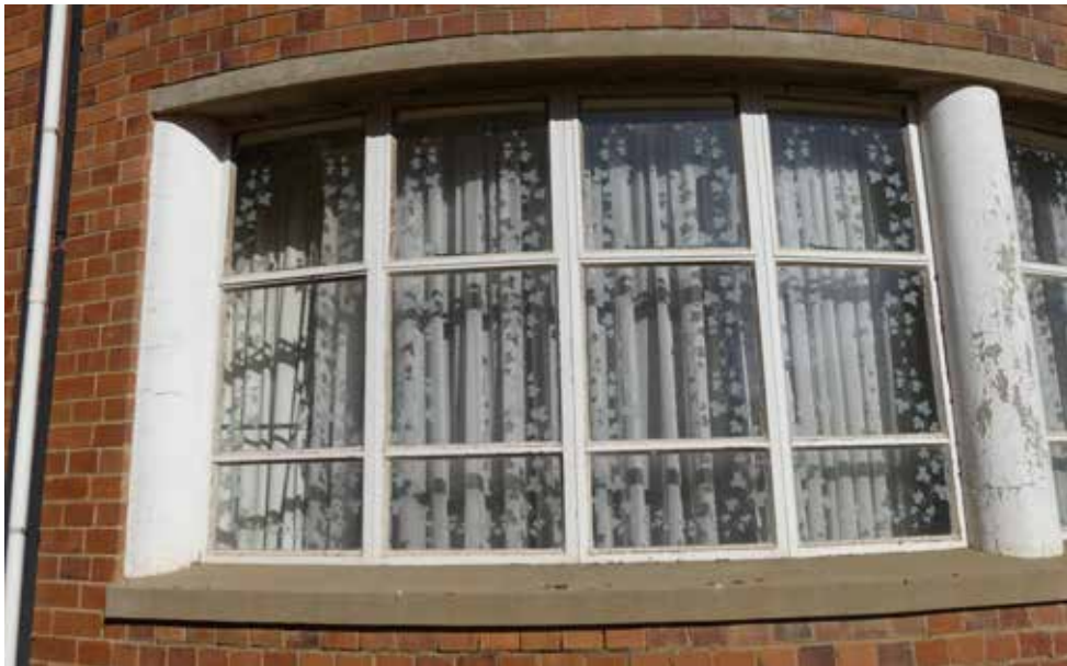
Curved windows of 1952 (original) wards - building 17.
