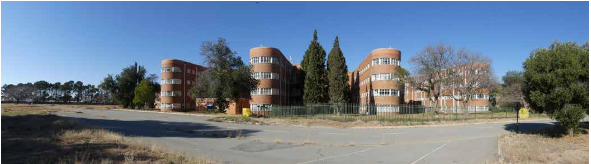
Panoramic view of Northern elevation of building 17 - Main hospital wards.
