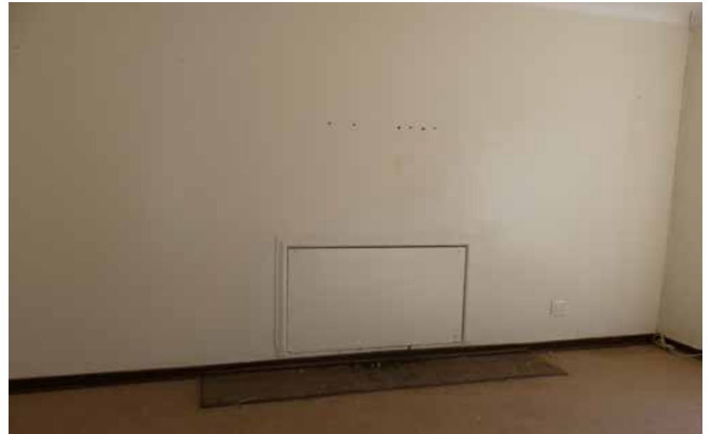
Modified fire place in building 5 - Doctor's House Type 7.
