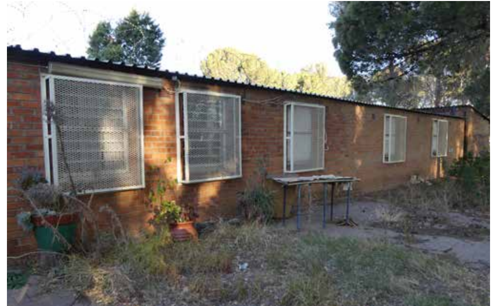
Eastern elevation of Nursery - building 34.
