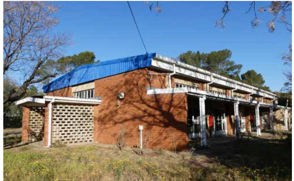
North, Western elevation of building 14.
