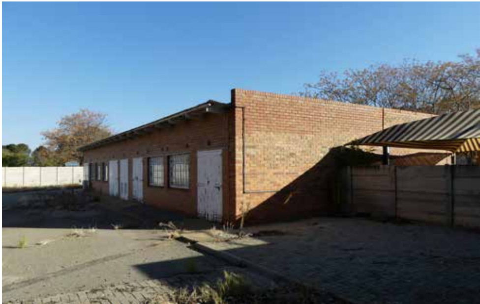
Northern elevation - building 31.
