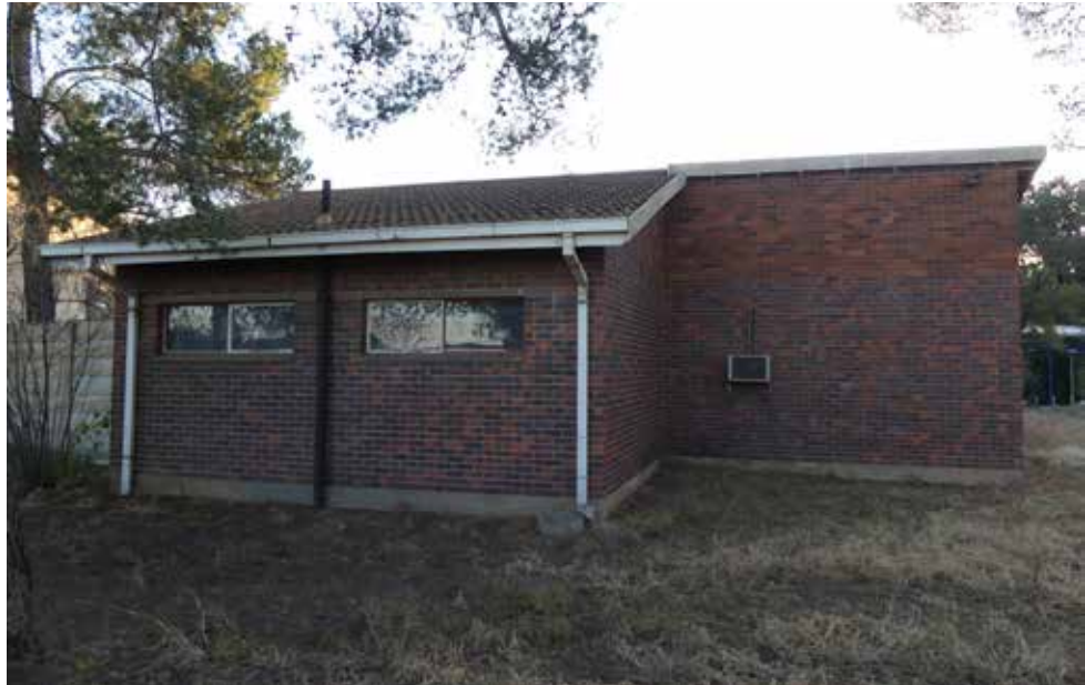
Eastern elevation - building 42.
