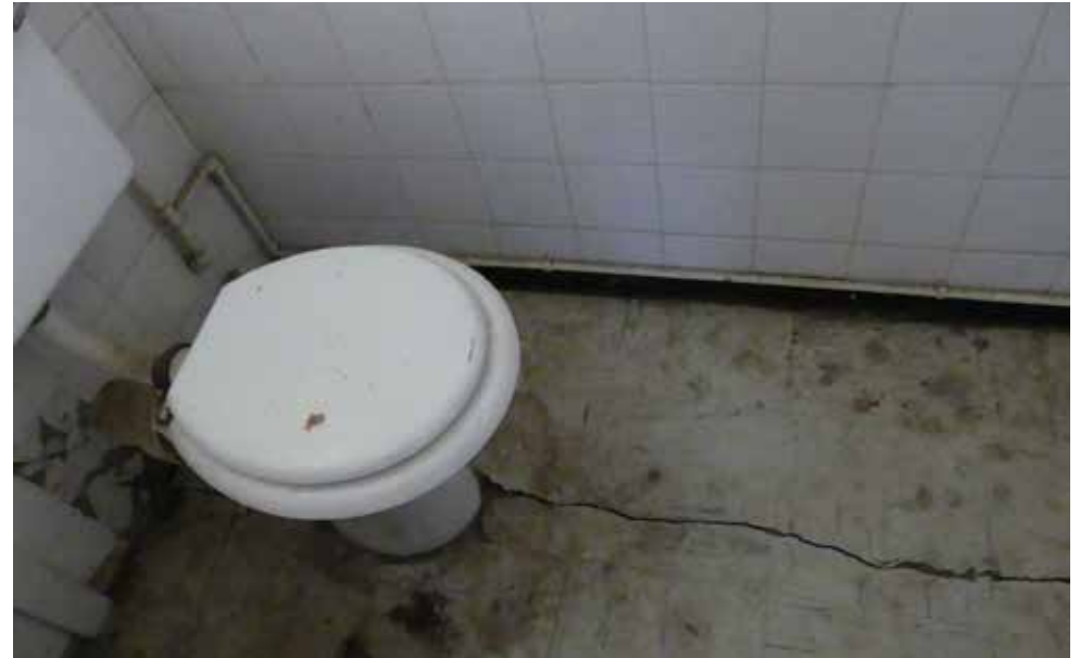
Toilet in building 1 - Doctor's House Type 7.
