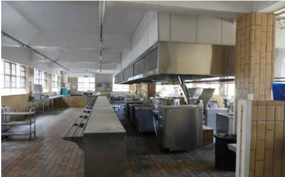
Interior of Kitchen - building 21.
