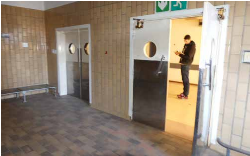
Doors to service area - building 17.
