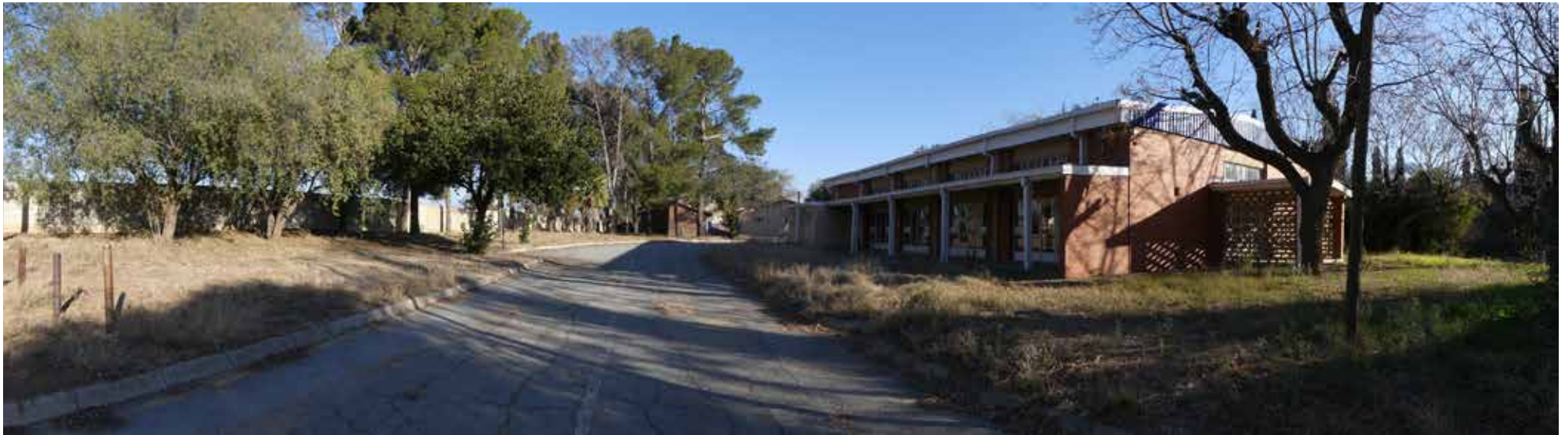
Panoramic view of Eastern elevation of building 14.
