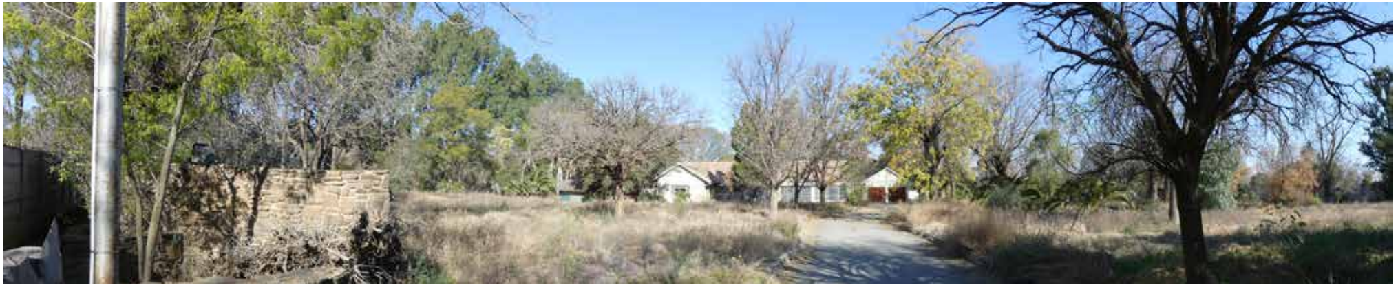
Panoramic view of building 6.
