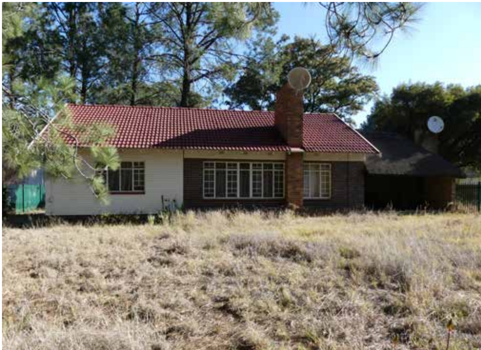
Back elevation of building 8.
