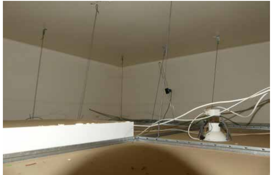
Original ceiling of the Boardroom of the Admin Building - building 17.
