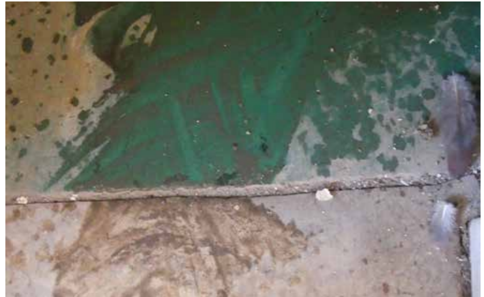
Original Linoleum and green floor paint on Third Floor - building 17.
