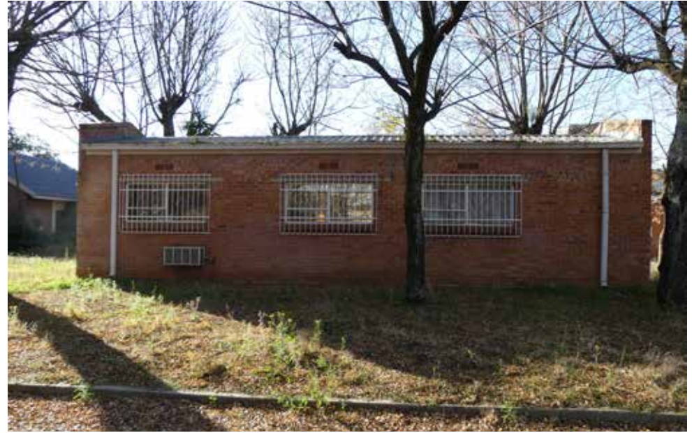
Southern elevation - building 30.
