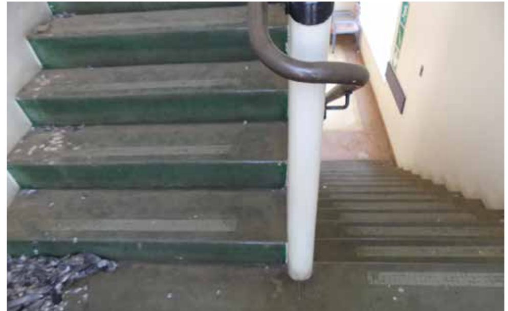
Original staircase with terrazzo and mosaics - building 17.
