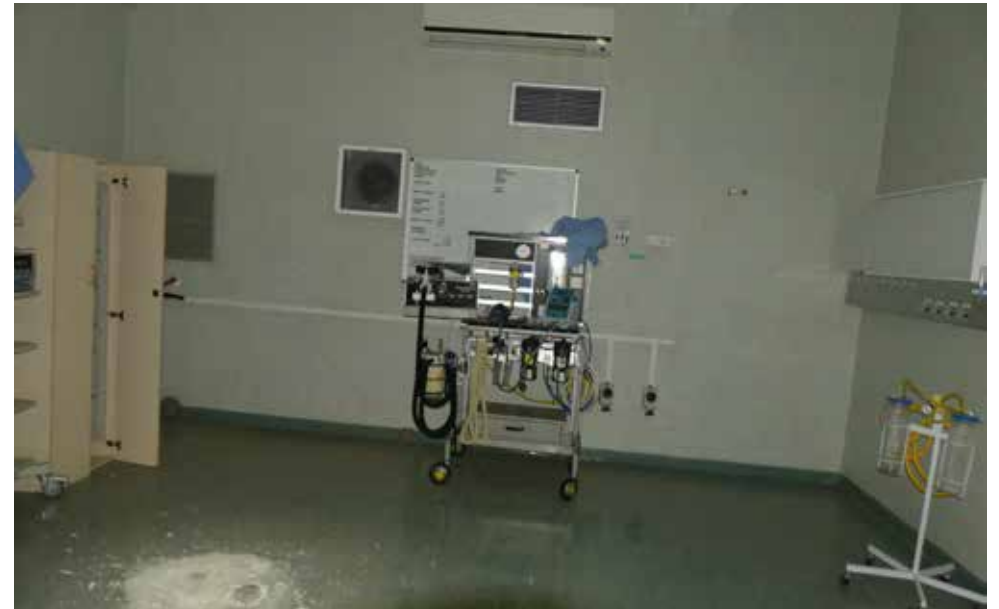
Theatres on First Floor - building 17.
