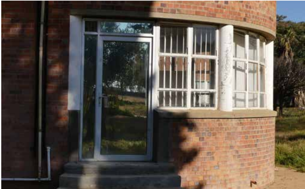
Modifications to the front of a ward - building 17.
