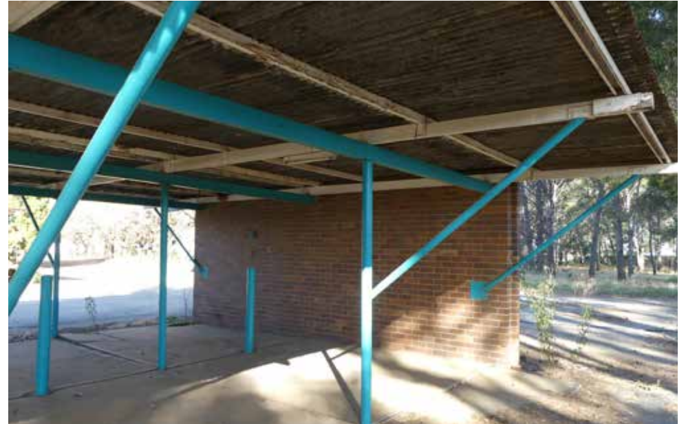
Detail of carport structure - building 25.
