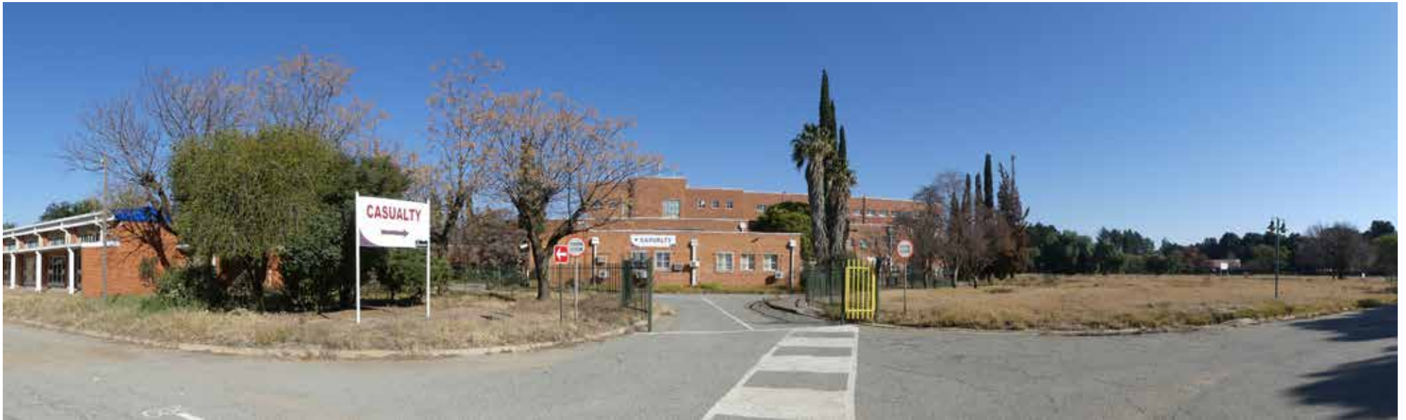
Western elevation of Admin building - building 18.
