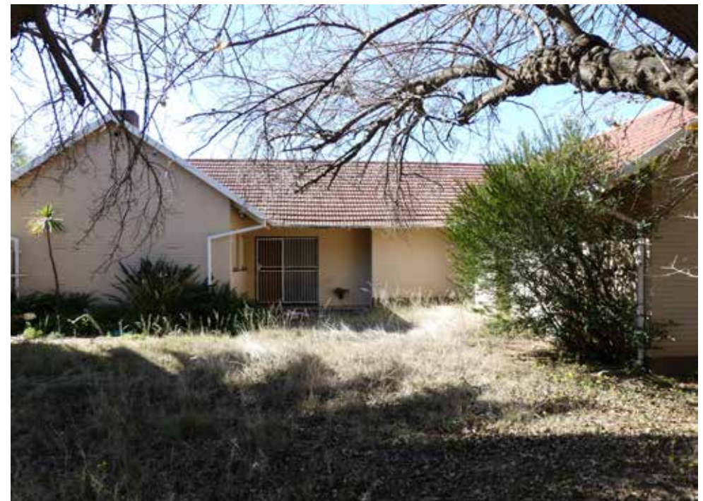
Entrance door of building 1 - Doctor's House Type 7.
