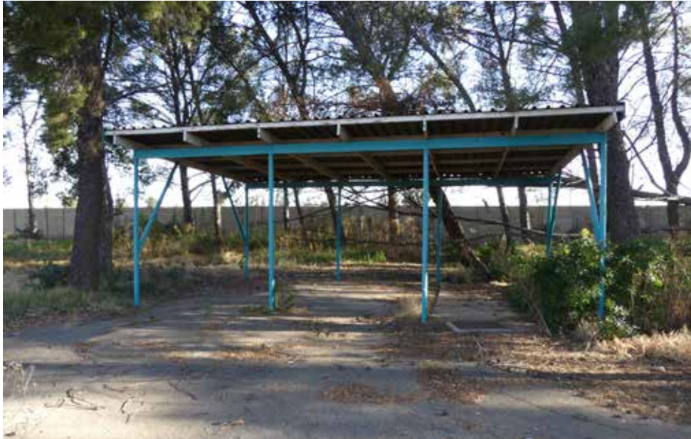
View of single sided carport - building 25.
