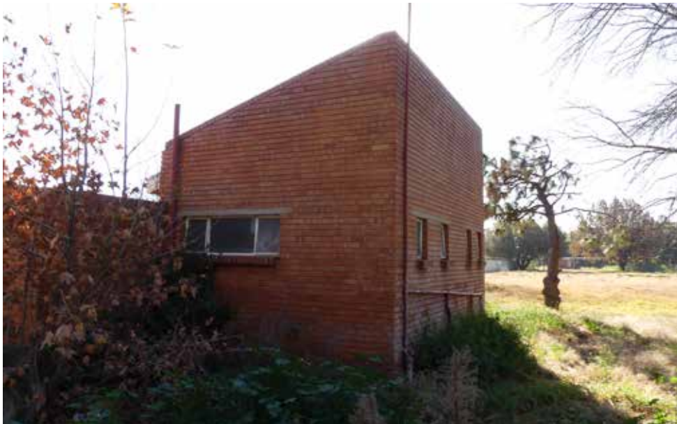
Toilet block - building 26.
