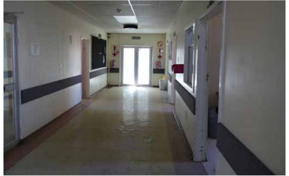
Corridor on Third Floor - building 17.
