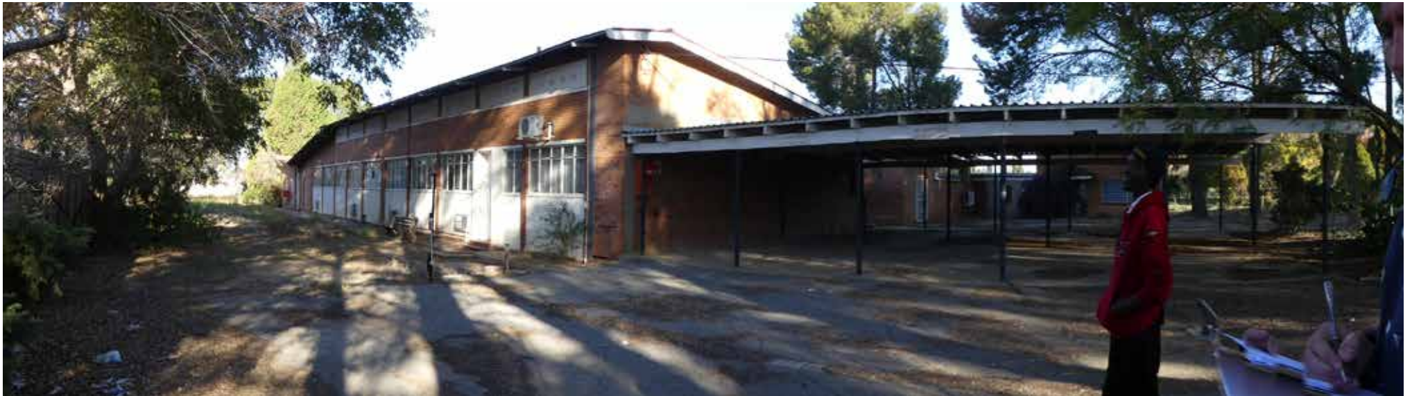
Panoramic view of front (North elevation) of building 13.
