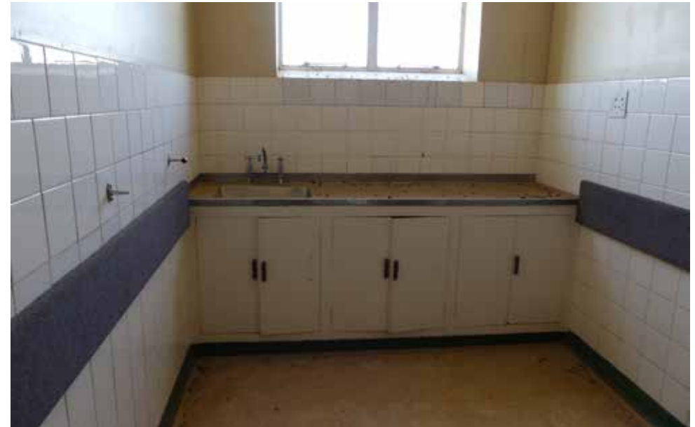
Original cupboards and sink in ward on Third Floor- building 17.
