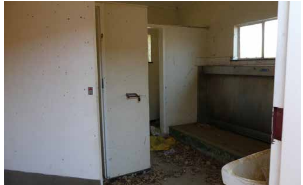
Interior of male toilets - building 26.
