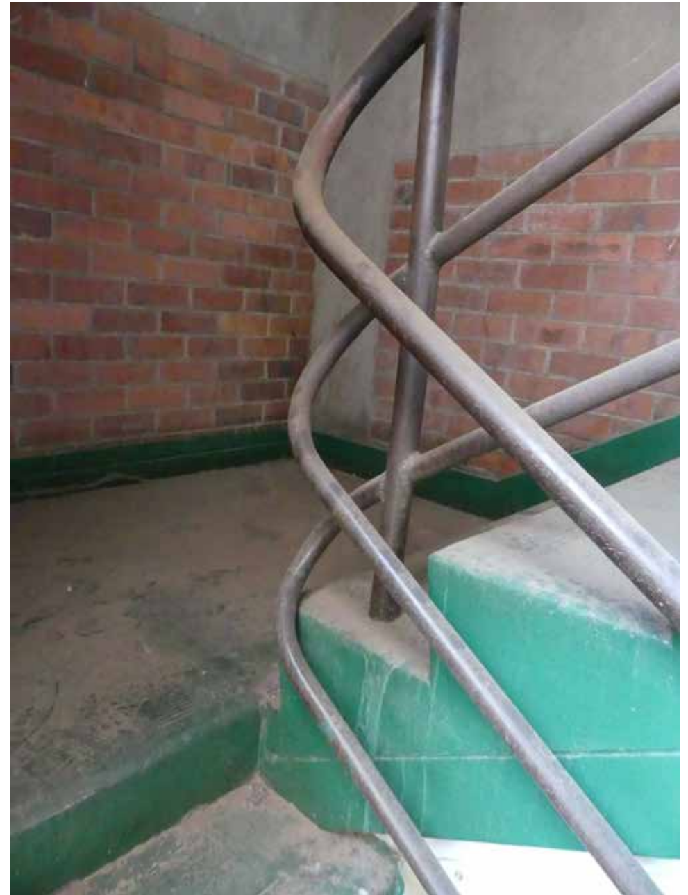
Detail of the fire escape handrail - building 17.
