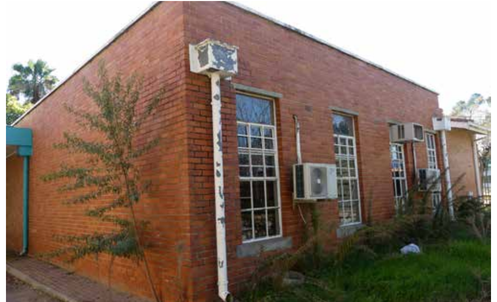
Southern elevation of Admin building - building 17.
