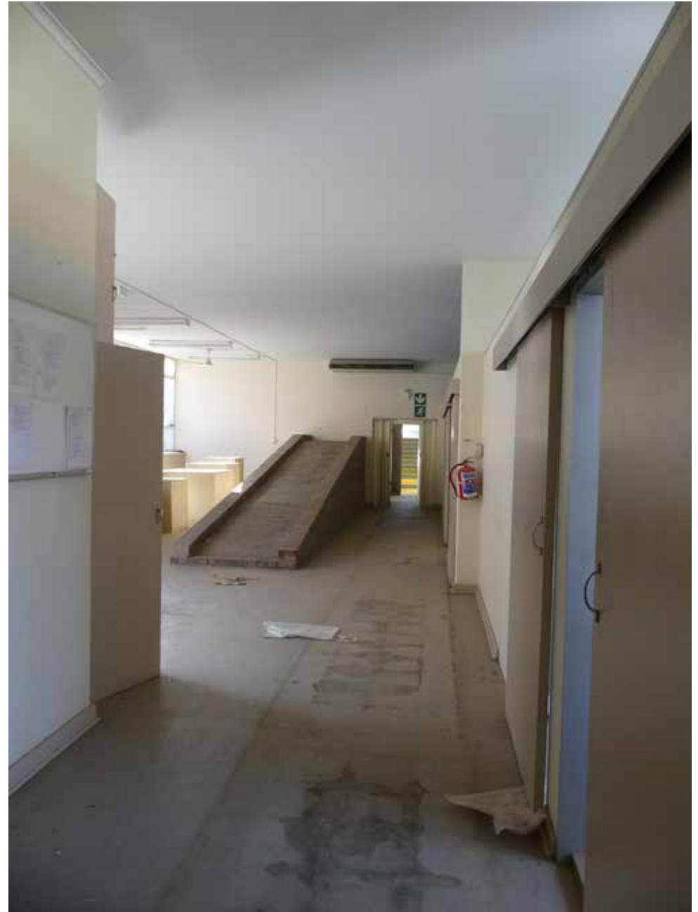
Interior of Laboratory building - building 23.
