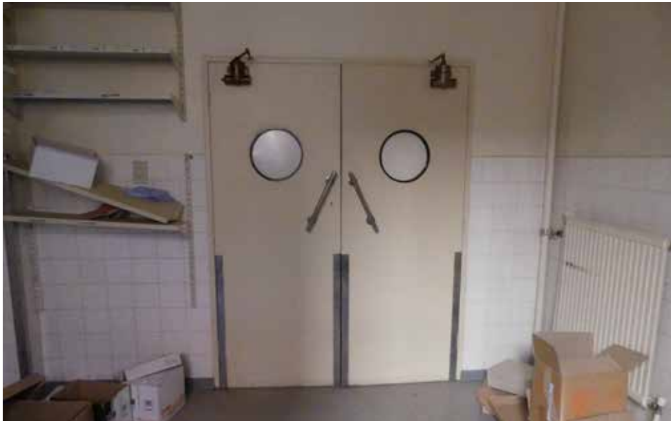
Original port hole doors to wards - building 17.
