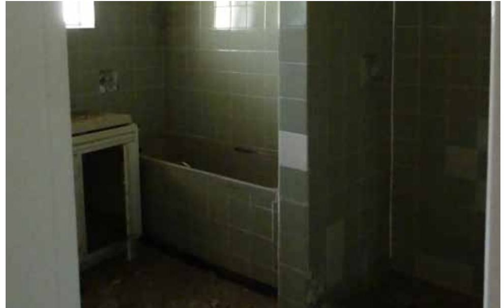
Family bathroom in building 7 - Doctor's House Type 6.
