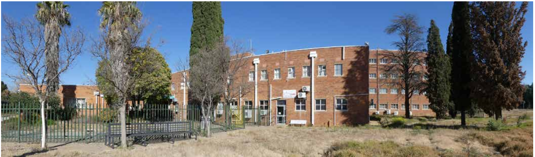
Panoramic view of Eastern elevation of building 17 - Main hospital casualty.
