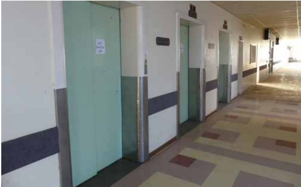
Original lift doors on Second Floor - building 17.
