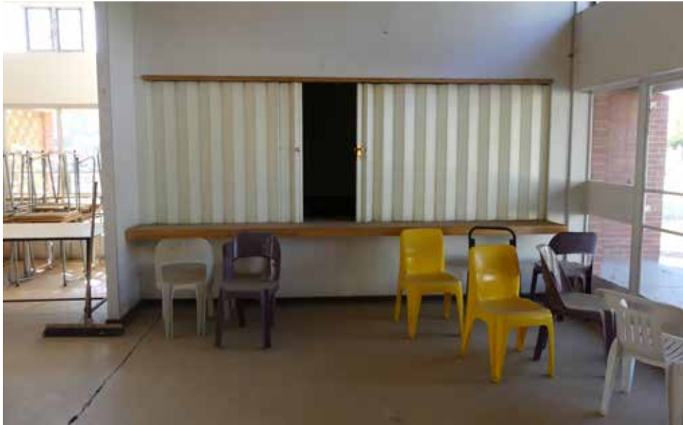
Serving hatch at back of building 14.
