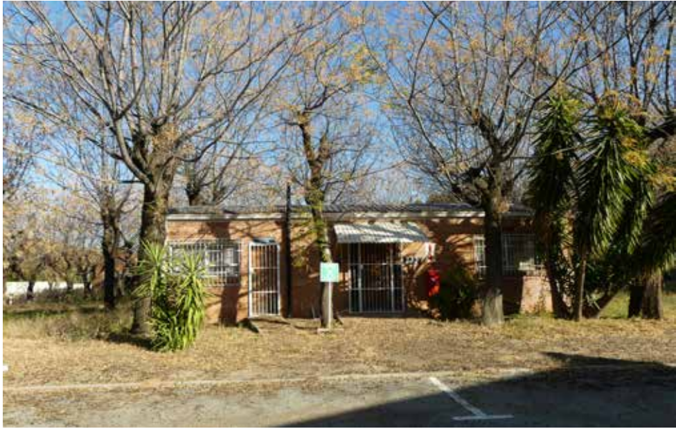
Northern elevation - building 30.
