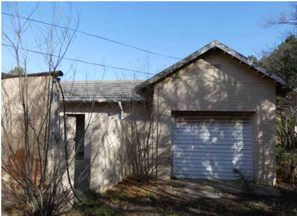
Garage of building 7 - Doctor's House Type 6.
