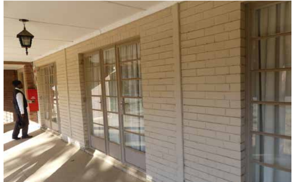
Detail of entrance into building - building 27.
