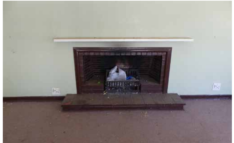
Original fire place in building 1 - Doctor's House Type 7.
