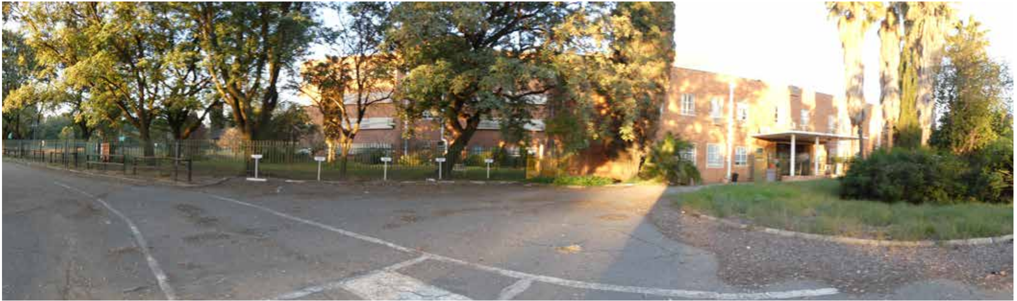
General site - looking East towards front of Hospital.
