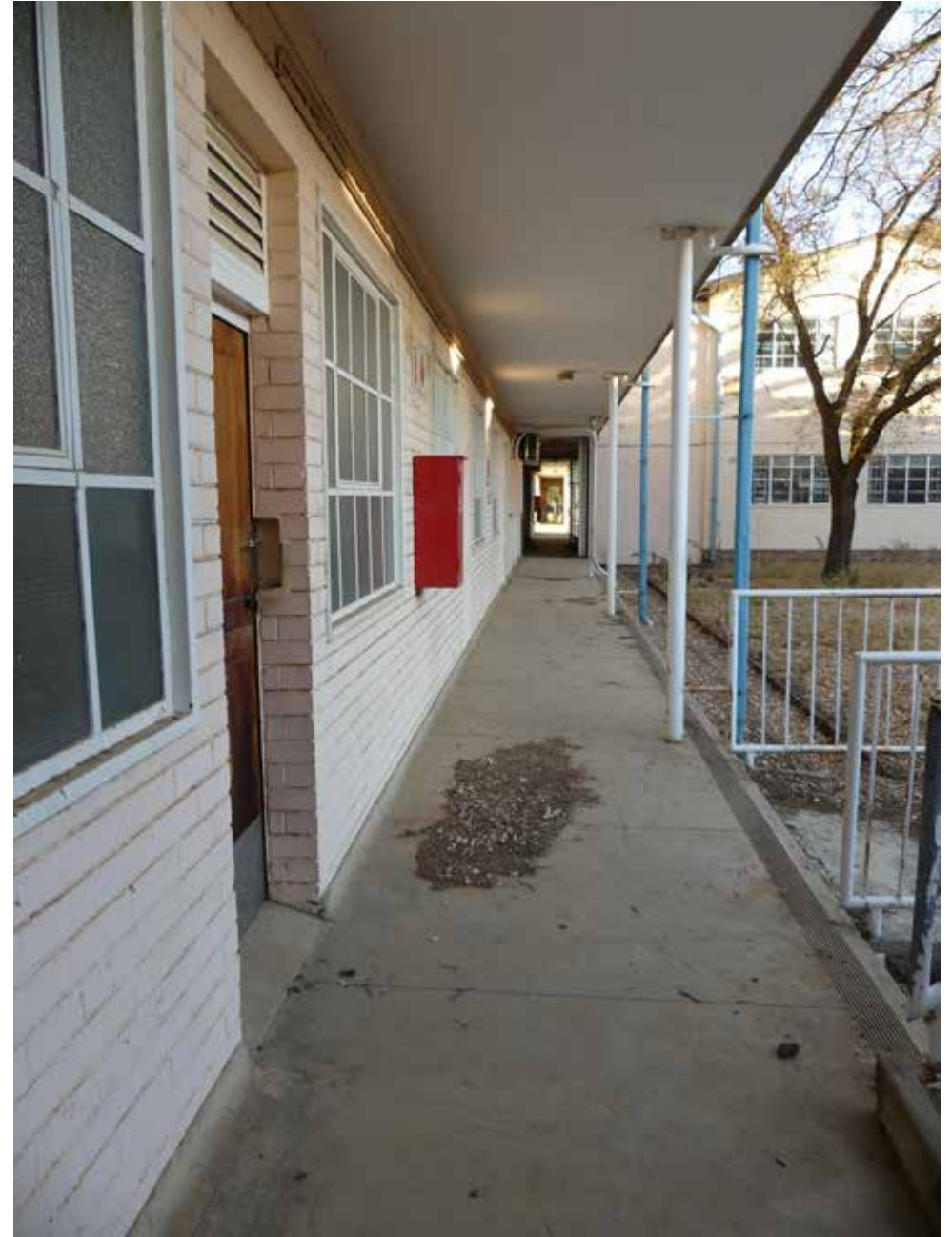
Exterior corridor - building 40.
