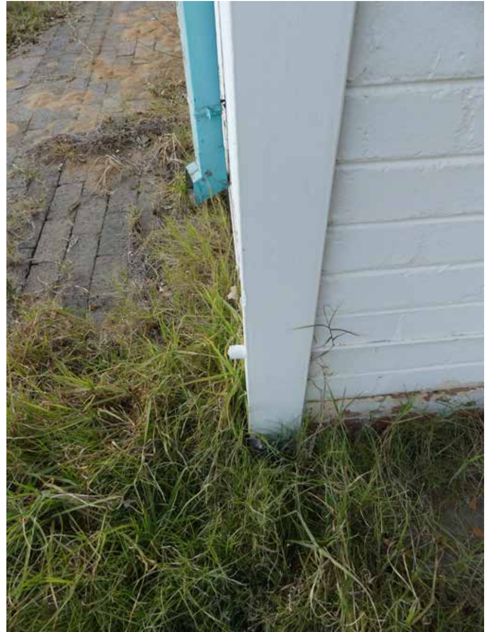
Edge detail - Steel frame and rods holding building together - building 39.
