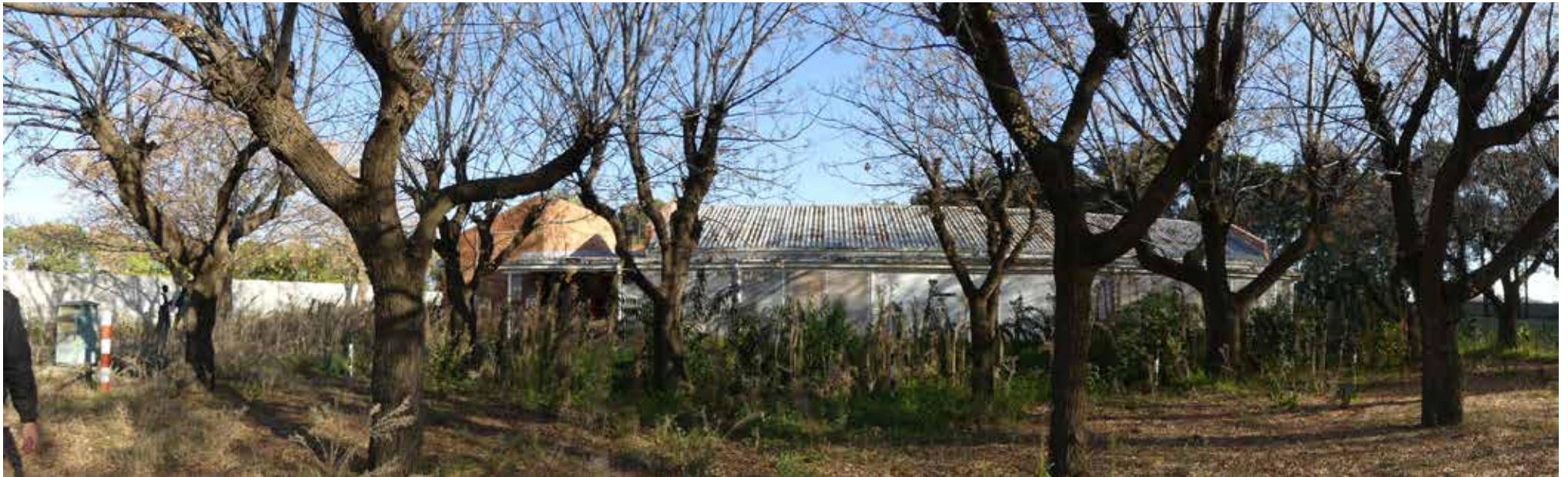
Northern elevation - building 33.
