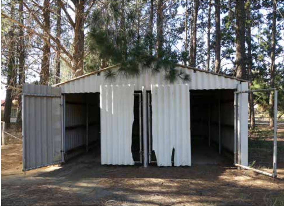
Front of building 10.
