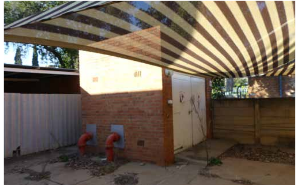
Entrance to pump house - building 29.
