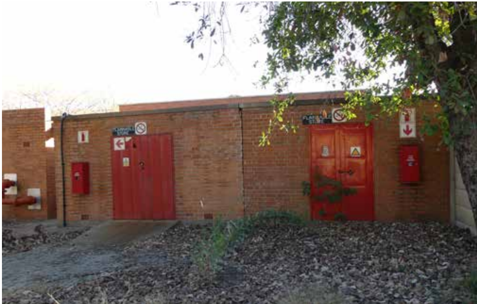
Flammable store - building 29.
