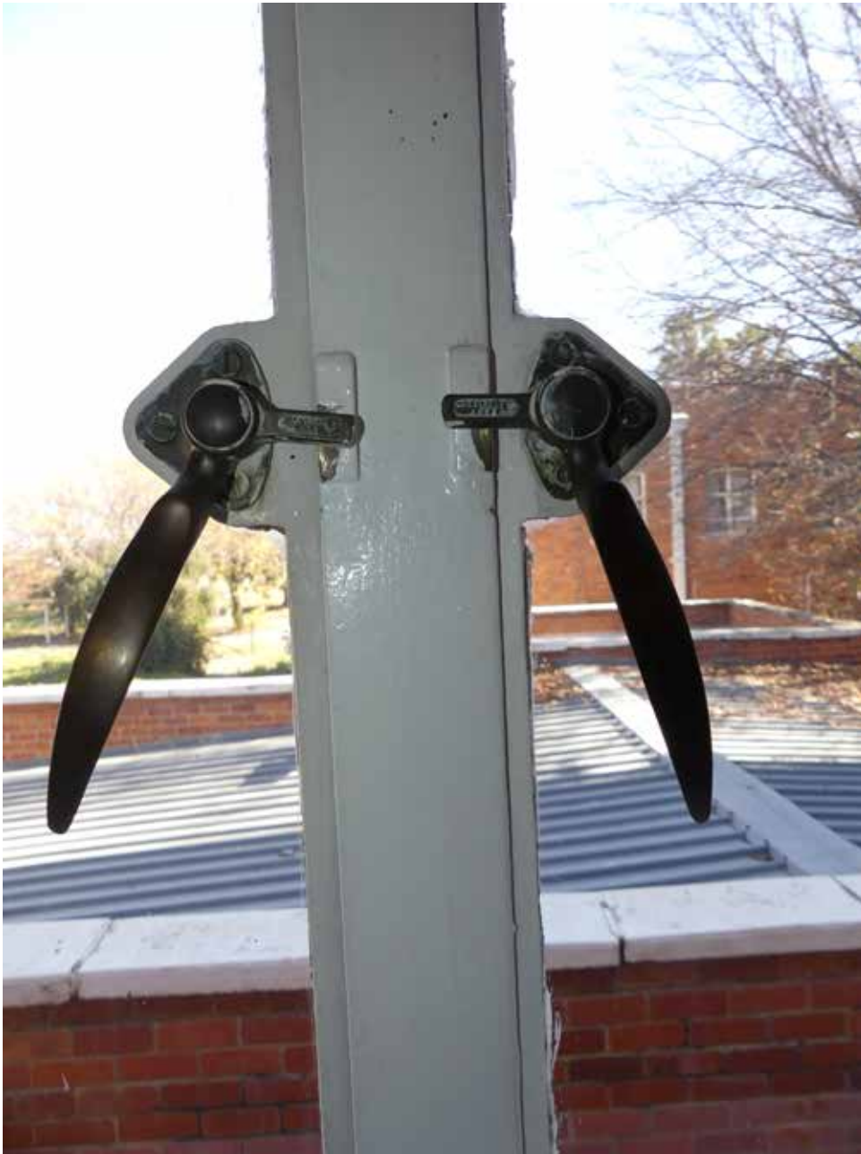
Original window hardware in link between Hospital and Laboratory building - building 17.
