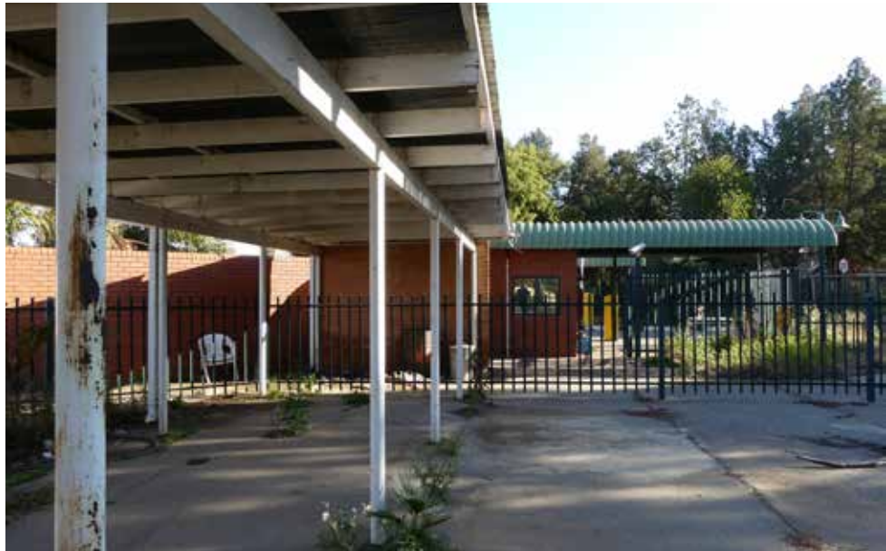
Exterior view of gate house from carport - building 15.
