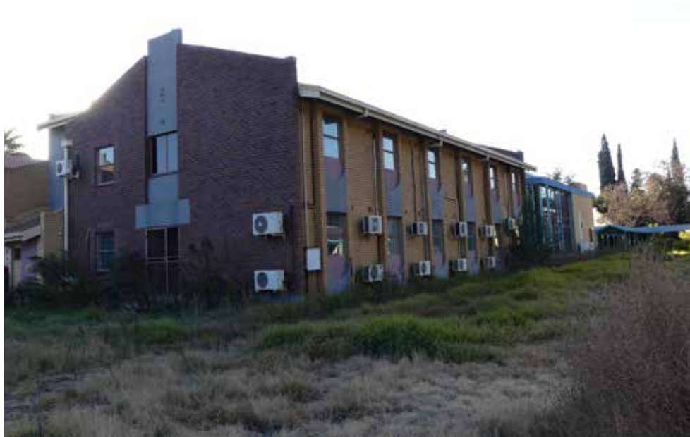
South, Eastern elevation - building 36.
