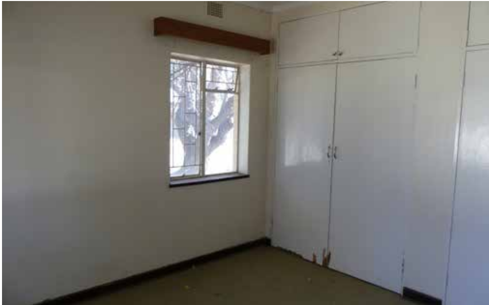
Bedroom in building 1 - Doctor's House Type 7.
