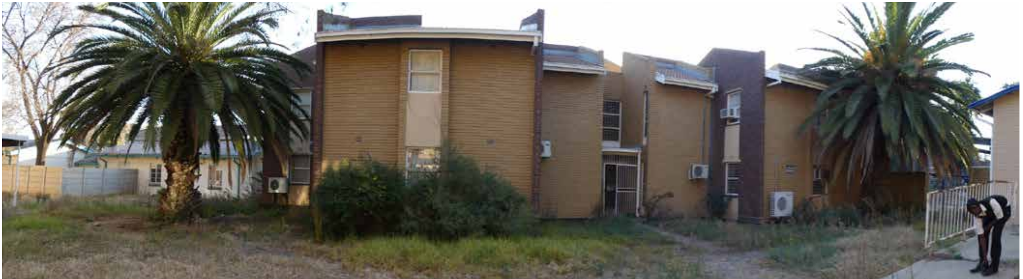
Eastern elevation - building 38.
