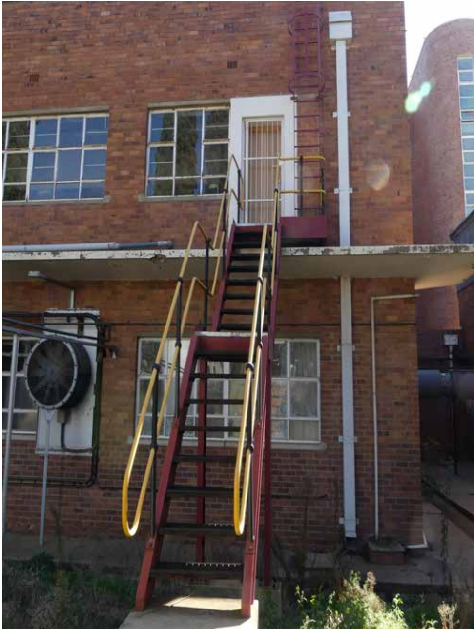
Fire escape from kitchen on First Floor - building 21.
