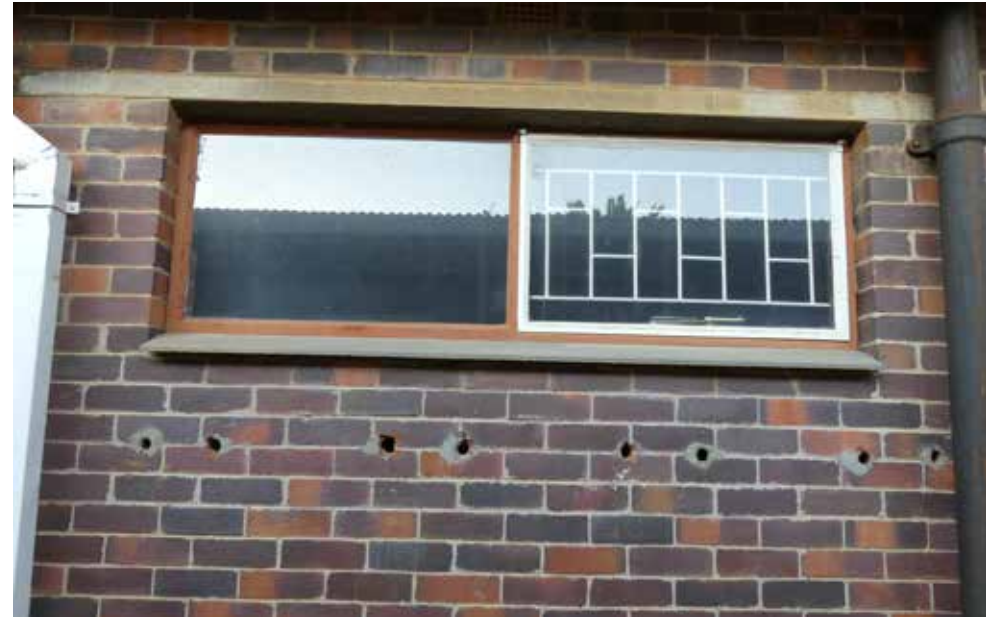
Window on Western elevation - building 42.
