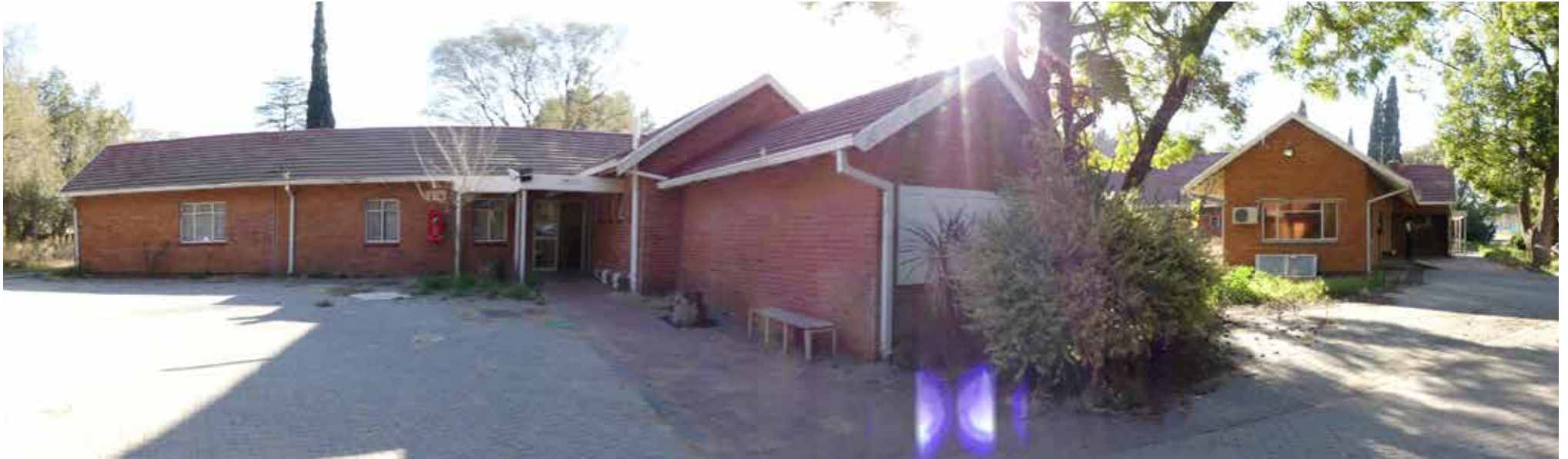
Panoramic view of Eastern elevation - building 16.
