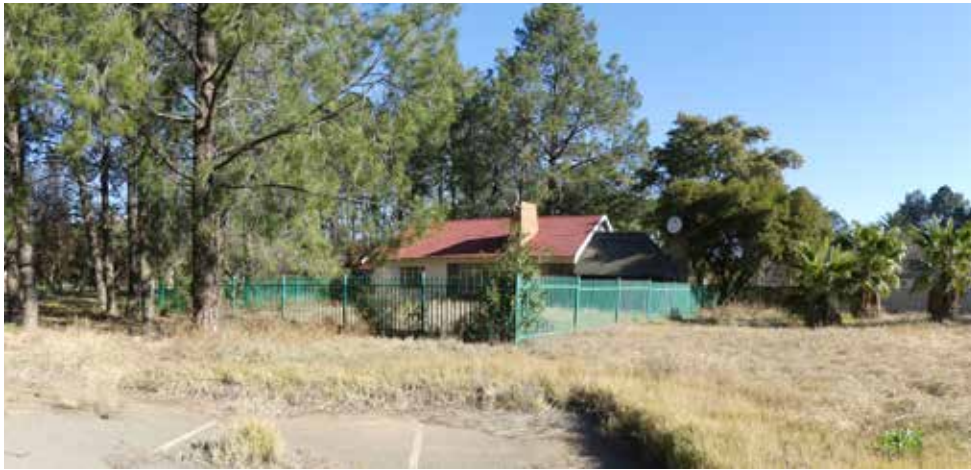
Panoramic view of building 8.
