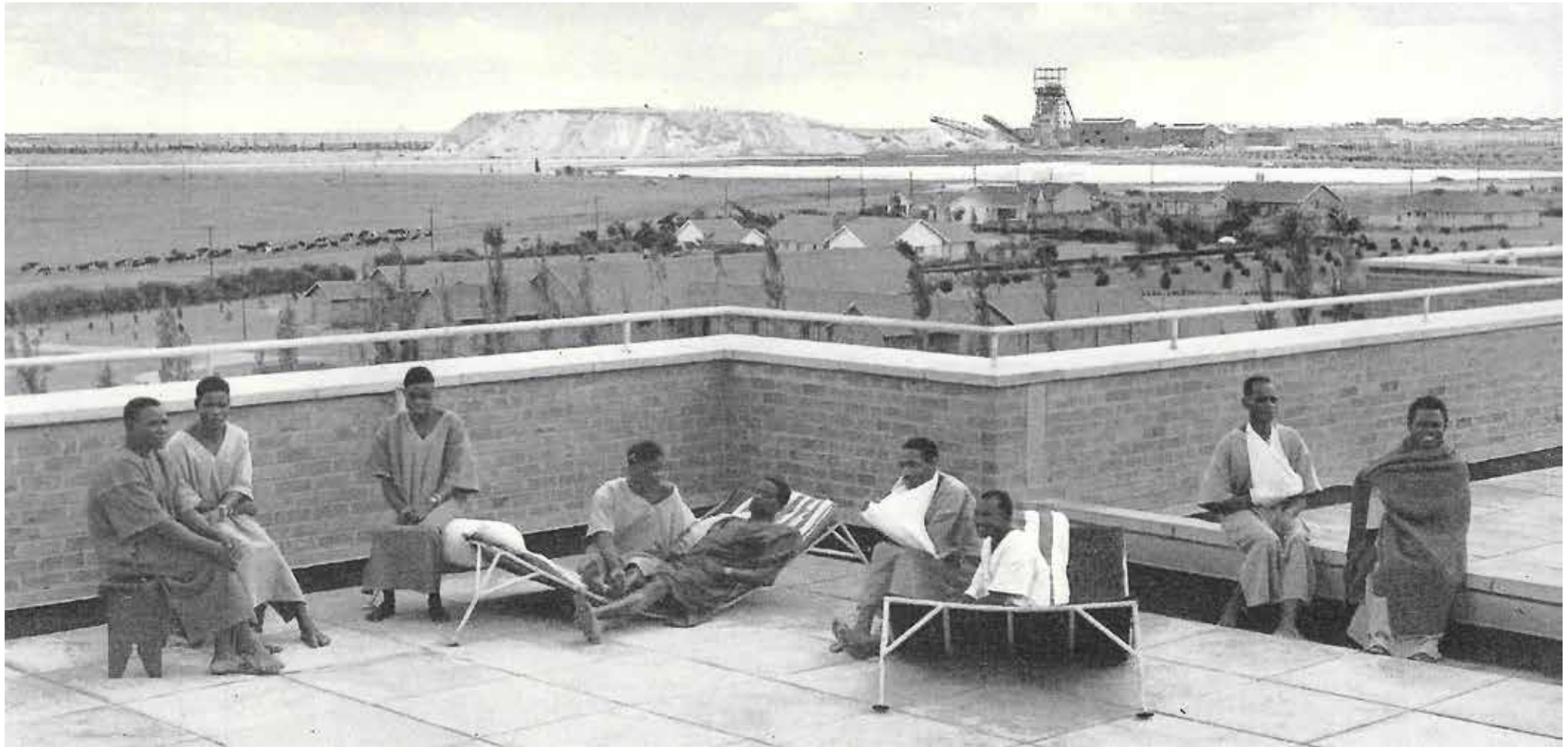
The roof of the hospital wards, designed to allow patients to convalesce in the sunlight and fresh air, as seen from this image of circa 1954 - at an undefined point the flat roof became ineffective and pitched corrugated sheeting was installed to waterproof the area - Anglo American Corporation, page 13.
