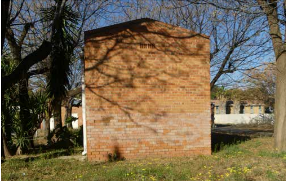
Western elevation - building 30.
