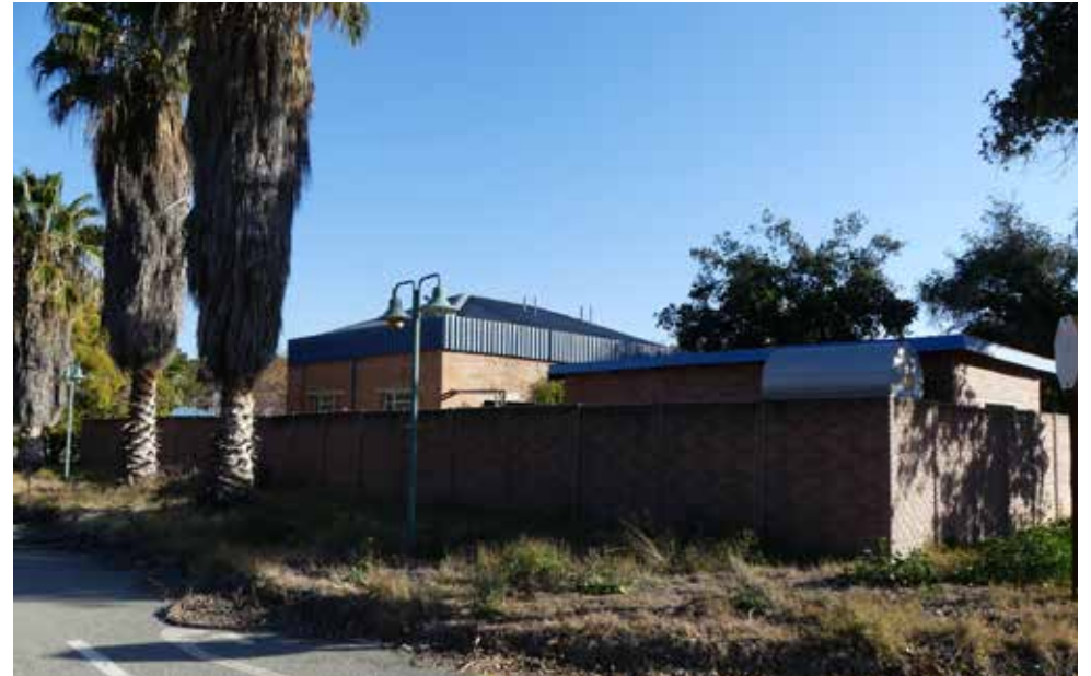
Eastern elevation - building 32.
