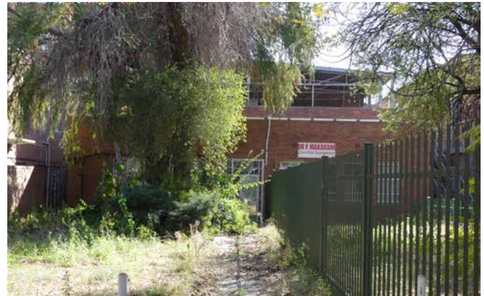
Southern elevation of X-Ray - building 22.
