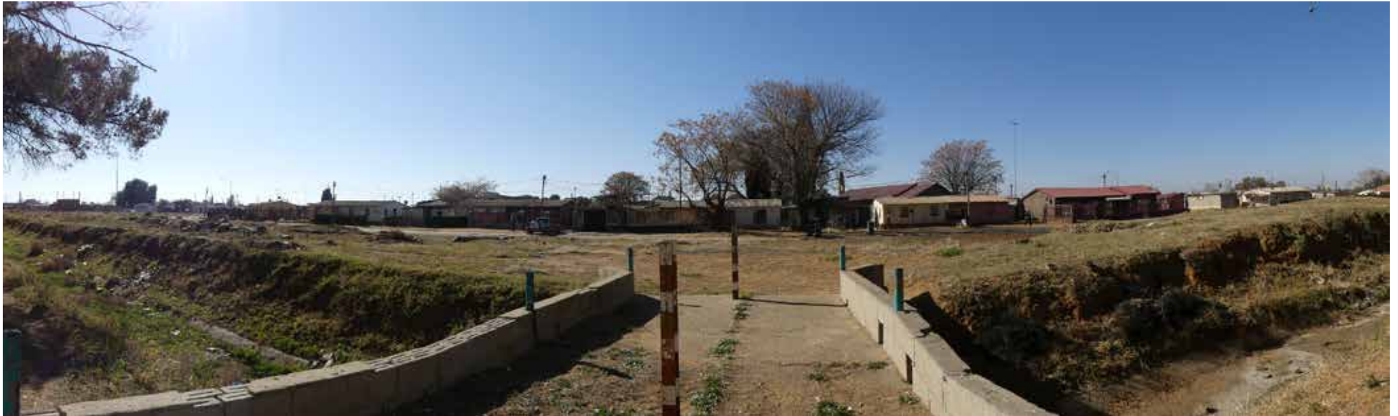
Exterior of site from Eastern access, pedestrian gate - Mokhomo Road.
