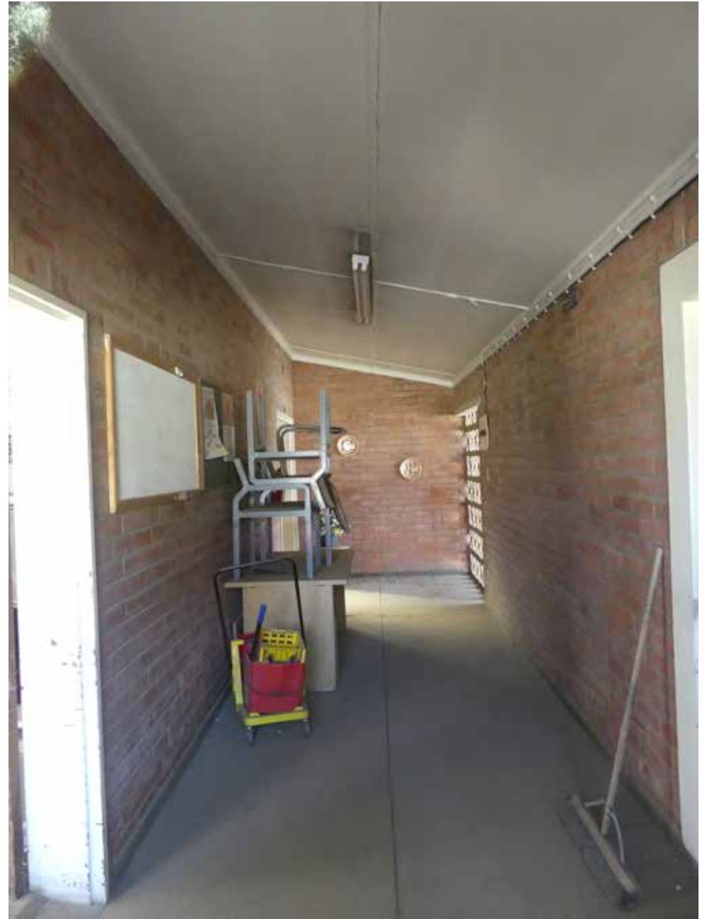
Interior of Mortuary - building 20.
