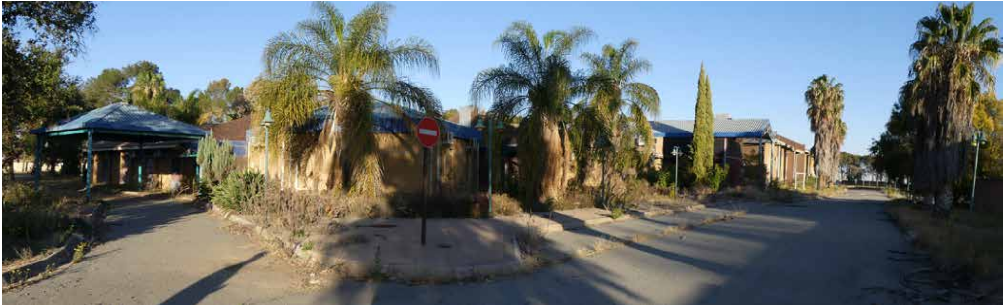
North, Western elevation - building 37.
