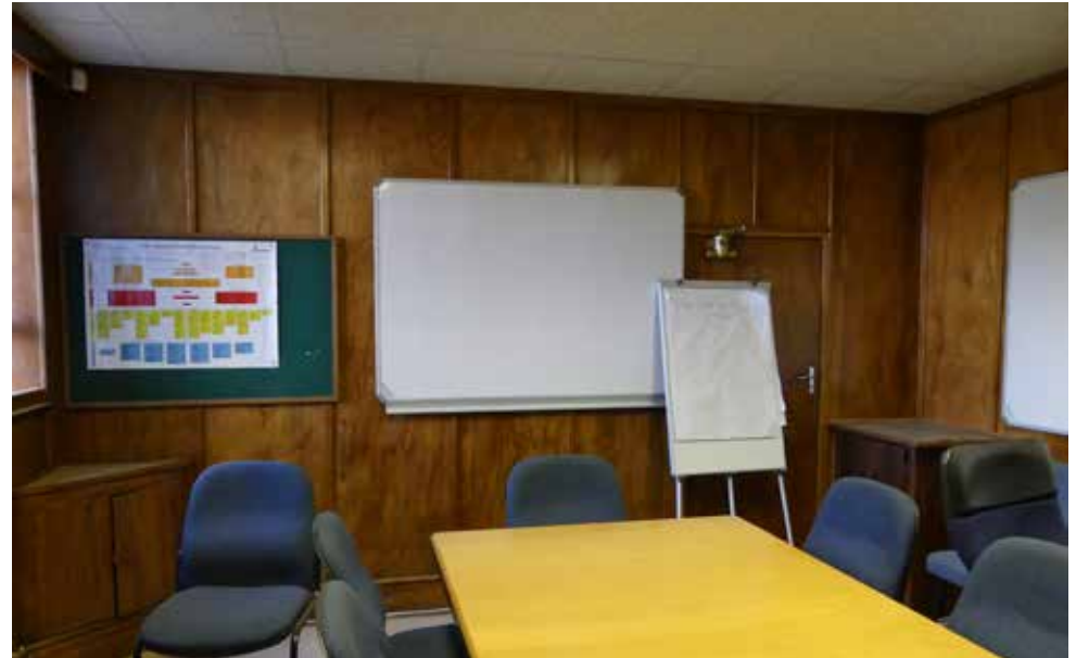
Wood panelling in the Boardroom of the Admin Building - building 17.
