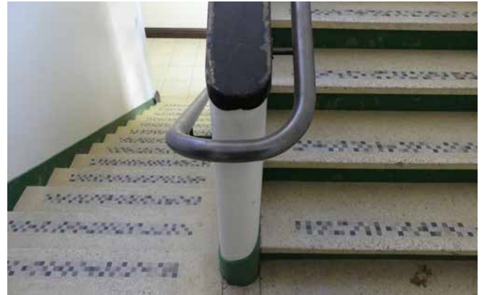
Original terrazzo and mosaic staircase to Admin (East) Block - building 17.
