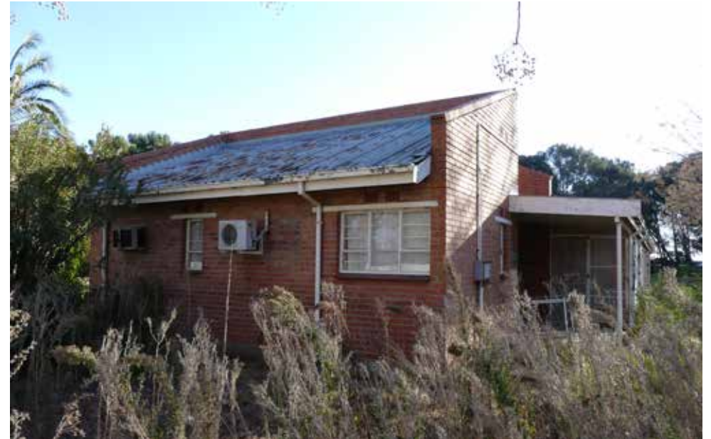
Eastern elevation - building 33.
