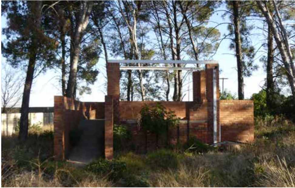
Northern elevation - building 45.
