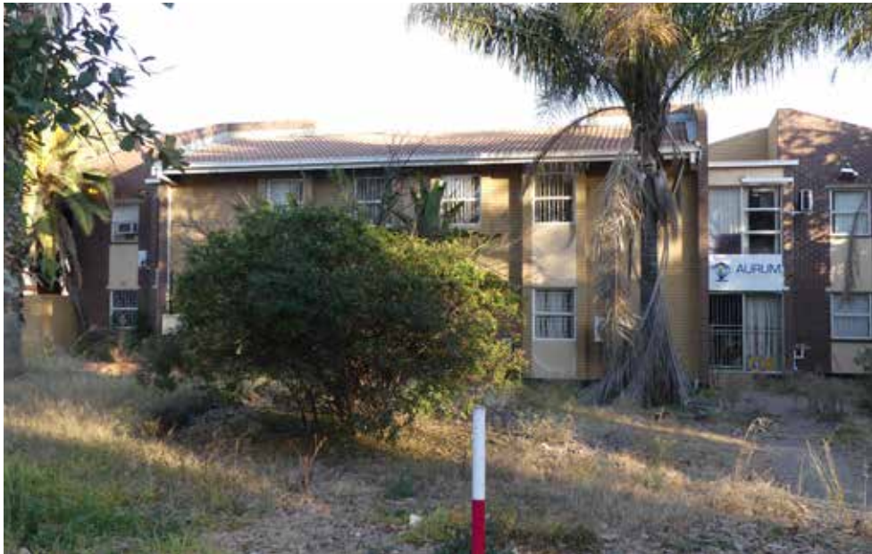
Northern elevation - building 38.
