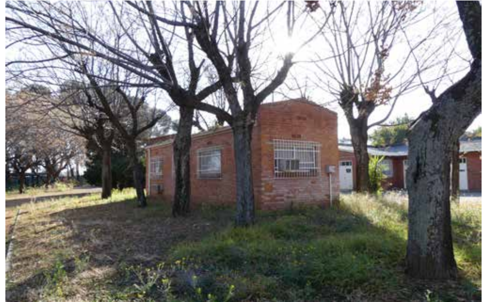
Eastern elevation - building 30.
