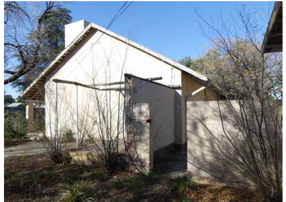
Side patio of building 7 - Doctor's House Type 6.
