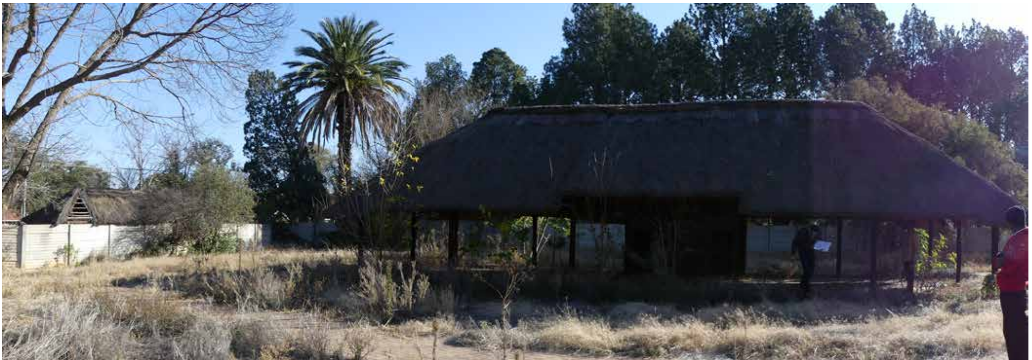
Thatch Lapa now in location of swimming pool - building 11.
