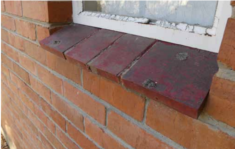
Detail of window cill - building 33.
