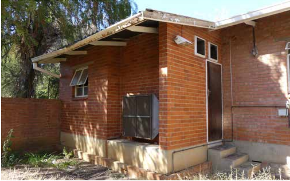
Northern elevation of Mortuary - building 20.
