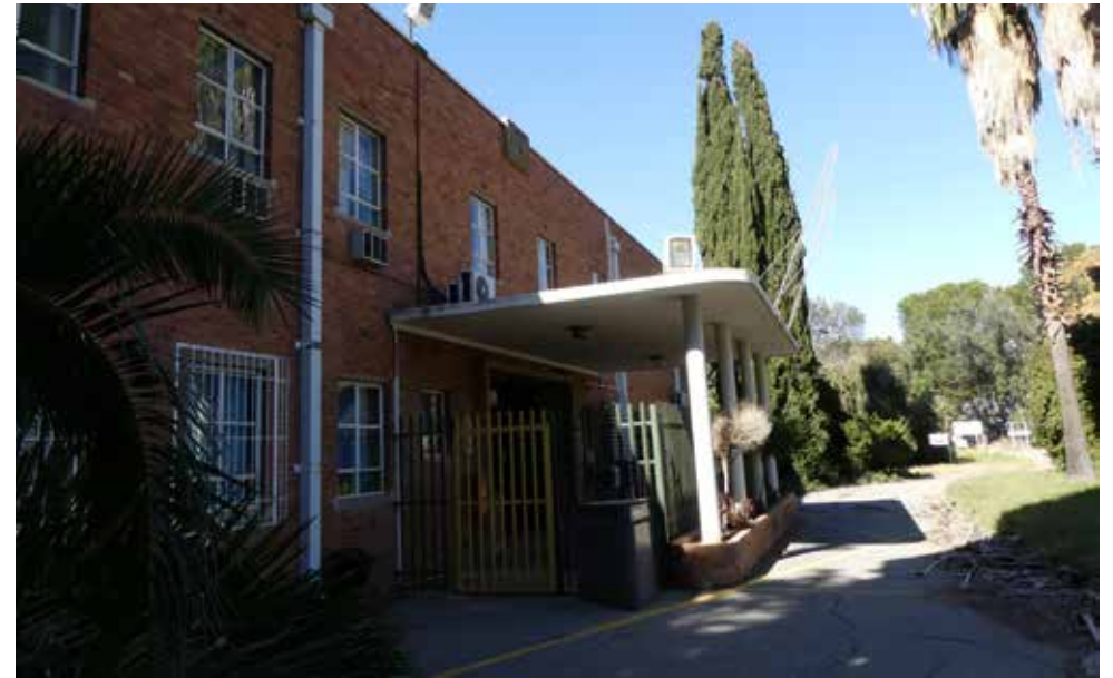
Portico to Administration Block - building 17.
