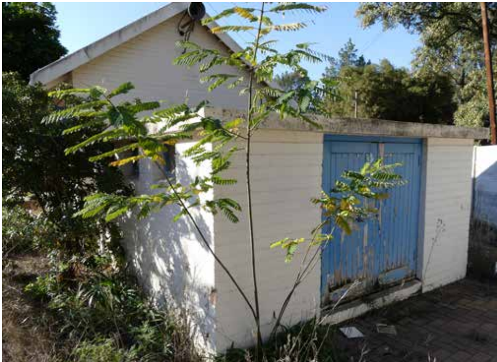
Addition to side of building 11.
