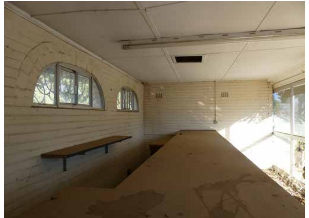
Interior of building 11.
