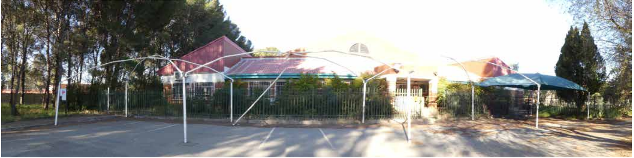
Panoramic view of Eastern elevation of building 12.
