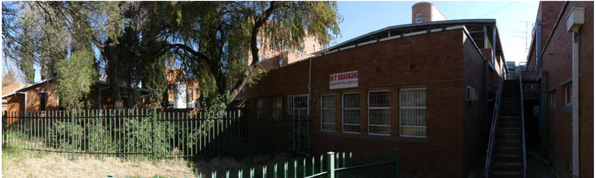
Southern elevation of X-Ray - building 22.
