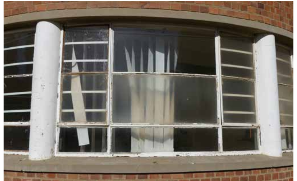
Curved windows of 1957 (additional) wards - building 17.
