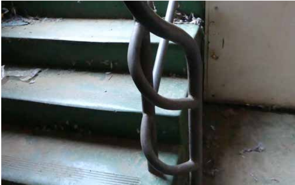
Detail of the fire escape - building 17.
