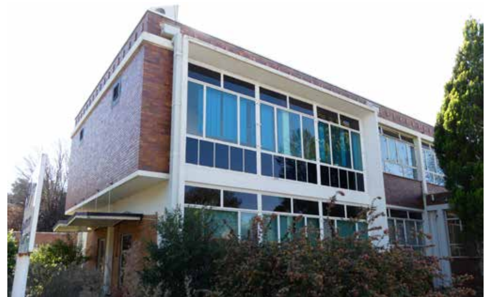
South / Western elevation of Laboratory - building 23.
