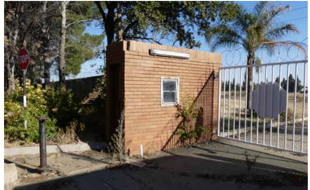
Gate House - building 26.
