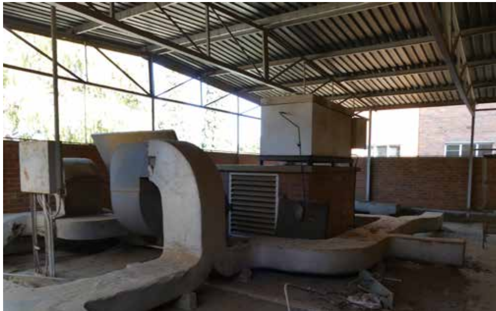
Roof of X-Ray building - building 22.
