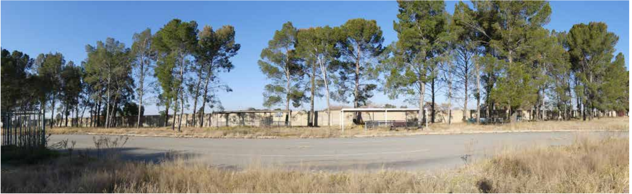
Eastern elevation - building 44.
