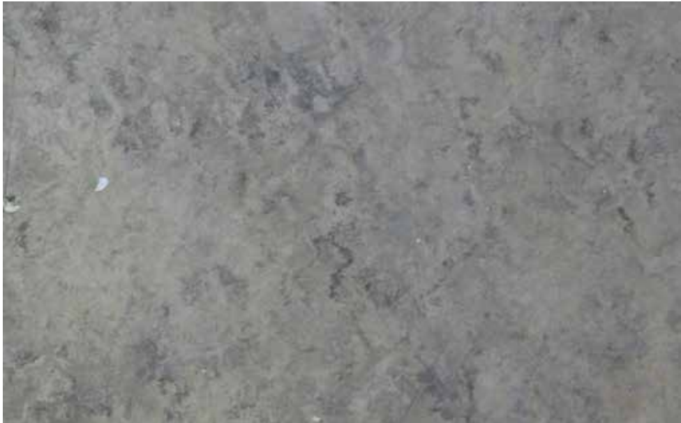
Original Linoleum on Third Floor - building 17.
