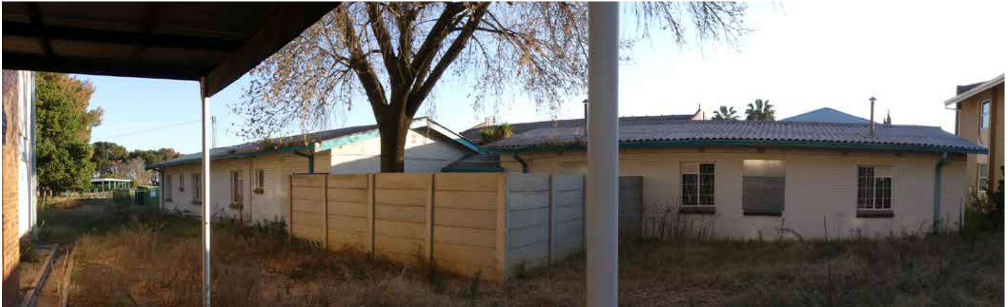
Eastern elevation - building 39.
