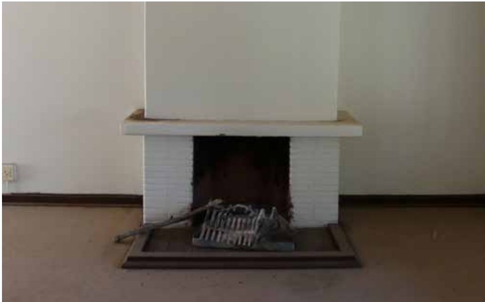
Fire place in lounge of building 3 - Doctor's House Type 6.
