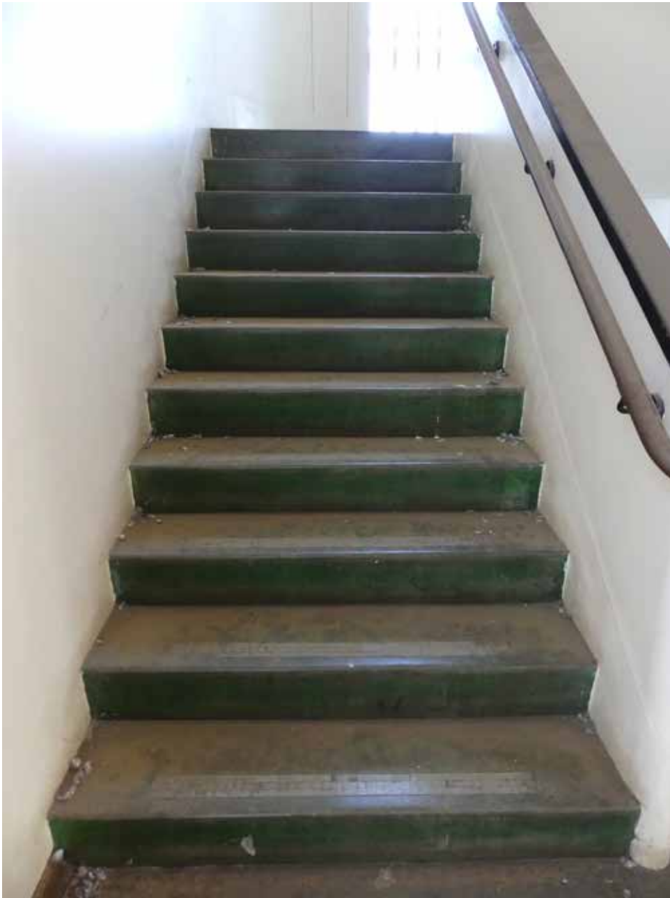
Original staircase with terrazzo and mosaics - building 17.
