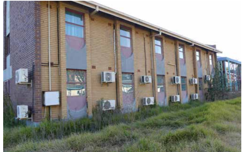
Eastern elevation - building 36.
