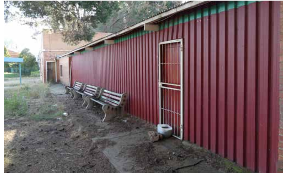
Part of South elevation of building 13.
