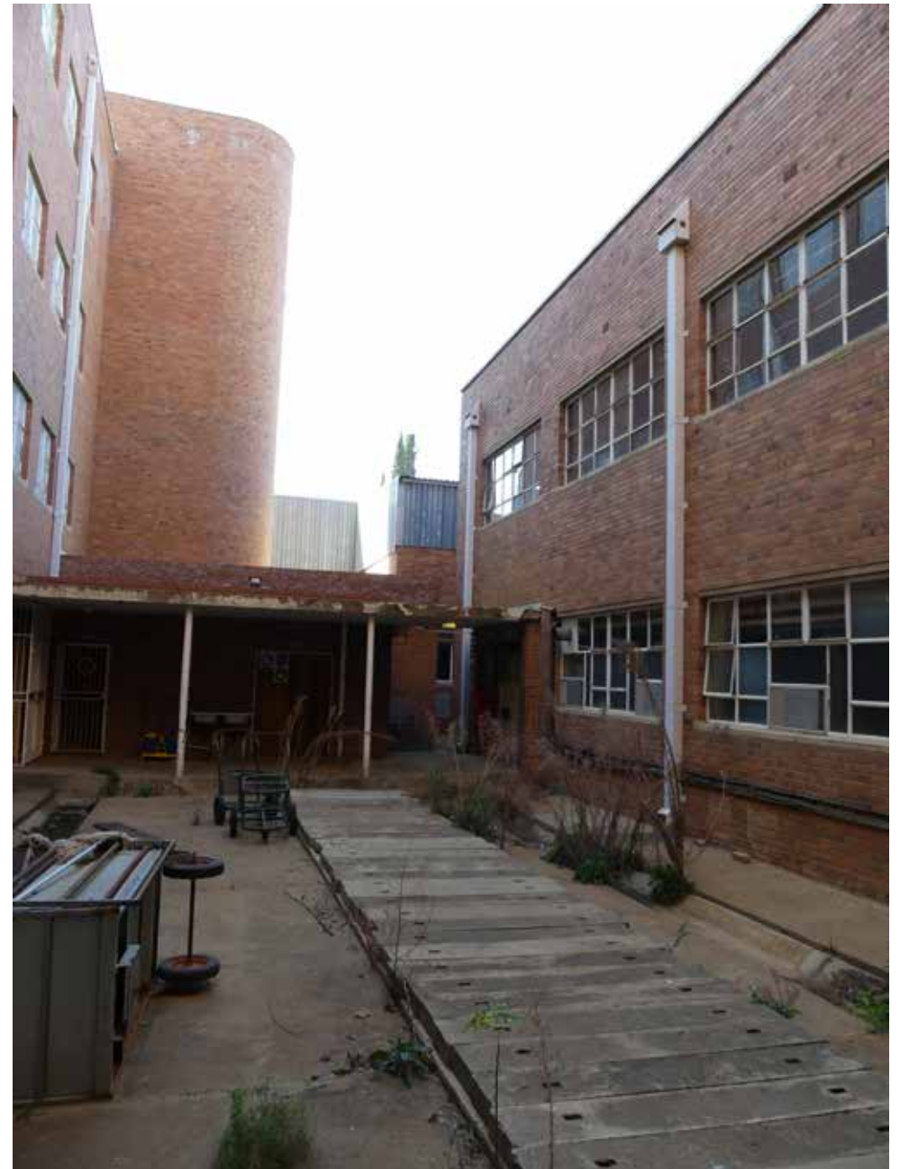
Laundry courtyard - building 21.
