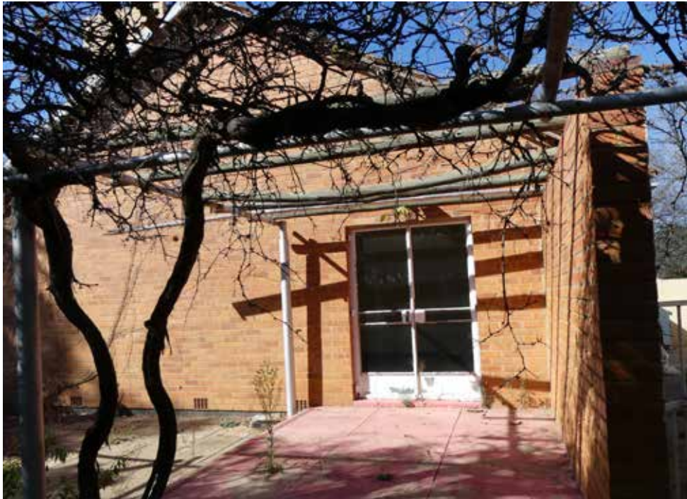
Original brick on side patio of building 3 - Doctor's House Type 6.
