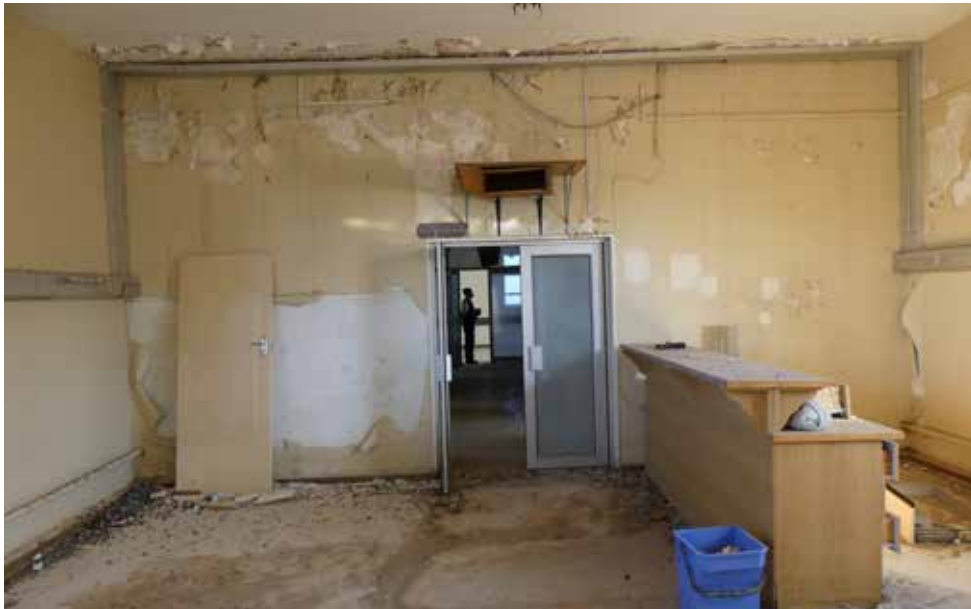
Ward on Third Floor - building 17.
