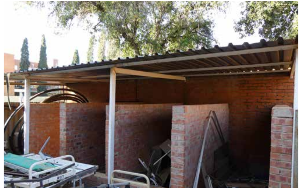
Part of flammable store area - building 29.
