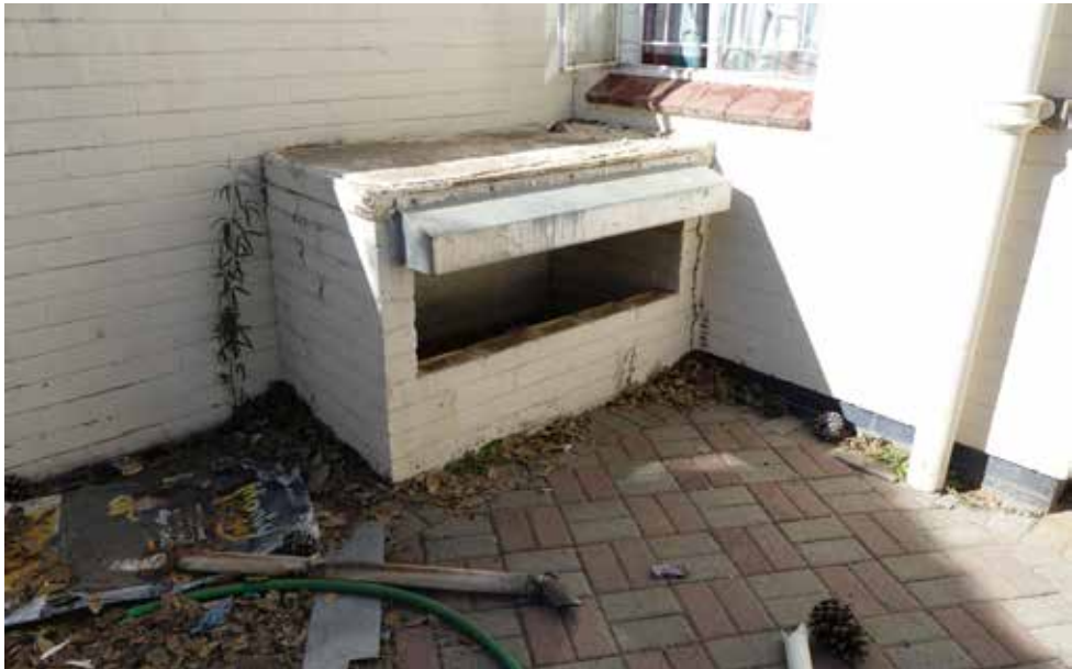
Kitchen courtyard and coal shed of building 2 - Doctor's House Type 7.
