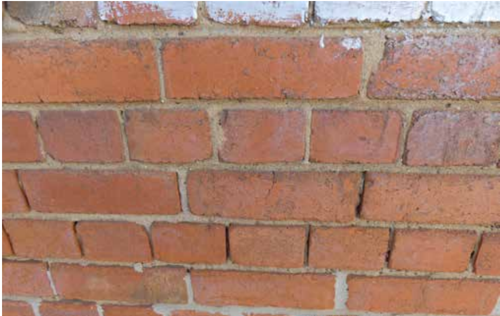
Detail of brick bond - building 31.
