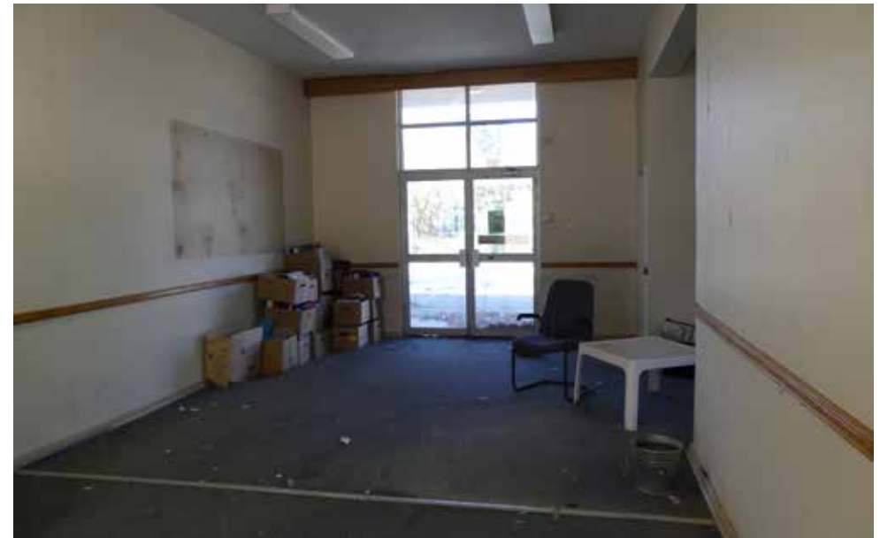
Interior of Laboratory building - building 23.
