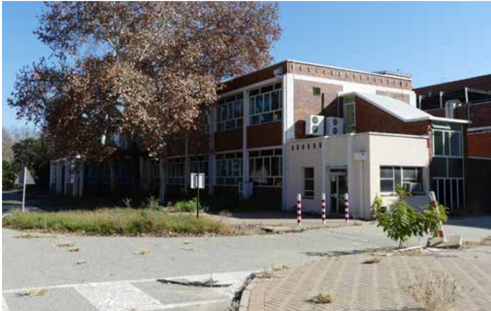
South / Eastern elevation of Laboratory building - building 23.
