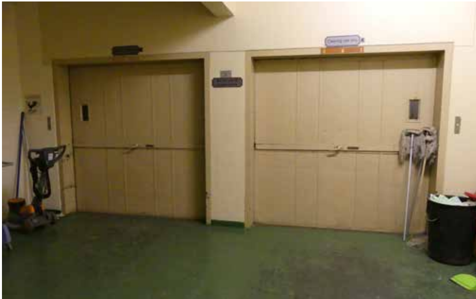
Original doors to the service elevators - building 17.
