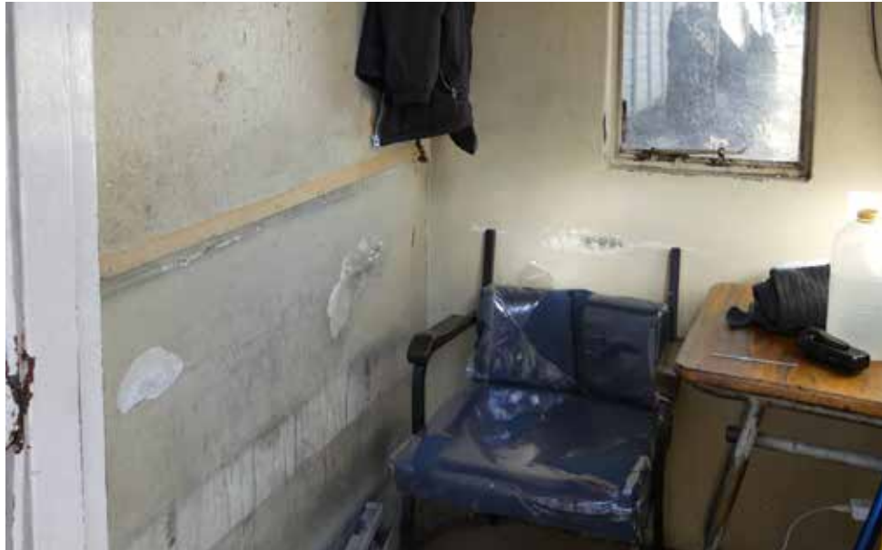
Interior of Pedestrian Guard House - building 19.
