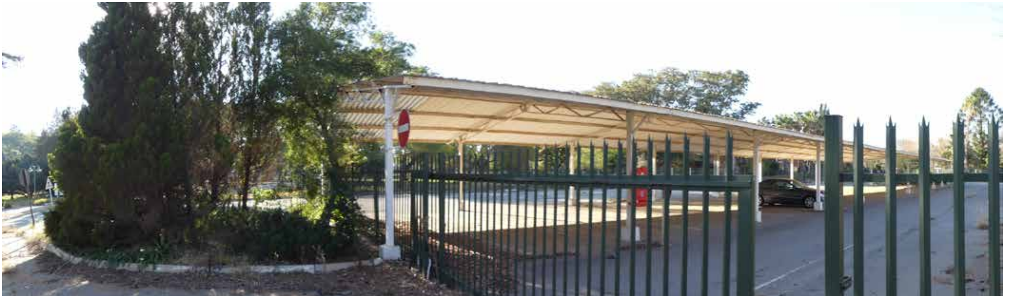
Panoramic view of carport - building 15.
