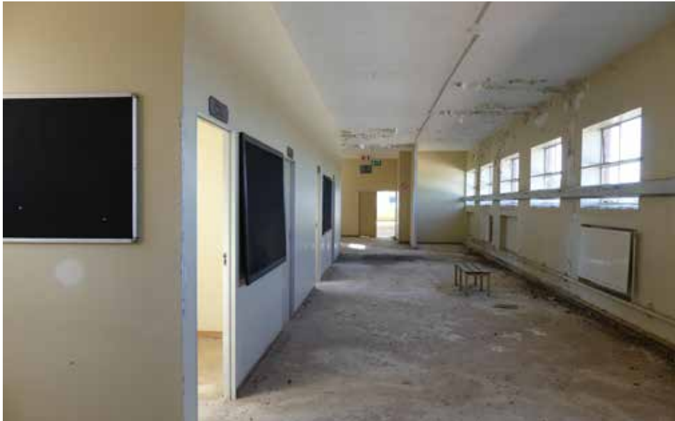
Ward on Third Floor - building 17.
