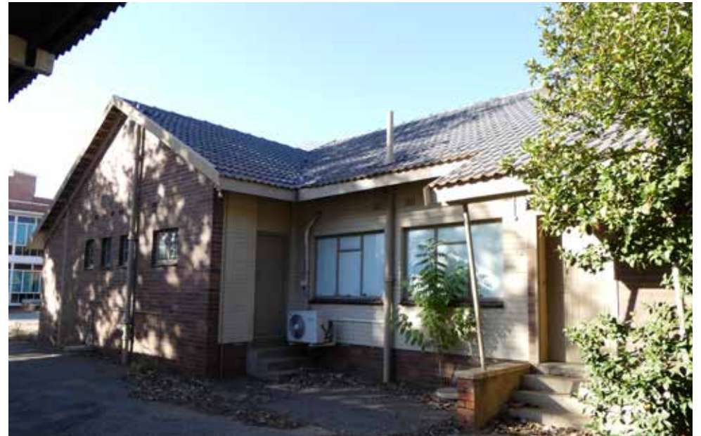
Western elevation - building 27.
