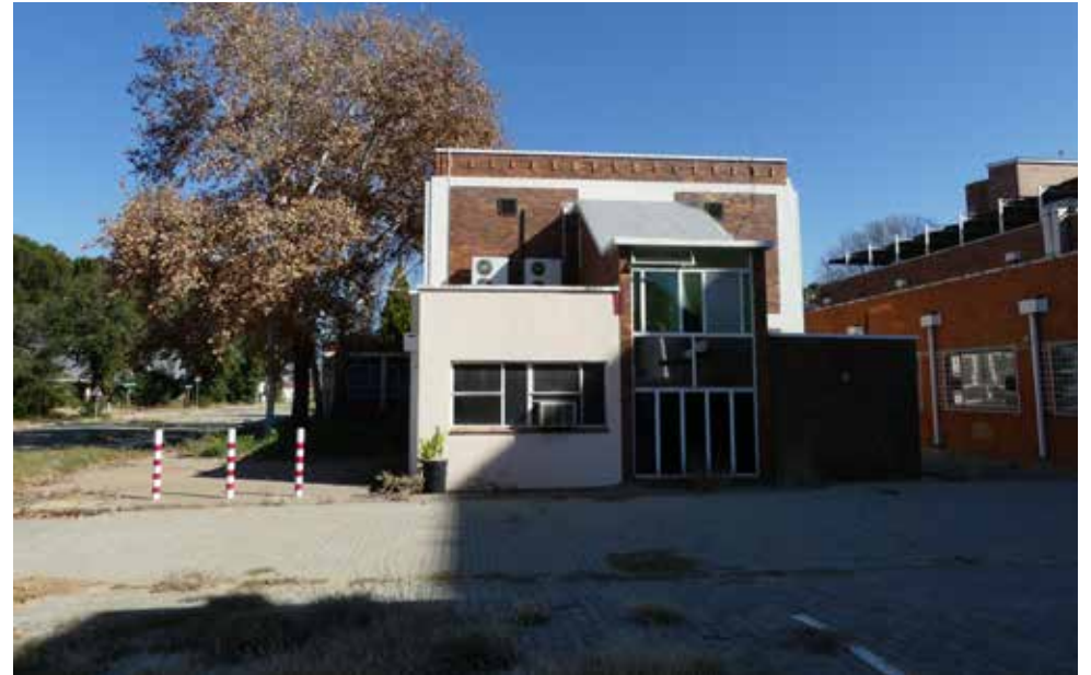
Eastern elevation of Laboratory building - building 23.
