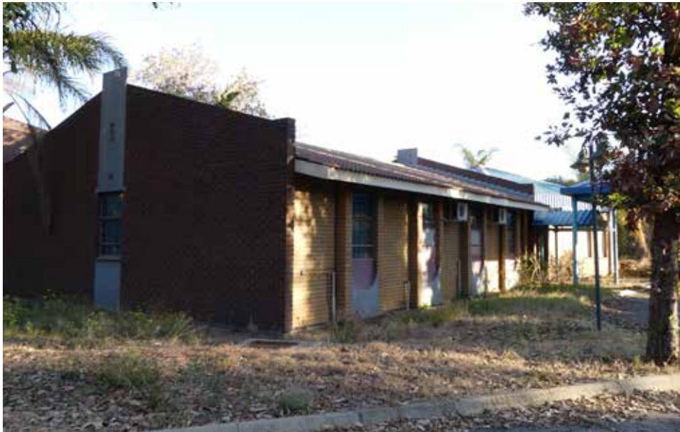
Northern elevation - building 37.
