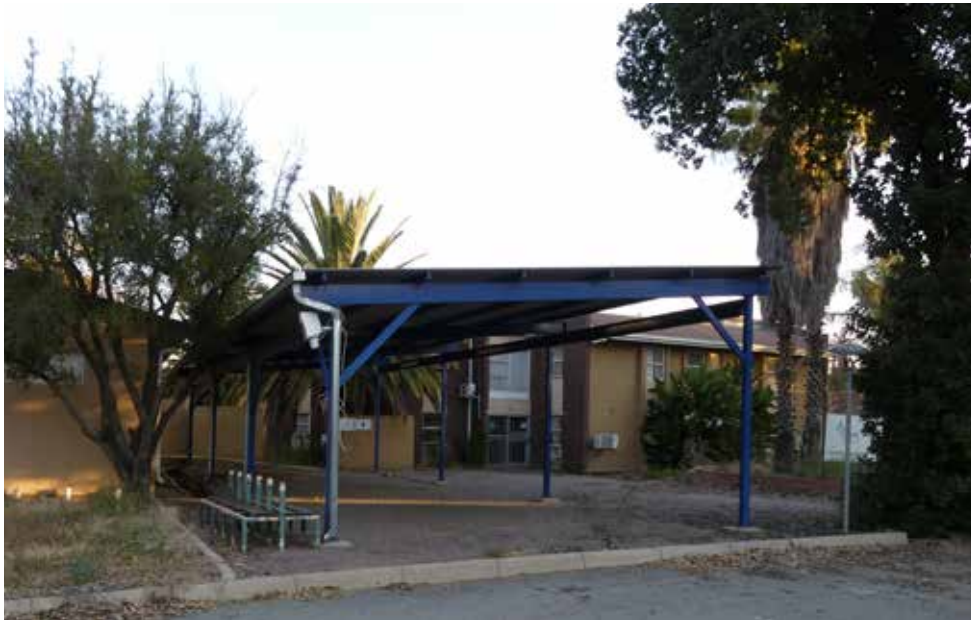
Northern elevation - building 43.
