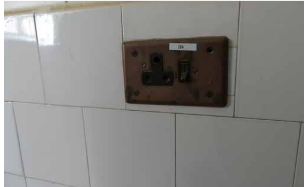
Original plug on Third Floor - building 17.
