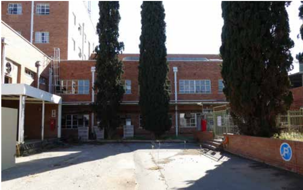
Southern elevation of Laundry & Kitchen - building 21.
