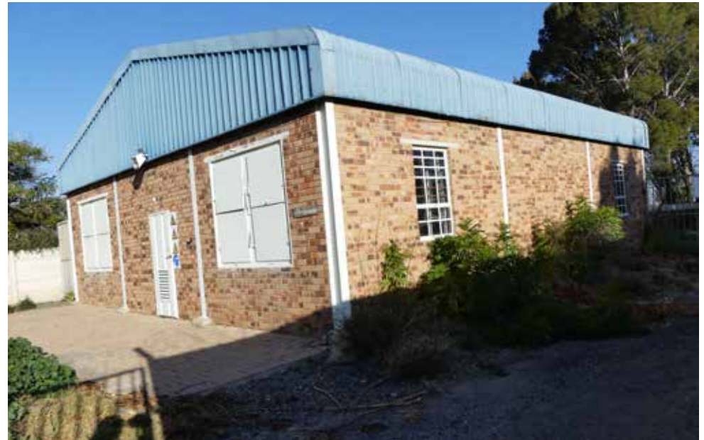
North, Western elevation of electrical room - building 34.
