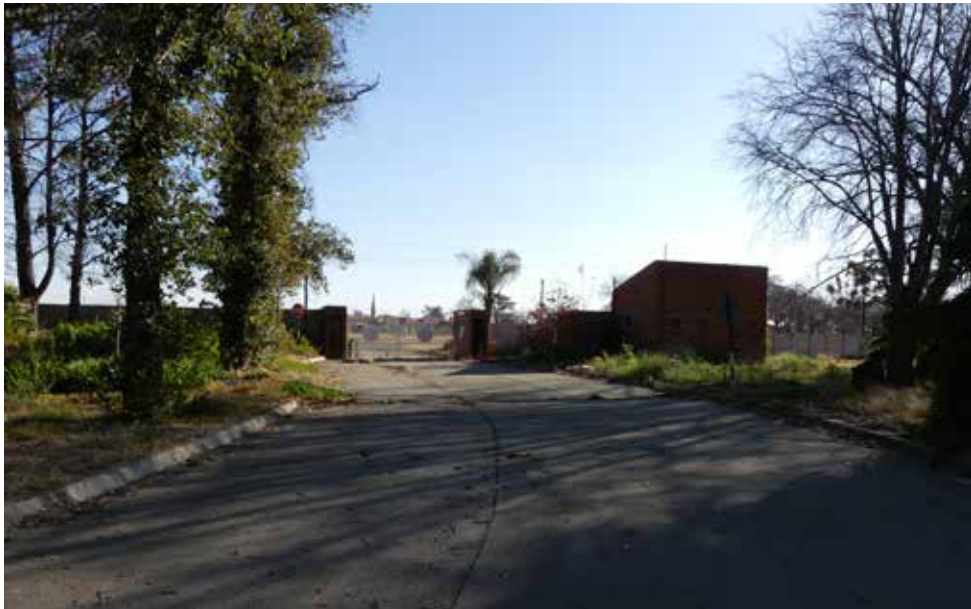
Eastern elevation of Gate House and Toilet block - building 26.
