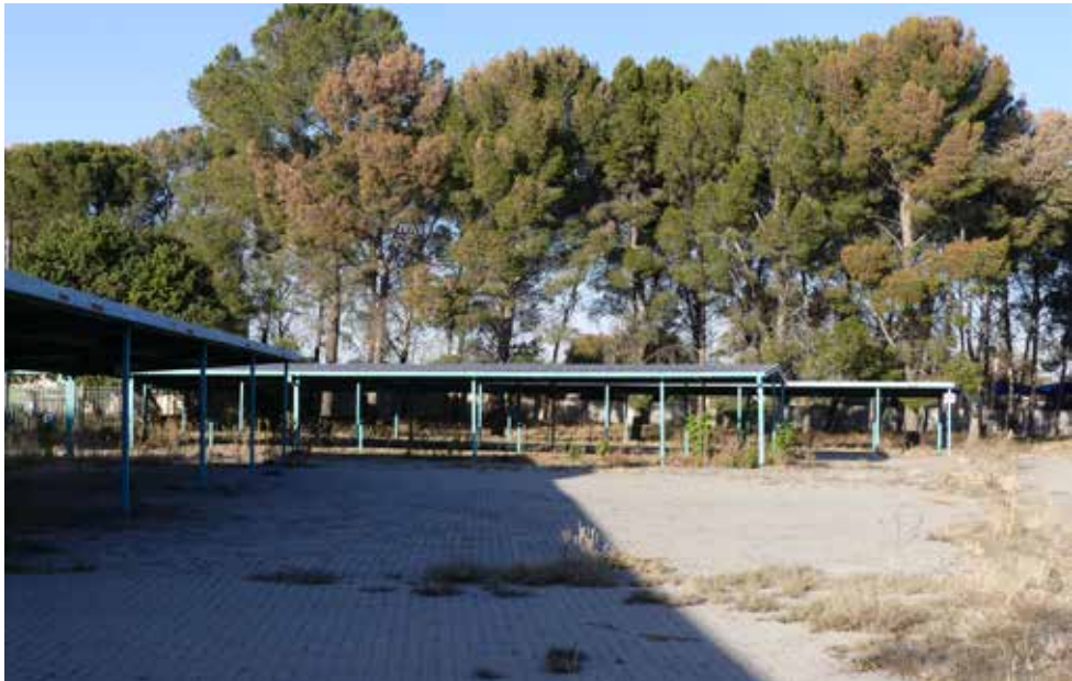
Western elevation of carports - building 35.
