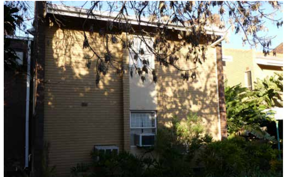
Partial Southern elevation - building 38.
