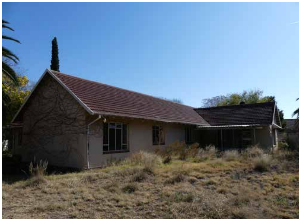
Back elevation of building 1 - Doctor's House Type 7.
