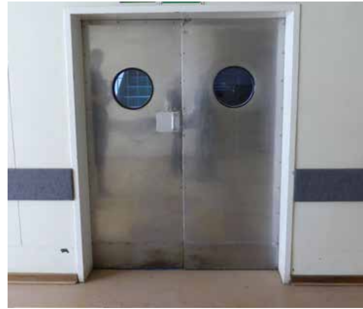
Modified original fire doors - building 17.
