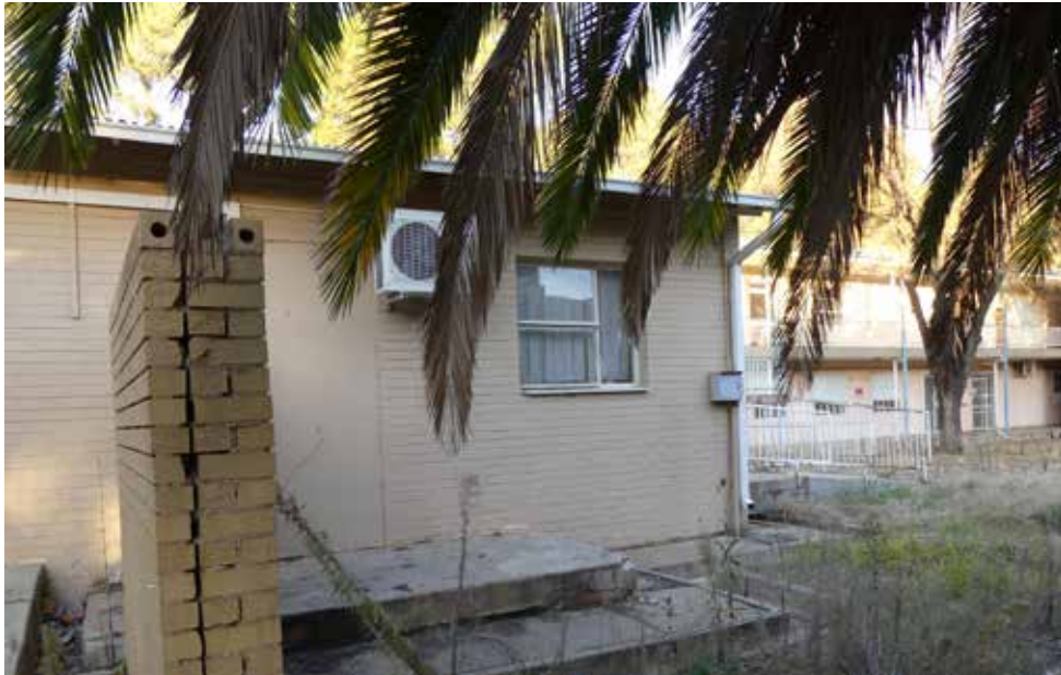
Western elevation - building 41.
