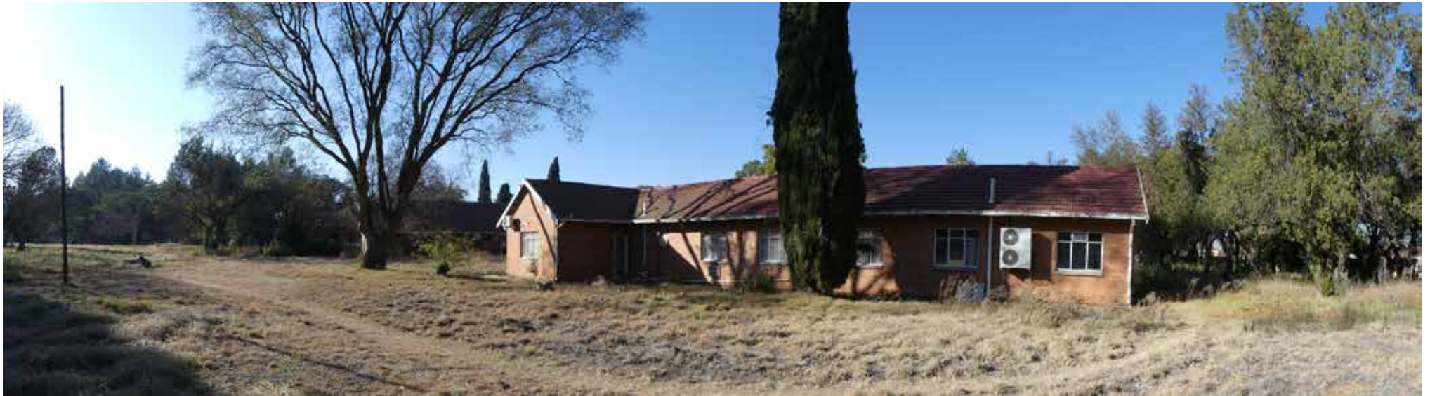
Panoramic view of Southern Elevation - building 16.
