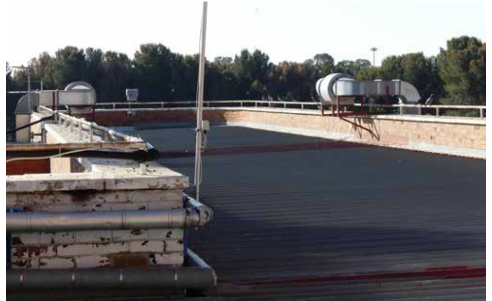
Contemporary corrugated roof sheeting placed over original flat roof - building 17.
