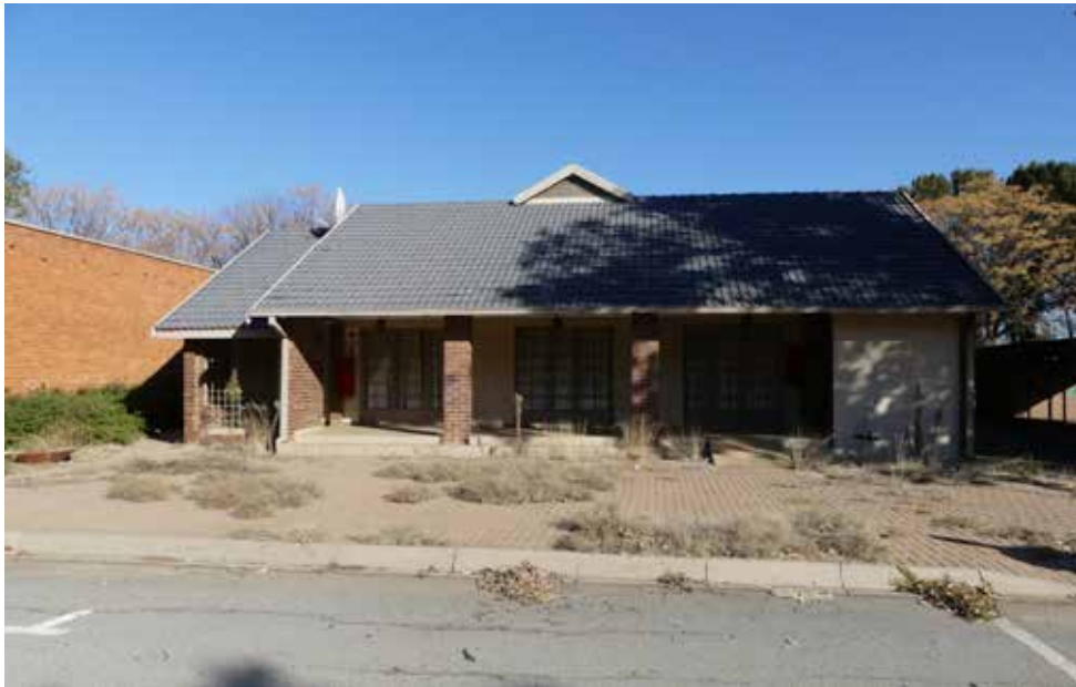
Northern elevation - building 27.
