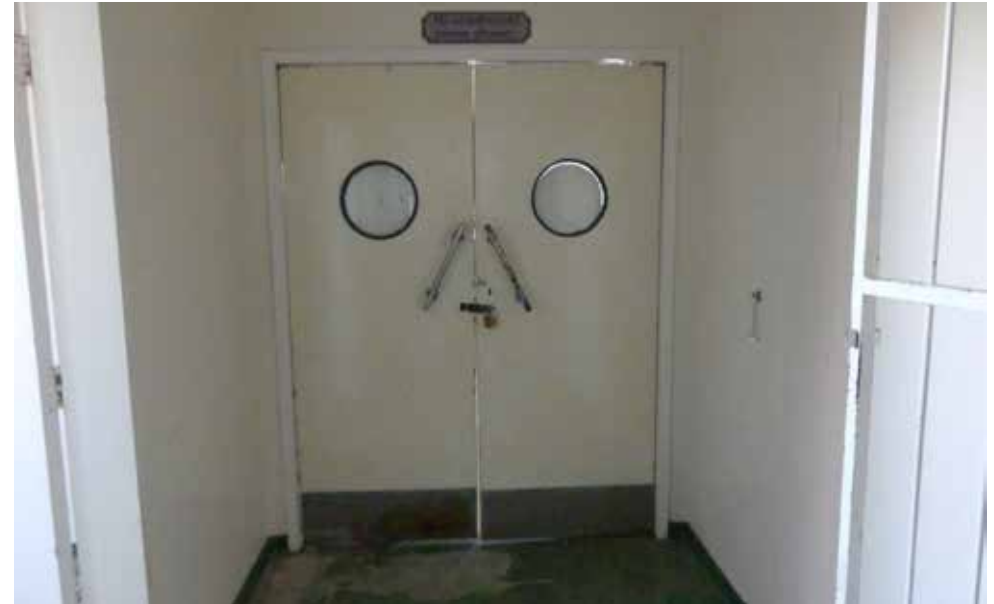
Original port hole doors on Second Floor - building 17.
