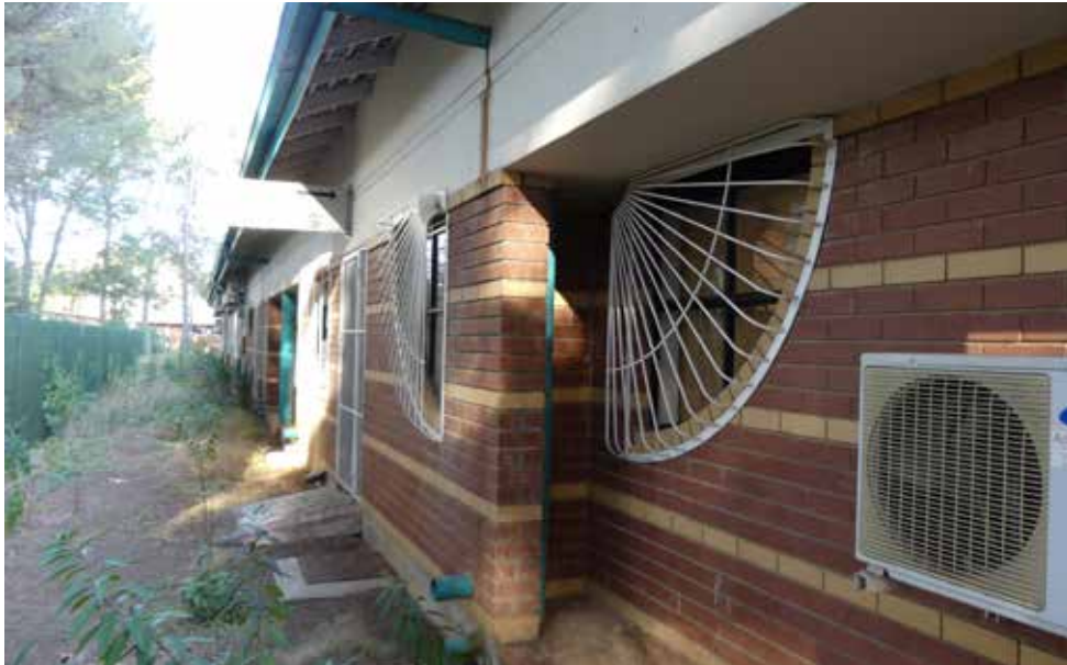
Detail of side of building 12.
