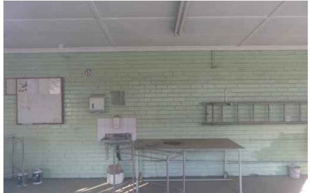
Interior of garage and paint shop - building 31.
