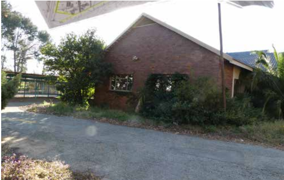
Southern elevation - building 24.
