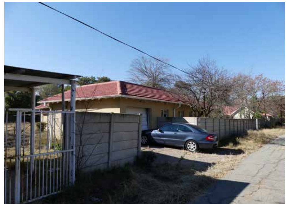
Entrance off of street of building 4 - Doctor's House Type 5.
