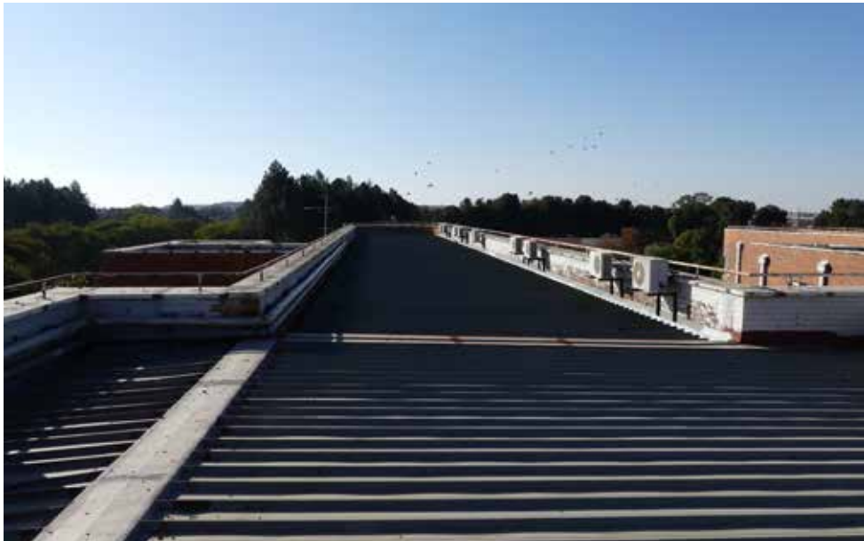
Contemporary corrugated roof sheeting placed over original flat roof - building 17.
