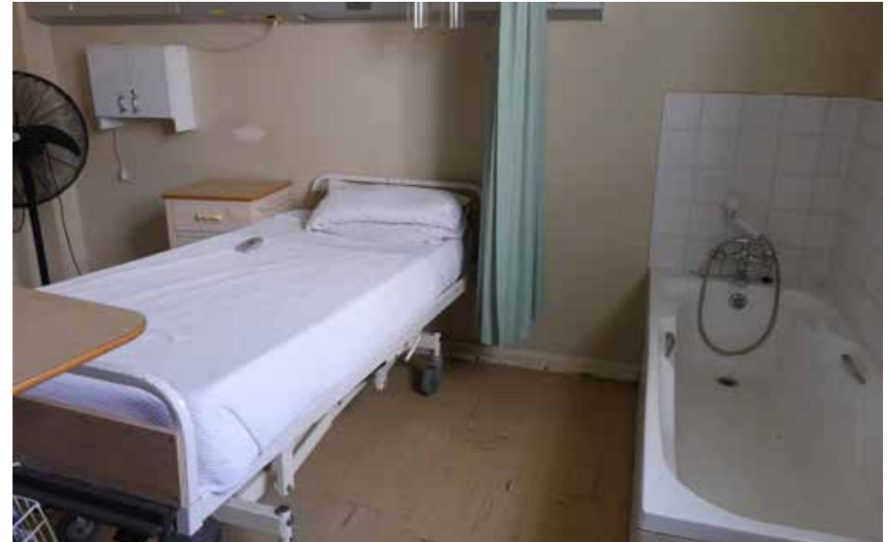
Beds in the ward on the Ground Floor - building 17.
