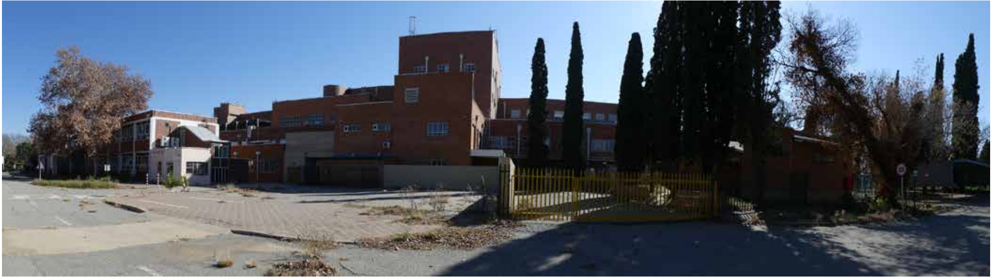
Panoramic view of partial Southern elevation of building 17 - Main hospital building service block.
