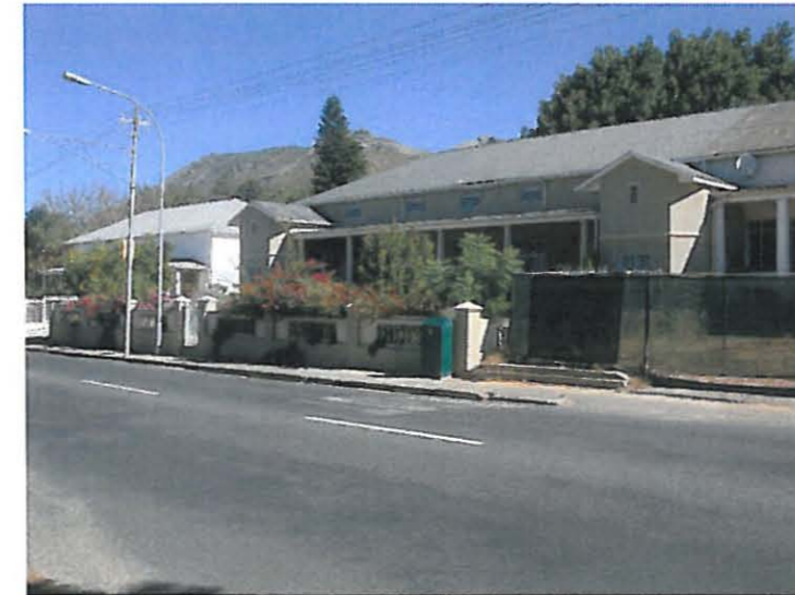
Site as viewed from Main Road in a westerly direction
