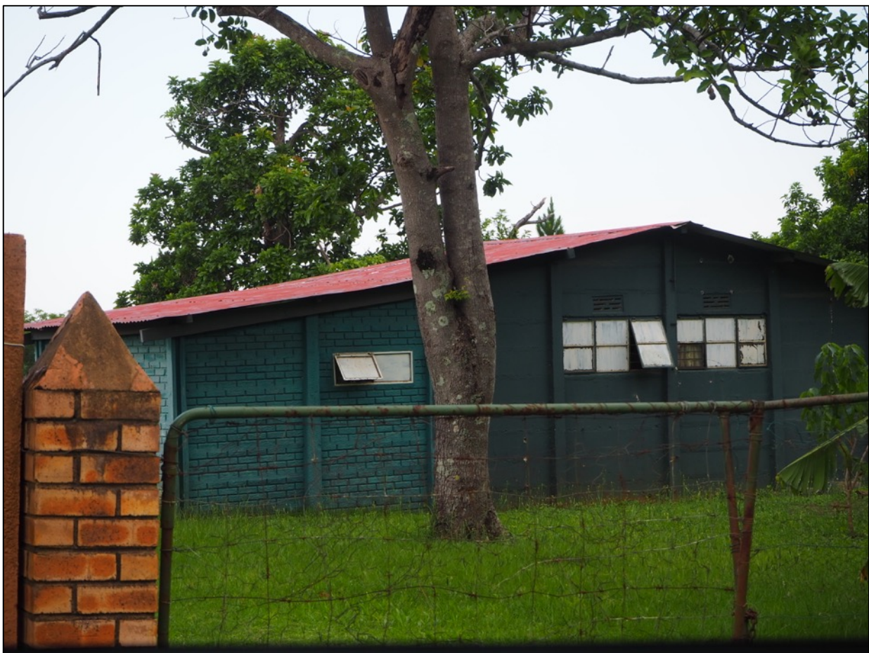
Figure 25. Occupational structure on site
