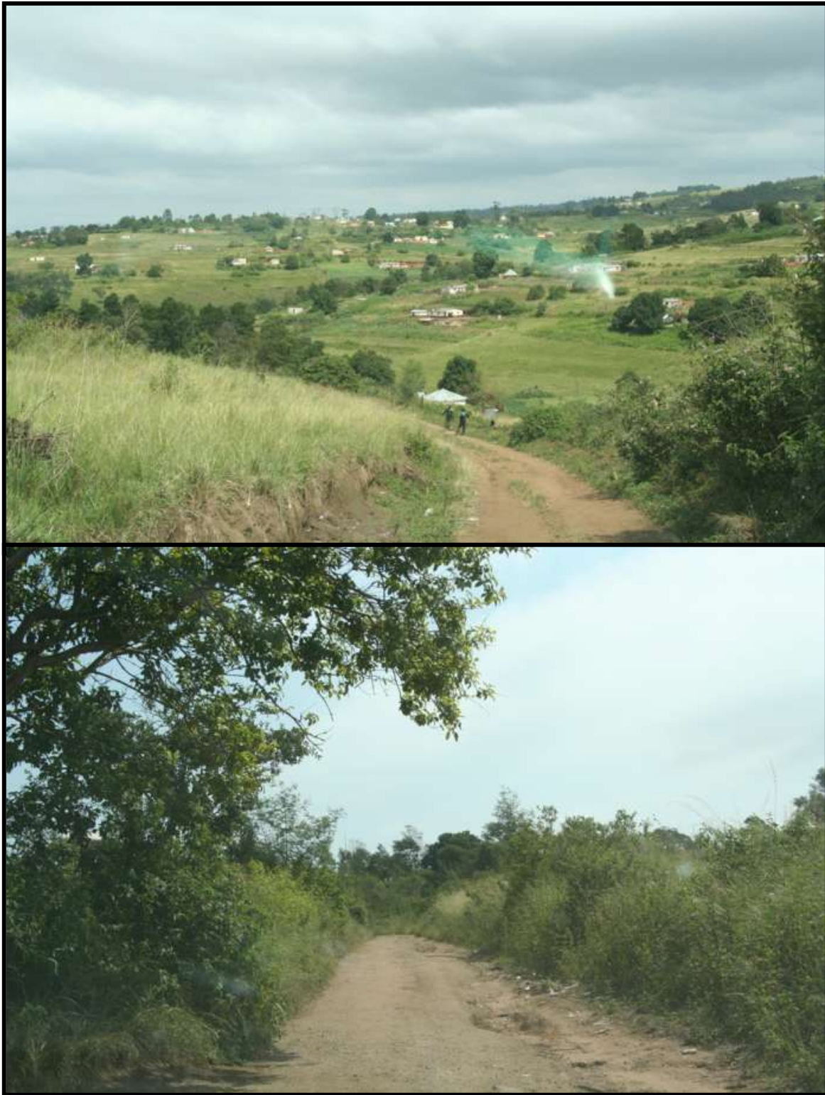
FIG. 7: GENERAL VIEWS OF THE ESIBHUKUDWENI ROAD
