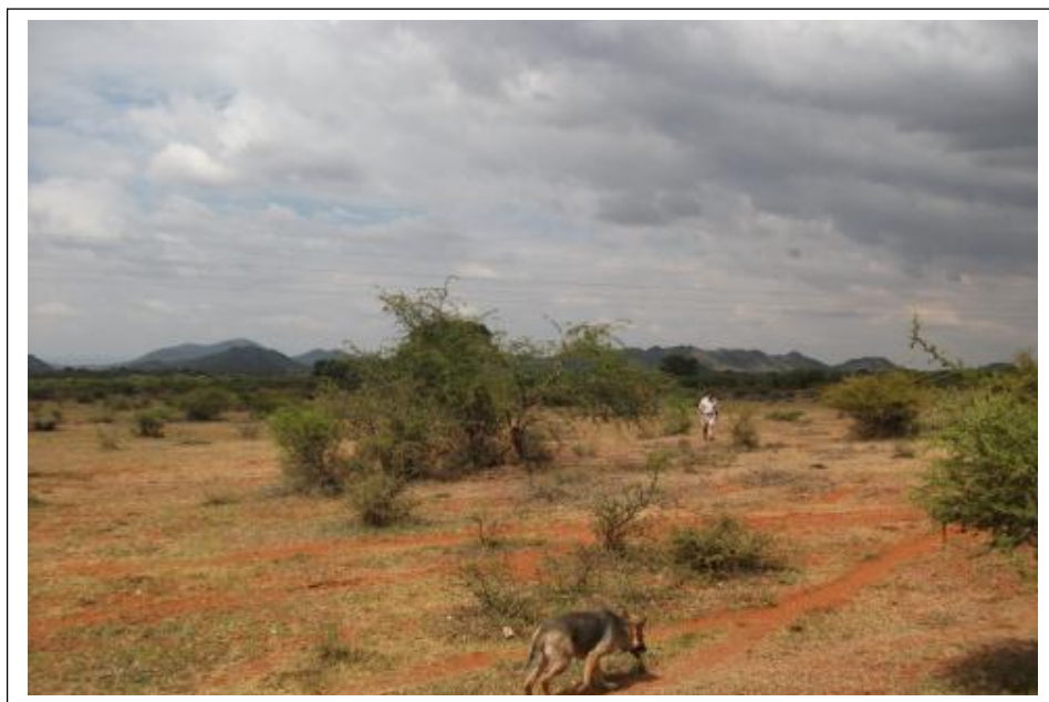
Figure 14- The proposed 132kV loop-in loop-out power line runs from the 132kV Middelpunt-Dithabaneng power line to the proposed new Boynton Substation. Both the power line and the substation are located in the midst of abandoned agricultural fields on the farm Mphatlele 457KS (above).
