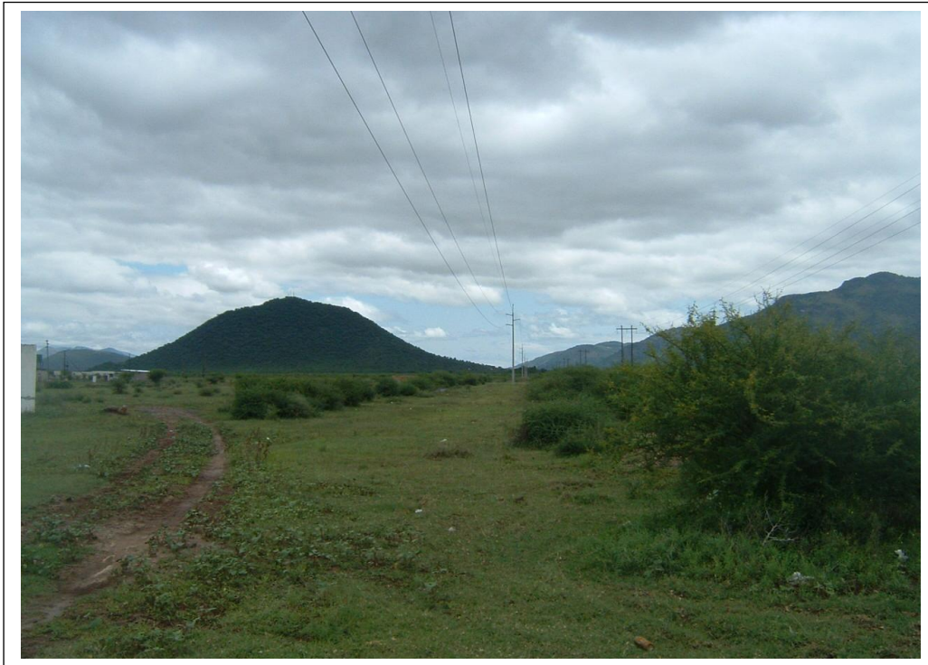
Figure 2- The Eskom Project Area to the west of the R555 near the Steelpoort River. The plate shows the view along Eskom's existing 132kV Jane Furse/Merensky power line. The proposed loop-in and loop-out power line will run from this power line to the proposed Grootboom Substation further to the east (above).
