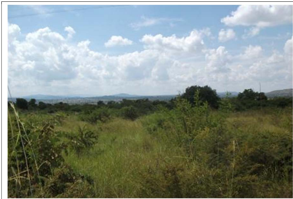
Figure 5- The Letaba/Tarentaalrand power line runs across relatively pristine bush north of the Letaba River before entering the Letaba Substation on the farm Letaba 567LT (above).
