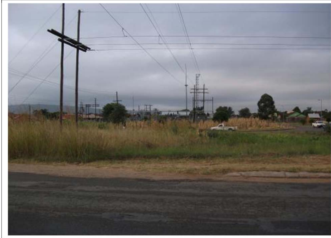
Figure 8- The 66kV power line running between the Letaba and the Risenga Substations will enter the Risenga Substation from the north after crossing a railway line and the road between Nokowankowa and Letsitele (above).
