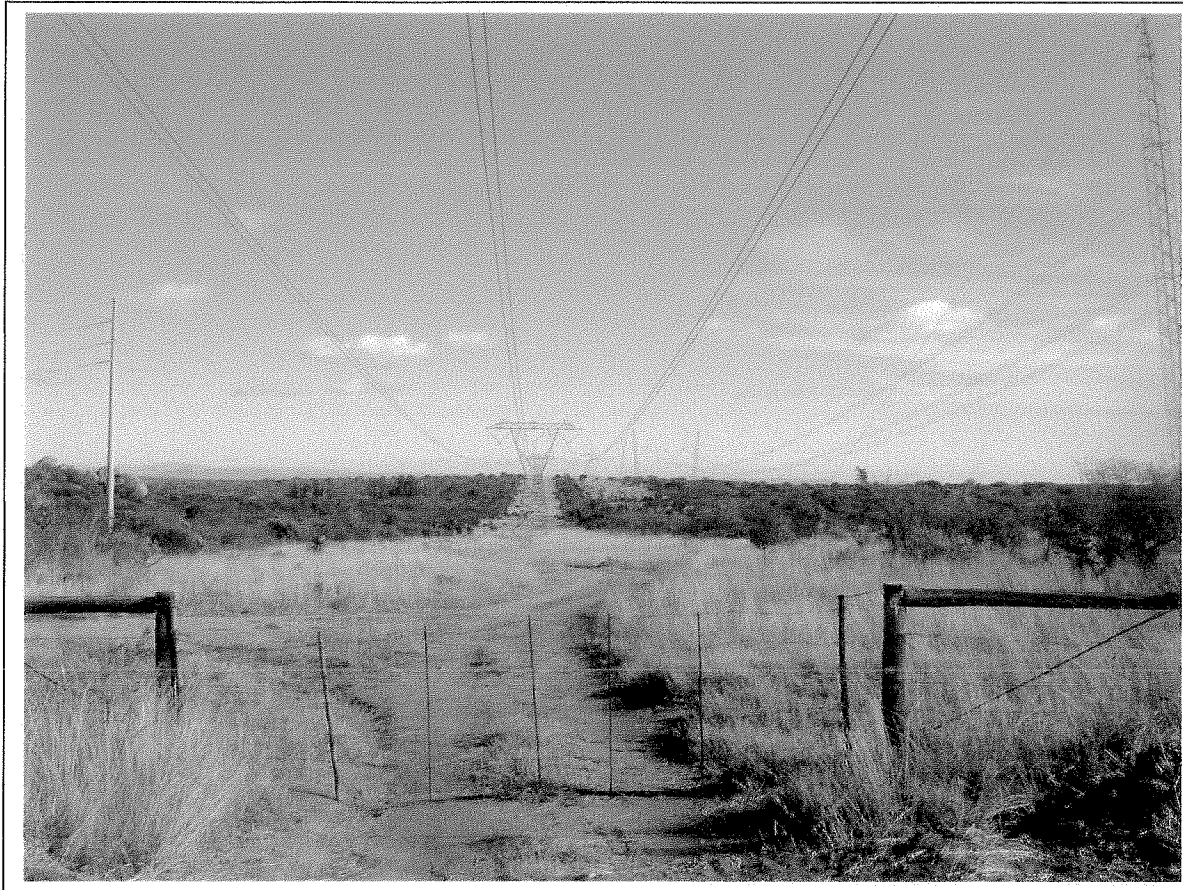
Figure 10- Option 04 for the proposed Mokopane Substation on the farm Noord Braband 774LR (above).
